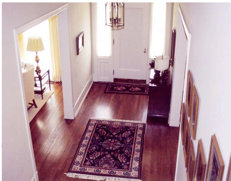
The original floors of quarter-sawed oak were exposed and refinished
