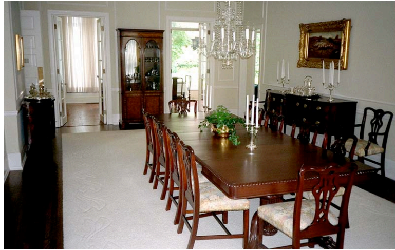
We repaired, replastered, and painted the walls.
