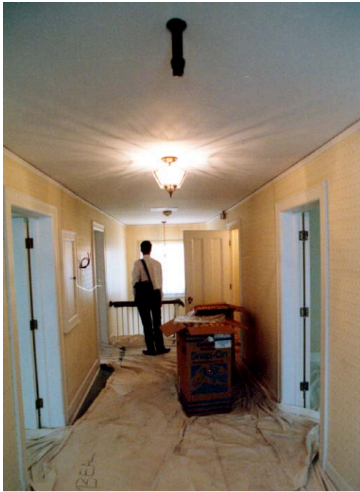
Installing the air handling and fire sprinkler systems
