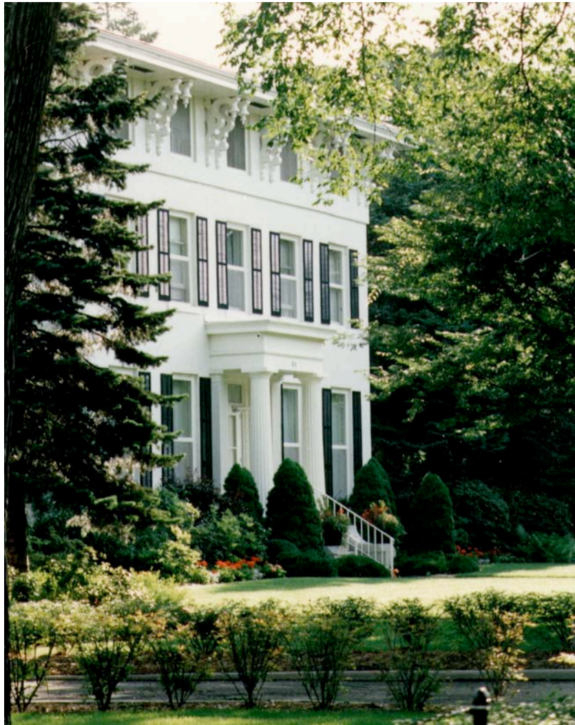
After the renovation
