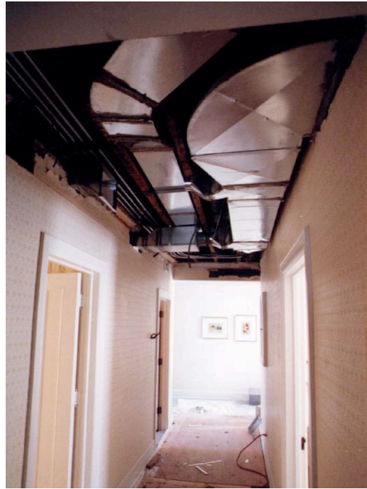
Installing the air handling and fire sprinkler systems
