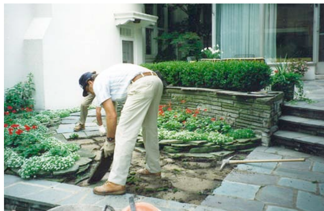
Repairing the patio
