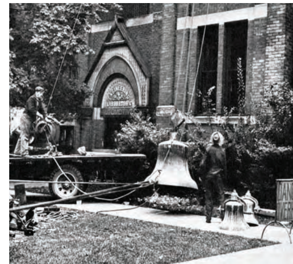
The bells were taken down from the Engineering Shop's Tower to be used as scrap metal for WWII.
