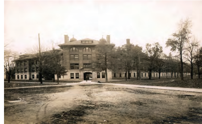
The New Engineering Building
