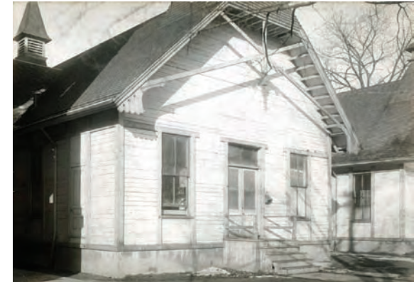
Surveying Building formerly the Pavilion Hospital
