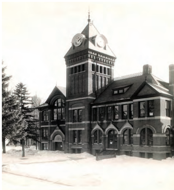
Engineering Shops with clock and chimes from the demolished University Library
