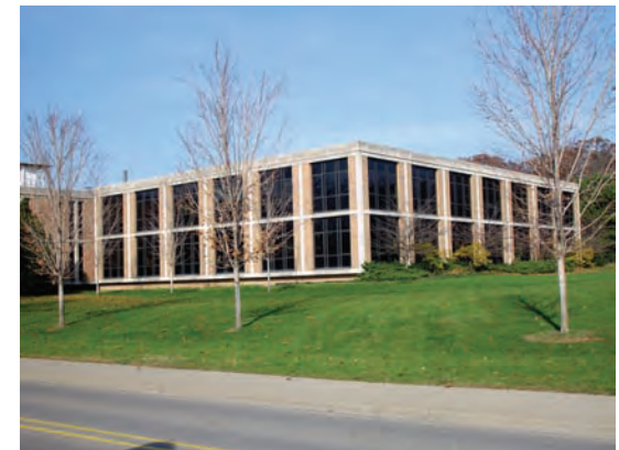
Space Physics Research Laboratory Addition
