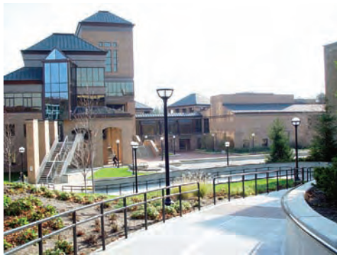
Lurie Engineering Center
