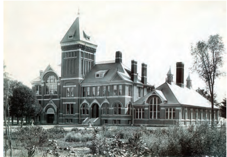
The Engineering Shops with the tower and forge (right)
