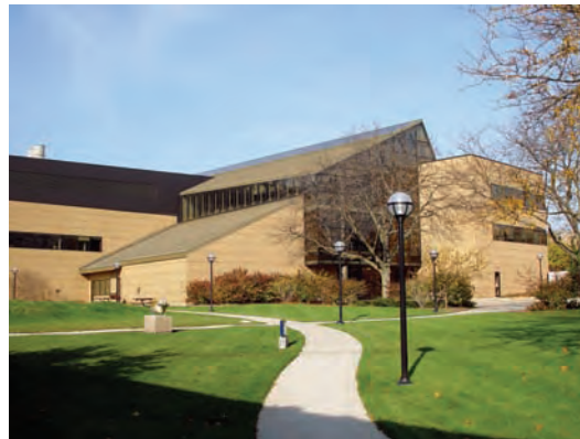
François-Xavier Bagnoud (FXB) Building
