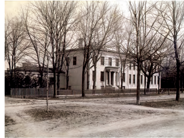
Dental Building on South University with the addition on the right of the Professors' House
