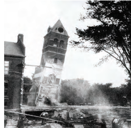
Demolition of the University Library Tower July, 1917
