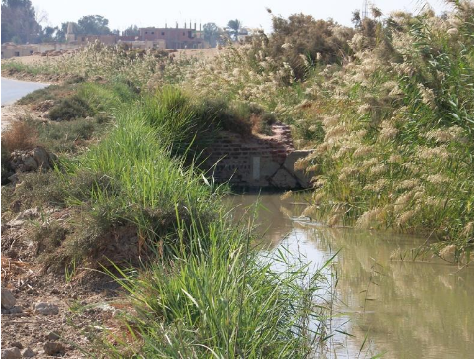
Figure 158: Modern water drop structure on the Bahr Wahbī near FD 22, facing west. Photo by author.
