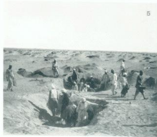
Excavation of canal B (p. 143) (see pl. xci, 5)
