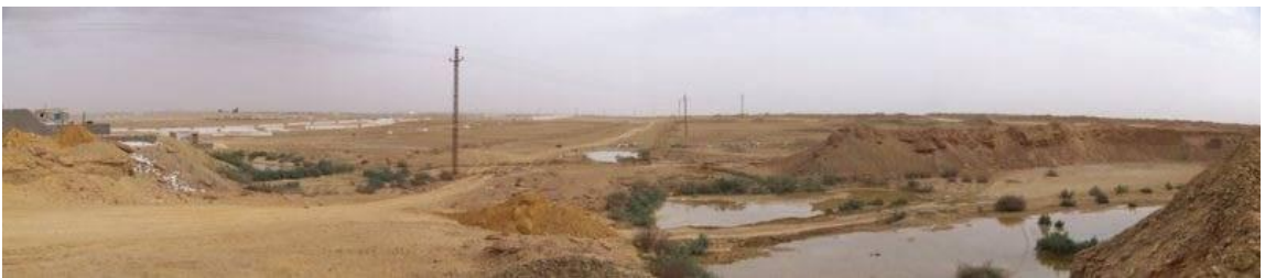
Figure 40: Landscape damage near the probable course of Canal C. Photo taken from the southern end of Qarya Thalatha, facing northeast. Quarrying damage is visible at right. The white features to the left are stone blocks loosely laid as foundation courses for settlement expansion. The area will become private property unless the government removes the blocks.
