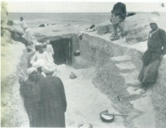
Canal F, with tunnel, overlooking L. basin (p. 143)
