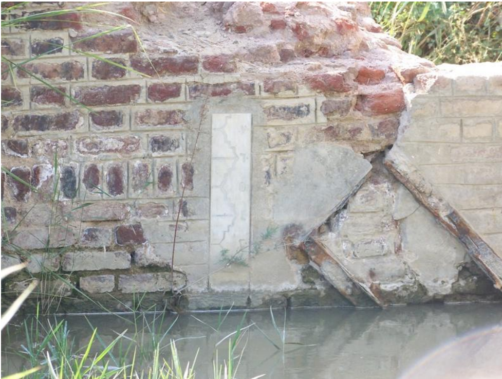
Figure 159: Detail of water level measurement device on the east face of the drop structure shown above. Photo by author.
