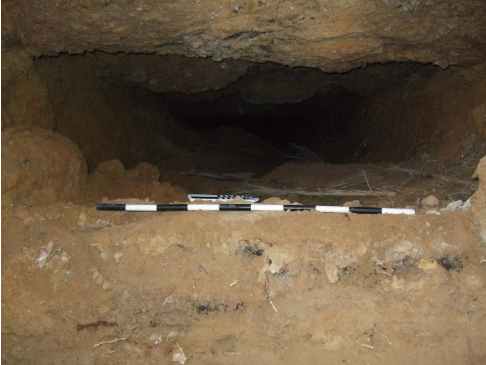
Figure 56: FD 025. Interior of the tunnel in Canal F after removal of debris, facing west. Photo by author.
