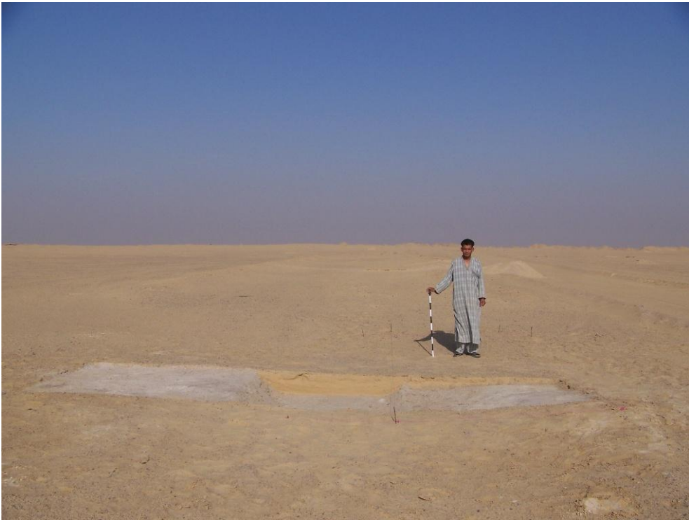
Figure 76: Trench FD 009 post-excitation of Canal G alignment, facing west. The lower elevation of the north bank is visible at right. Photo by author.
