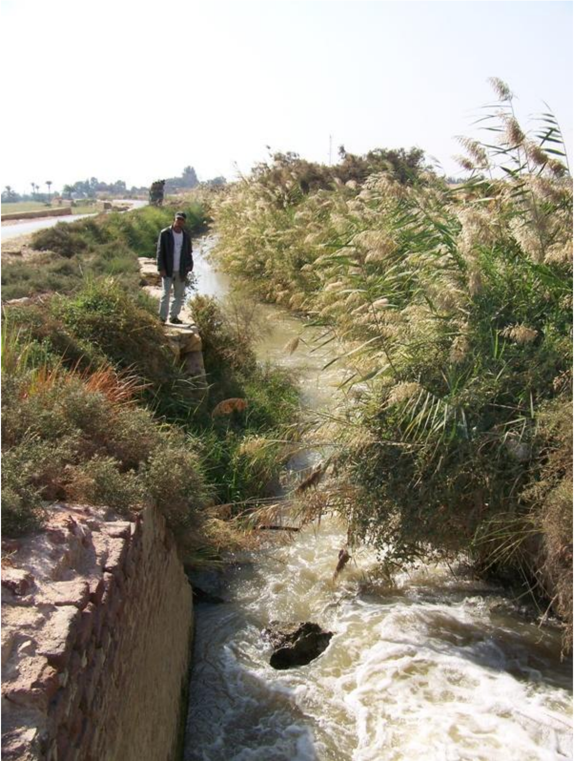
Figure 160: High energy flow behind the water-drop shown above. A number of brick retaining walls have been built to limit erosion. The rocks in the bottom of the channel are known as rip-rap and are intended to dissipate energy. Photo by author.
