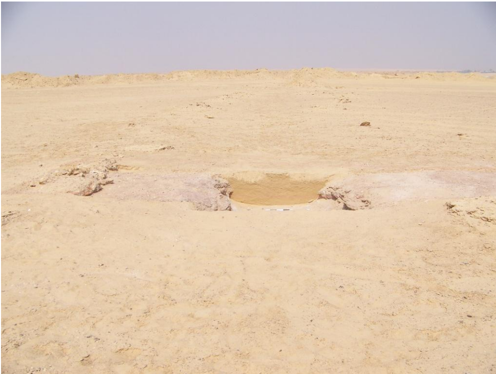
Figure 62: Trench FD 007 post-excitation of Canal G alignment, facing northwest. Photo by author.
