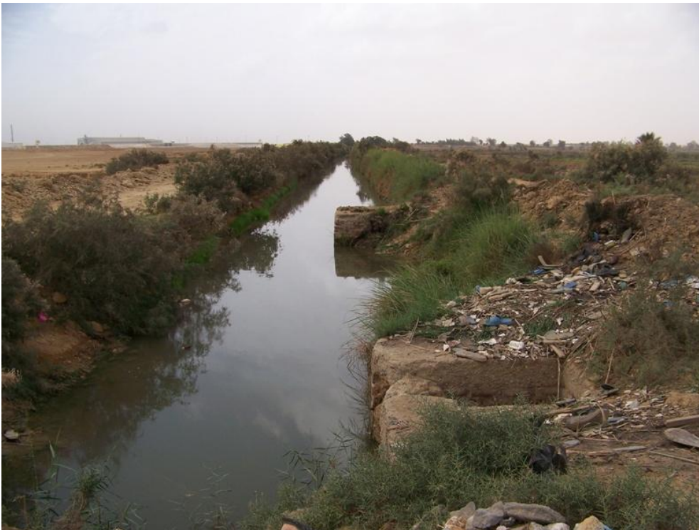
Figure 47: The southern terminus of the modern Tira’at al-Jamhurriyah at the southern end of the L-Basin, facing west. The canal follows the line of the “Embankment” indicated on Caton-Thompson and Gardner’s map of the irrigation system and may reuse it for one or both berms. Photo by author.
