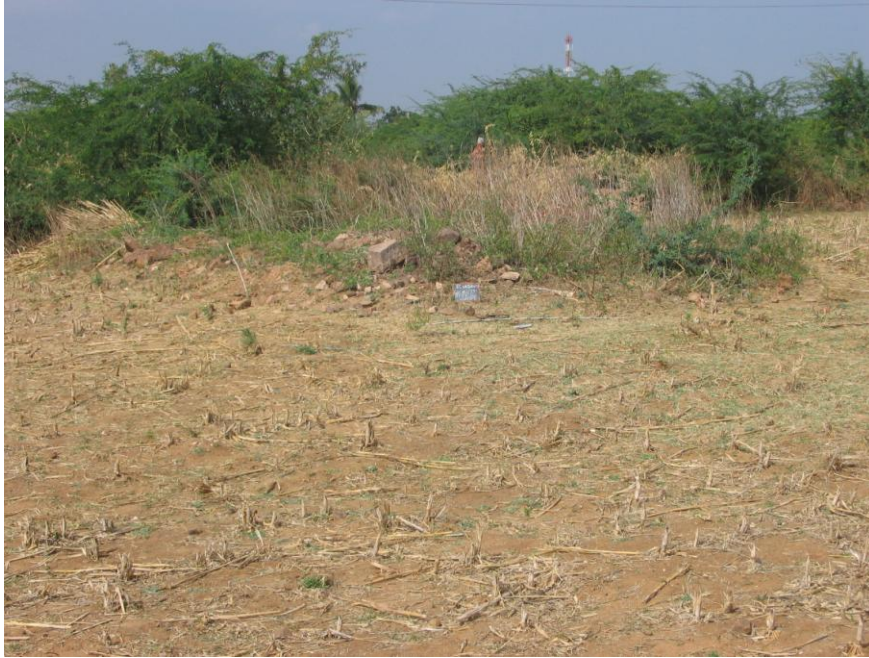
Figure 4.22: Loc. 0730 Collapsed brick structure.
