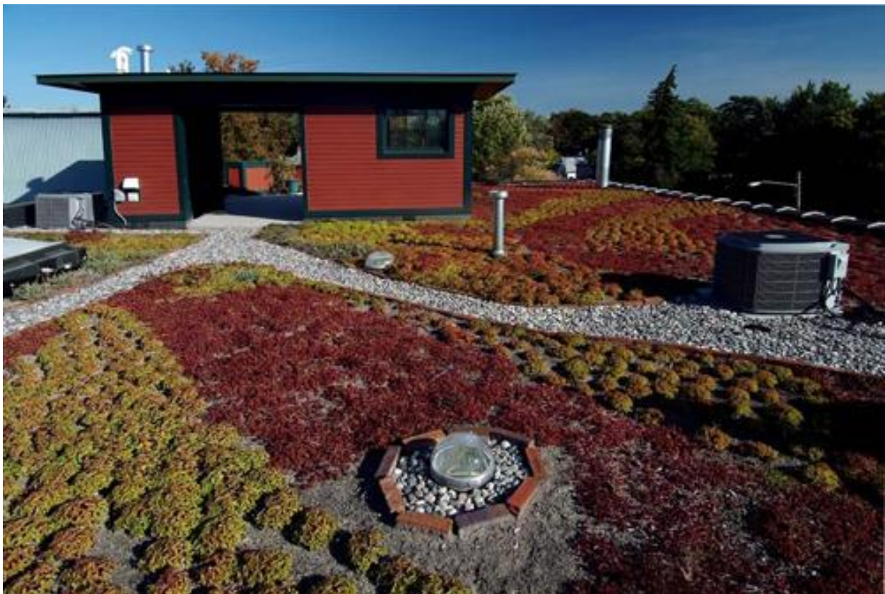
Figure 7.2. Green Roof atop the East Hills Center (of the Universe) building in Grand Rapids. Designed by Guy Bazzani. Source: Cool Cities. "The Uptown Revitalization Project." Accessed from: http://www.coolcities.com/project61.html .
