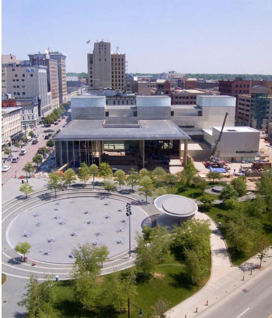
Figure 8.3. Grand Rapids Art Museum, aerial view. Source: Grand Rapids Art Museum: LEED Gold Certified / WHY Architecture. why architecture? Accessed from http://ad009cdnb.archdaily.net/wp-content/uploads/2008/05/gram-aerial.jpg .
