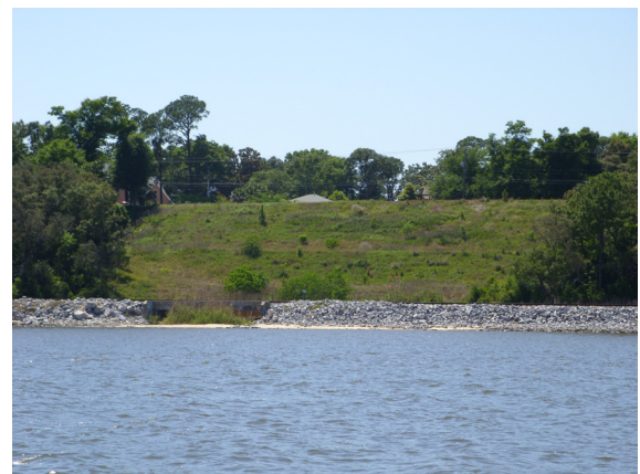
Figure 7- Mallory Heights Current Condition, 1
