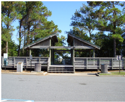
Figure 11- Bay Bluffs North Current Condition, 1
