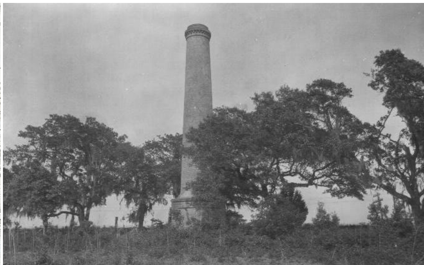
Figure 4- Historical Image, Old Chimney, 1940s
