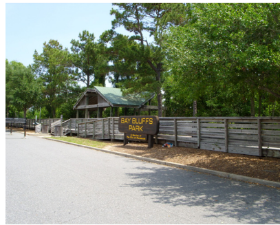
Figure 12- Bay Bluffs North Current Condition, 2
