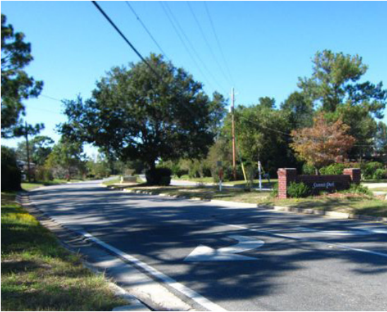
Figure 14-Summit Boulevard- Current Condition
