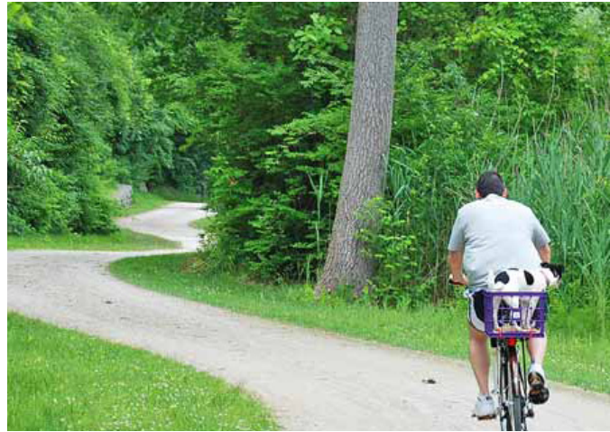
Figure 194- Crushed Limestone Pathway
