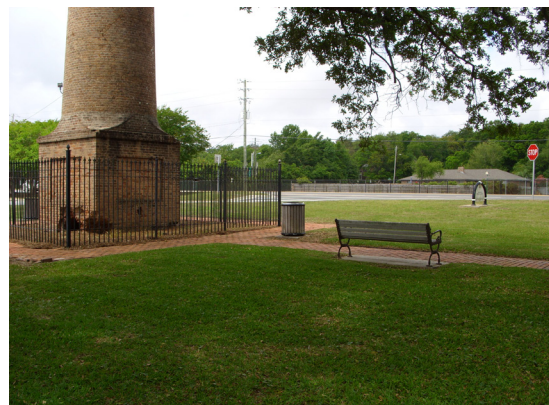
Figure 15- Chimney Park Current Condition, 1
