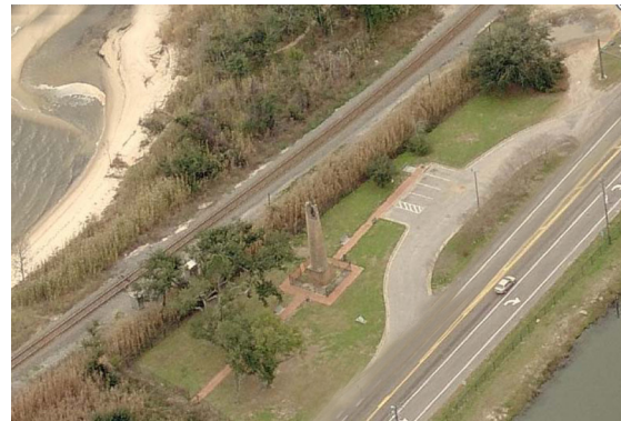
Figure 128- Chimney Park Current Site Condition
