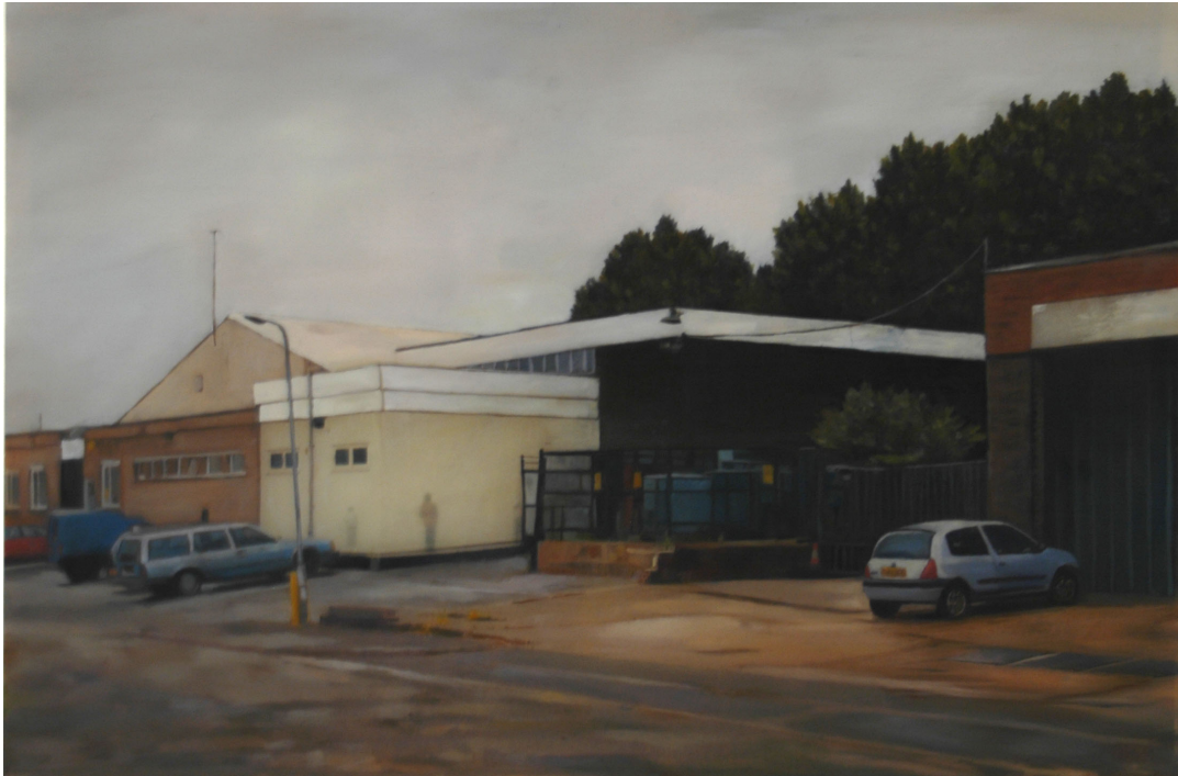
Figure 26 - Storage Unit. Mentor, Ohio.
