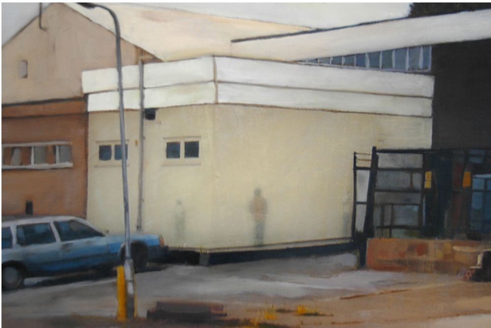
Figure 27 - Storage Unit. Mentor, Ohio – detail.
