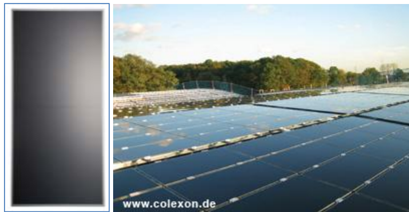
Figure 62. CdTe PV cell modules (First Solar, 2012).
