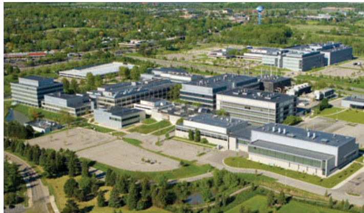
Figure 114. North Campus Research Complex (NCRC).
