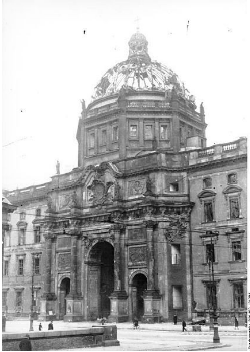
Fig. 32. Damage to west façade of Stadtschloss and cupola around February to March, 1945. Bundesarchiv, Photo 183-J31381. Photographer unknown.
