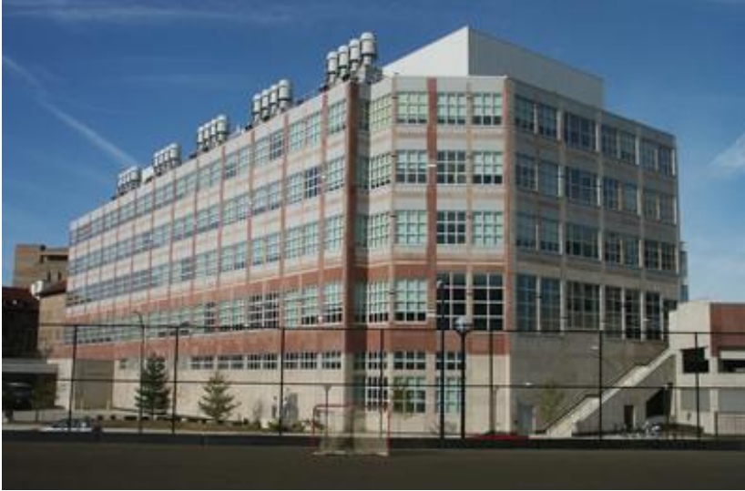
Figure 4.2 Exterior photo of the LSI (University of Michigan, 2010)
