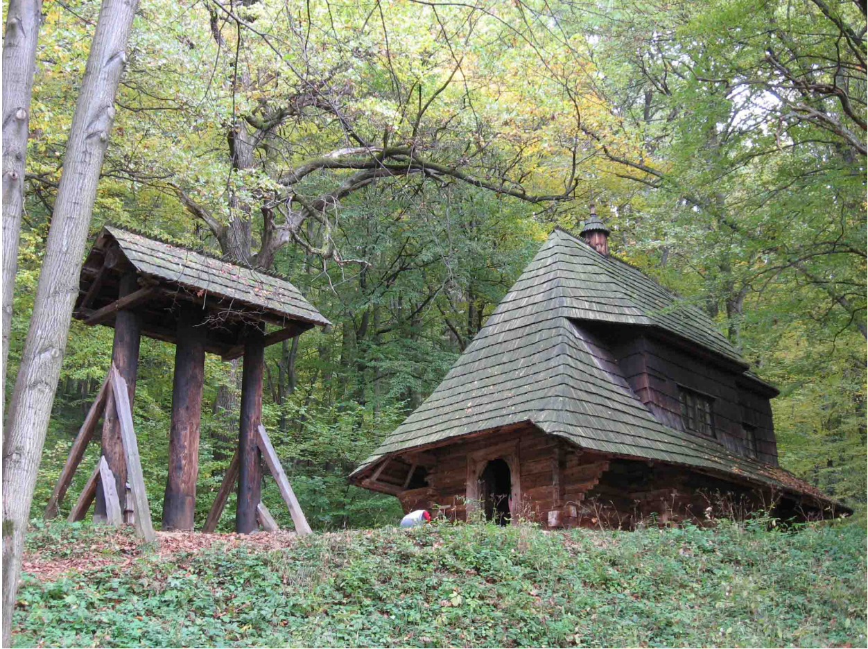
Image 4.5: Exterior of the Church of the Coronation of the Blessed Virgin (1750), originally at Rosolin (Ustrzyki Dolne county), Museum of Folk Architecture, Przemyśl. A small village church, architecturally typical of the Boyk mountaineer inhabited Subcarpathian region of the Polish Lithuanian Commonwealth.
