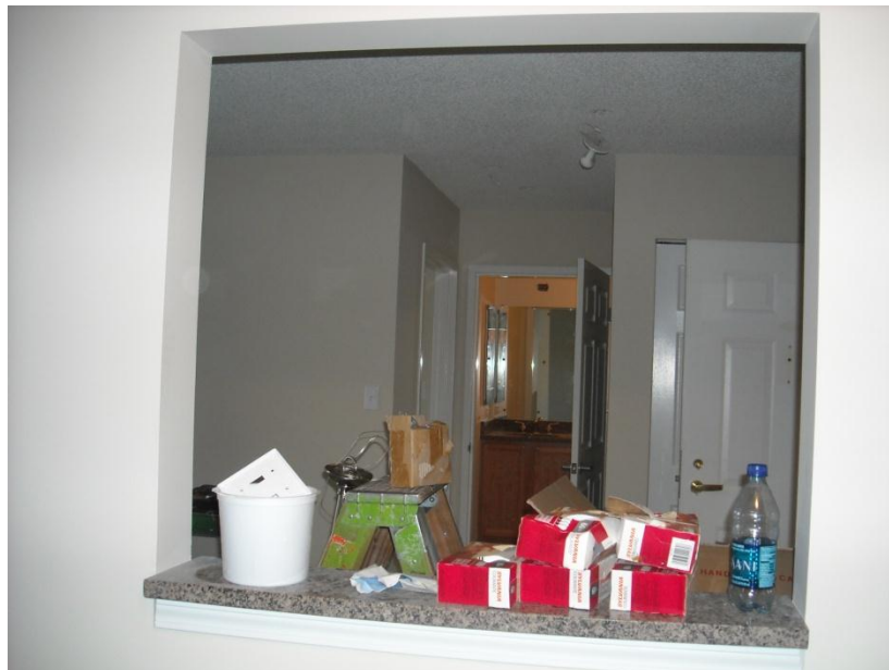
Photo 5.4– “Wall Cutouts” in Older Retirement Community to Remodel
