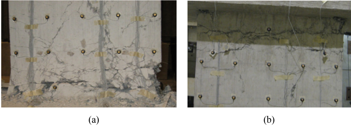
Figure 4.8 Damage on the back side of Specimen CB-1 at 5.2% drift at (a) the bottom end and (b) the top end of the beam
