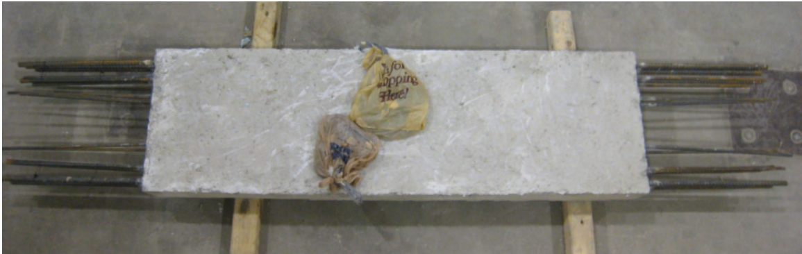
Figure 3.7 Precast coupling beam after demolding
