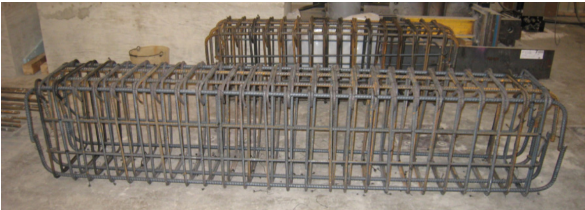
Figure 3.8 Reinforcement cages for top and base blocks
