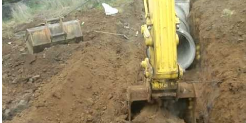
Fig. 4.1: Limited visibility facing excavator operators and uncertainty regarding location of buried utilities
