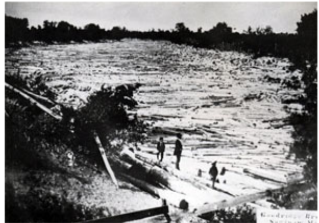
Figure 1.4: Log float on the Tittabawassee River in Saginaw County, MI (HSSC 2013).
