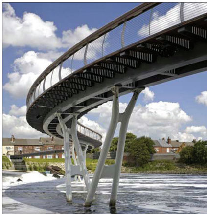
Curved pedestrian bridge in Castleford, West Yorkshire England . Designed by Architects McDowell+Benedetti , this is an excellent example of the type of innovative design that could define the 200 Block's pedestrian bridge over the Boardman River. (Photo by Tim Soar.)
