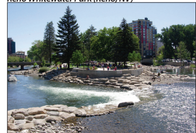
Reno Whitewater Park (Reno, NV)
