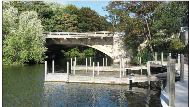
Crest of Union Street Dam (bottom): Fish ladder and utility building along with existing infrastructure functionality should be considered in any retrofit to the dam.
