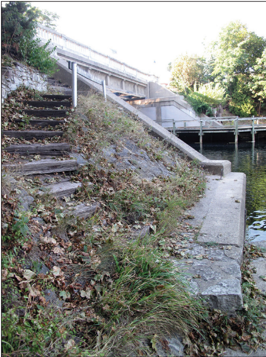
Steep Slopes Along Union Street (left): This access point is inaccessible and dangerous. The pedestrian tunnel would provide an accessible alternative to this entrance while connecting to the larger path system along the river.
