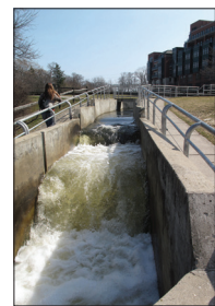
Figure 46: Existing Dam and Proposed Retrofit. The existing dam, fish ladder and secondary spillway will be altered for the proposed whitewater park. Proper functioning of the park will require additional fill and an expanded riparian edge.
