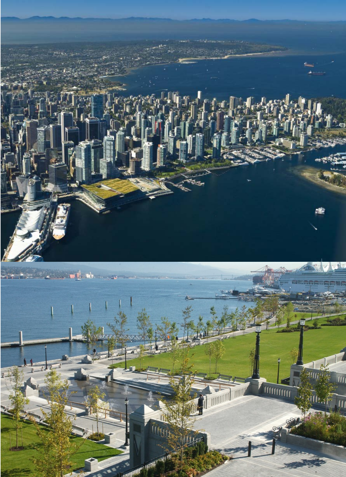
Figure 10.42: Coal Harbour and surrounding context, looking South, and central fountain at looking north east, in the early morning. (photographs and landscape design by PWL Partnership).
