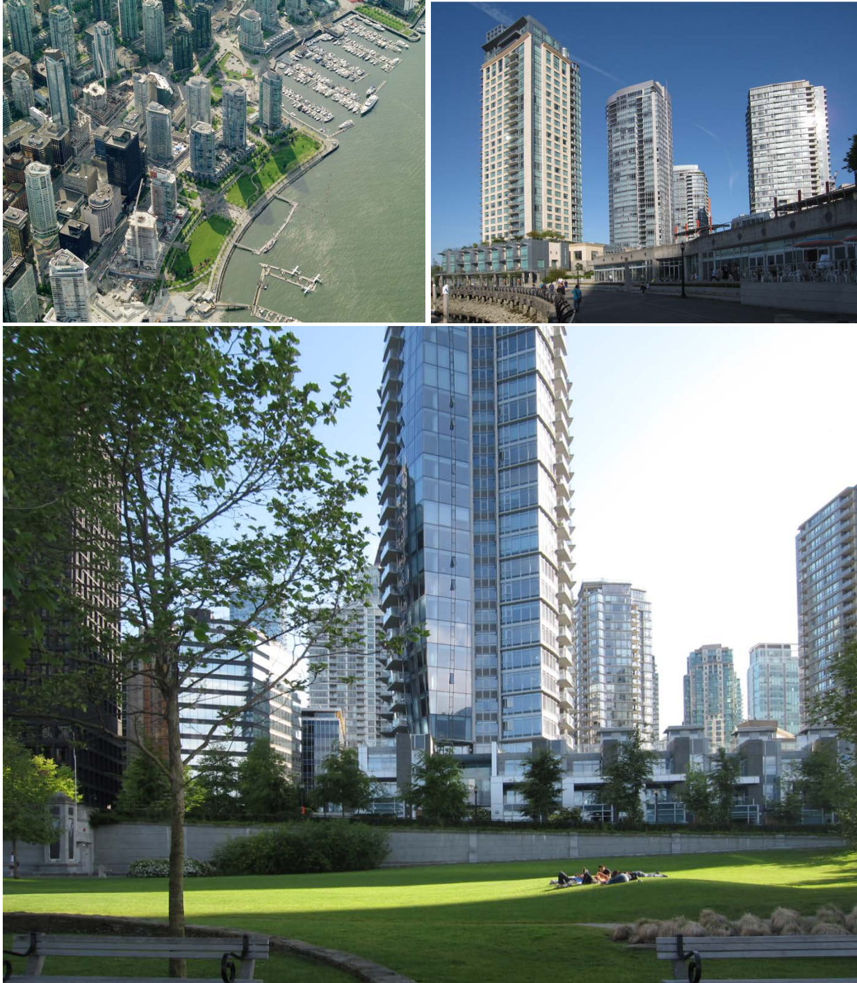
Figure 10.43: The eastern end the Marathon property at Coal Harbour (bing-3-d, Robert Walsh).
