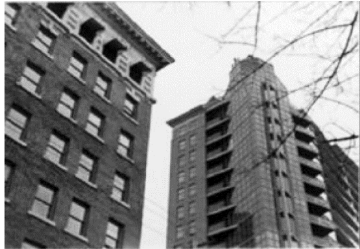
A contemporary building incorporating elements from the adjacent heritage building.
