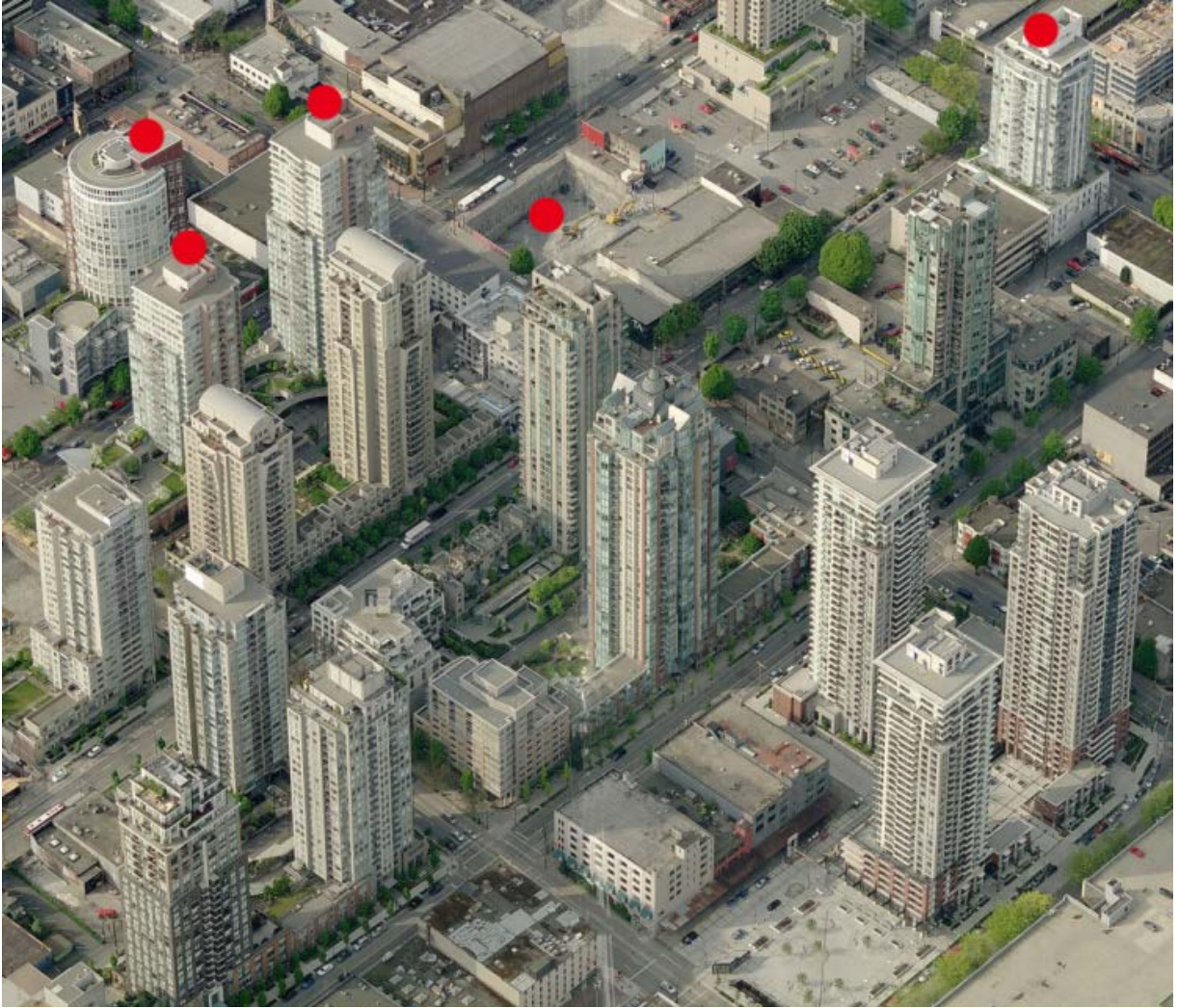
Figure 10.52: Image 3 from figure 10.49: Downtown South neighborhood, adjacent to Yaletown. Tower under construction and other towers with red dots are CD-1 projects; all other towers shown in this image were constructed without rezoning, using default guidelines (bing 3-d).
