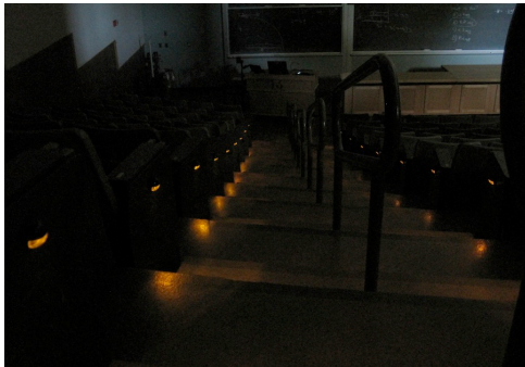
Fig 2a - Stairway lighting.
