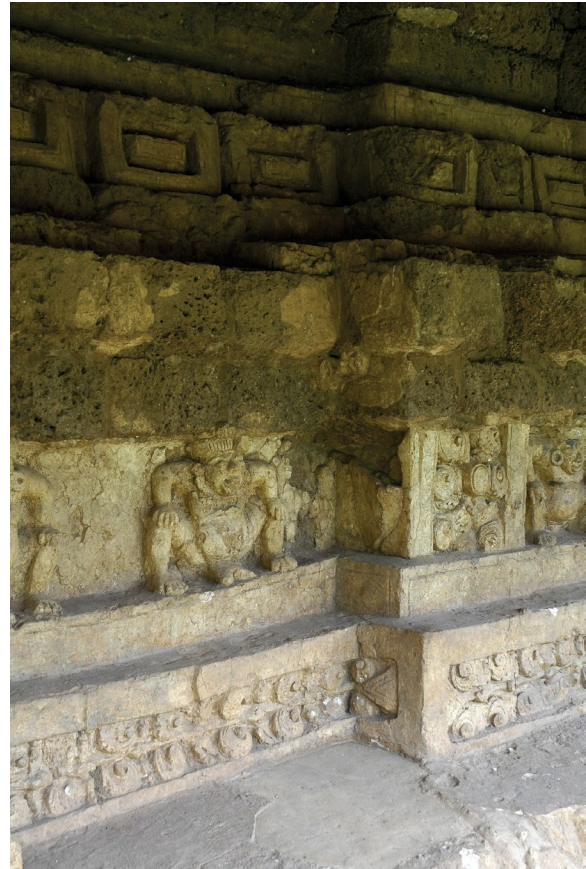
Figure 3.6. Stucco sculpture of “dwarves” and decorative motifs at the base of the Khao Klang Nai monument, Sri Thep. Note the laterite blocks visible behind the stucco façade.
