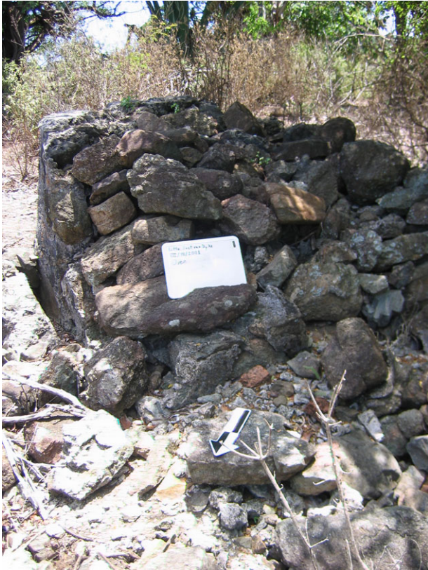
FIGURE 7. Ruins of an oven behind the Lettsoms' house. (Photo by the author)
