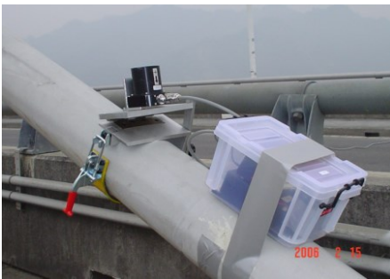
Figure 6 Sensor on Gi-Lu bridge
