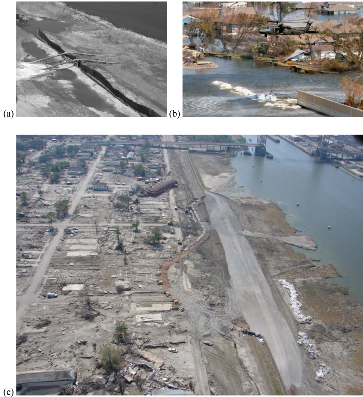
Figure 1-1, Levee failures in New Orleans resulting from Hurricane Katrina (a) Levee erosion along St. Bernard Parish frontage (Seed et al 2008a), (b) Emergency repairs at the 17 th Street Canal levee breach (Seed et al 2008c), and (c) Lower 9 th Ward Inner Harbor Navigation Canal Levee Failure ( with emergency repair levee in place ) (Seed et al 2008b)
