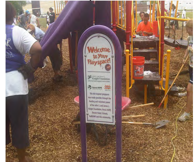
Figure 3.8 KaBoom playscape construction at the Paul Robeson Academy
