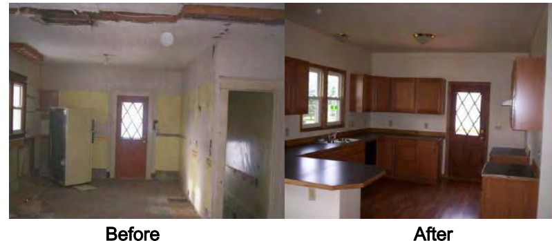
Figure 5.4 Kitchen Rehabilitated by Genesee County Land Bank
