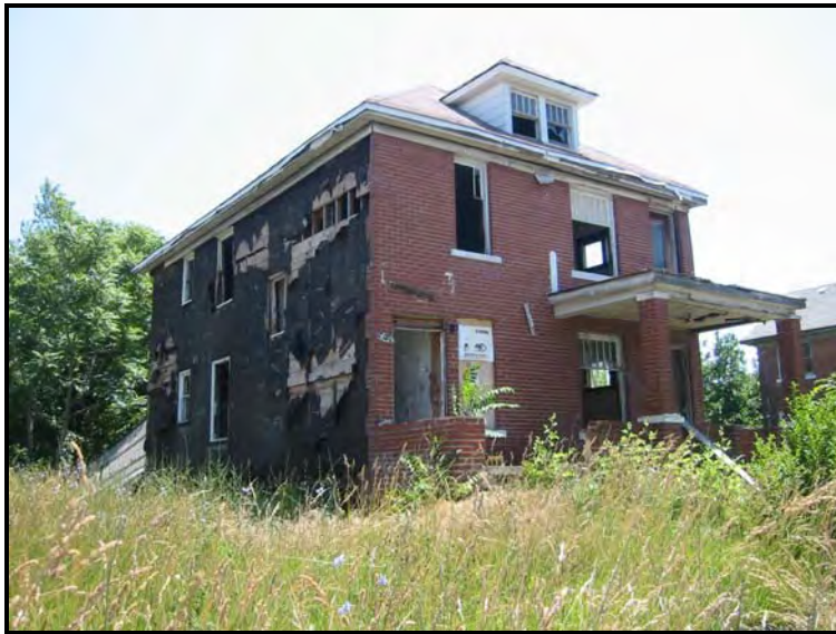
Figure 4.2 Possible Structure Targeted for Demolition – Detroit
