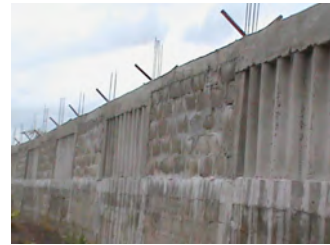
Photo 16: Existing Brick Fence. (Photo by Dennis Aggrey)
