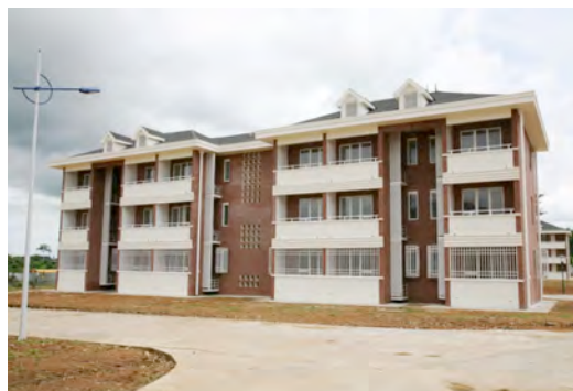
Photo 6: Dormitory buildings for faculty members
