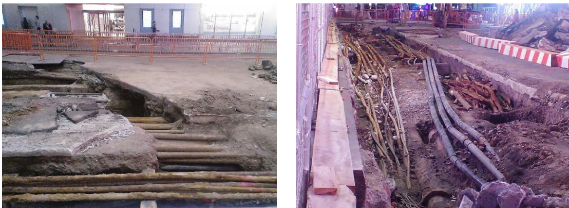
Figure 2.1 Examples of urban underground congestion
