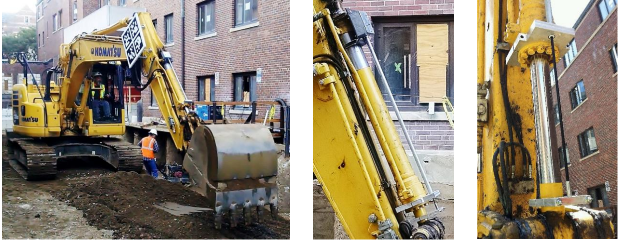
Figure 2.26 Cable potentiometer prototype installed on Komatsu excavator
