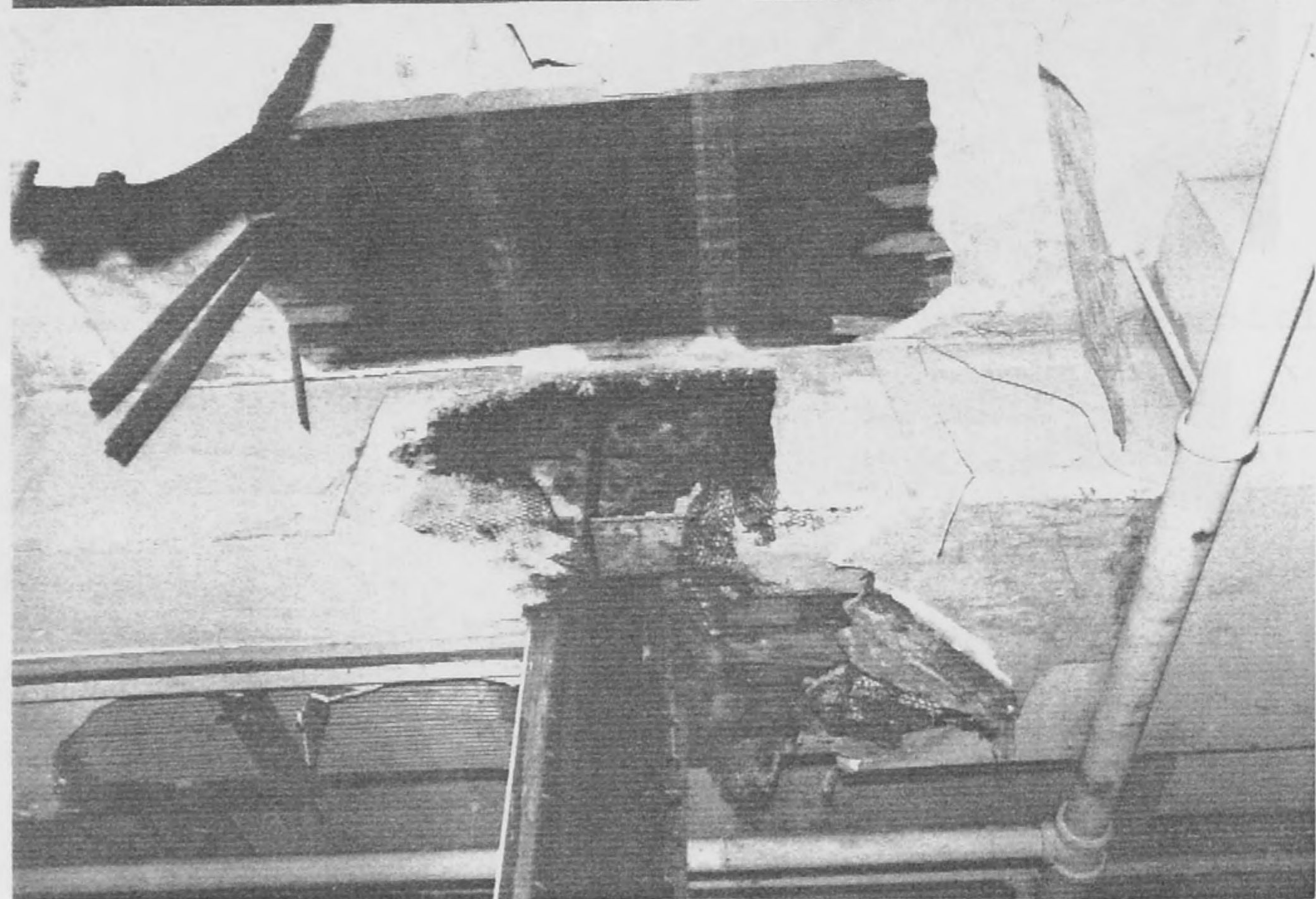
Fig. 6.13 Details of Steel Frame in Building G
