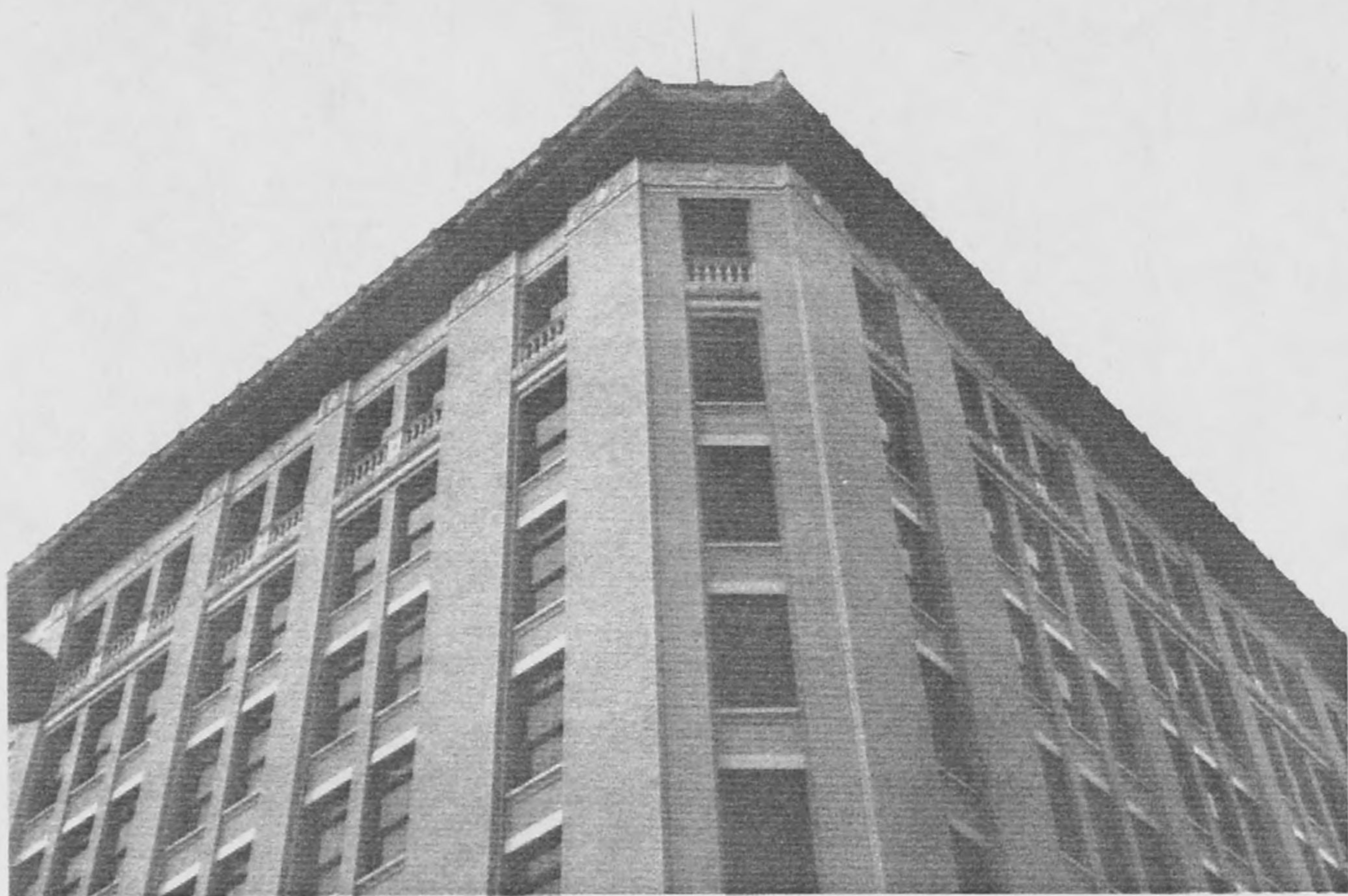
Fig. 6.20 Parapet of Building J
