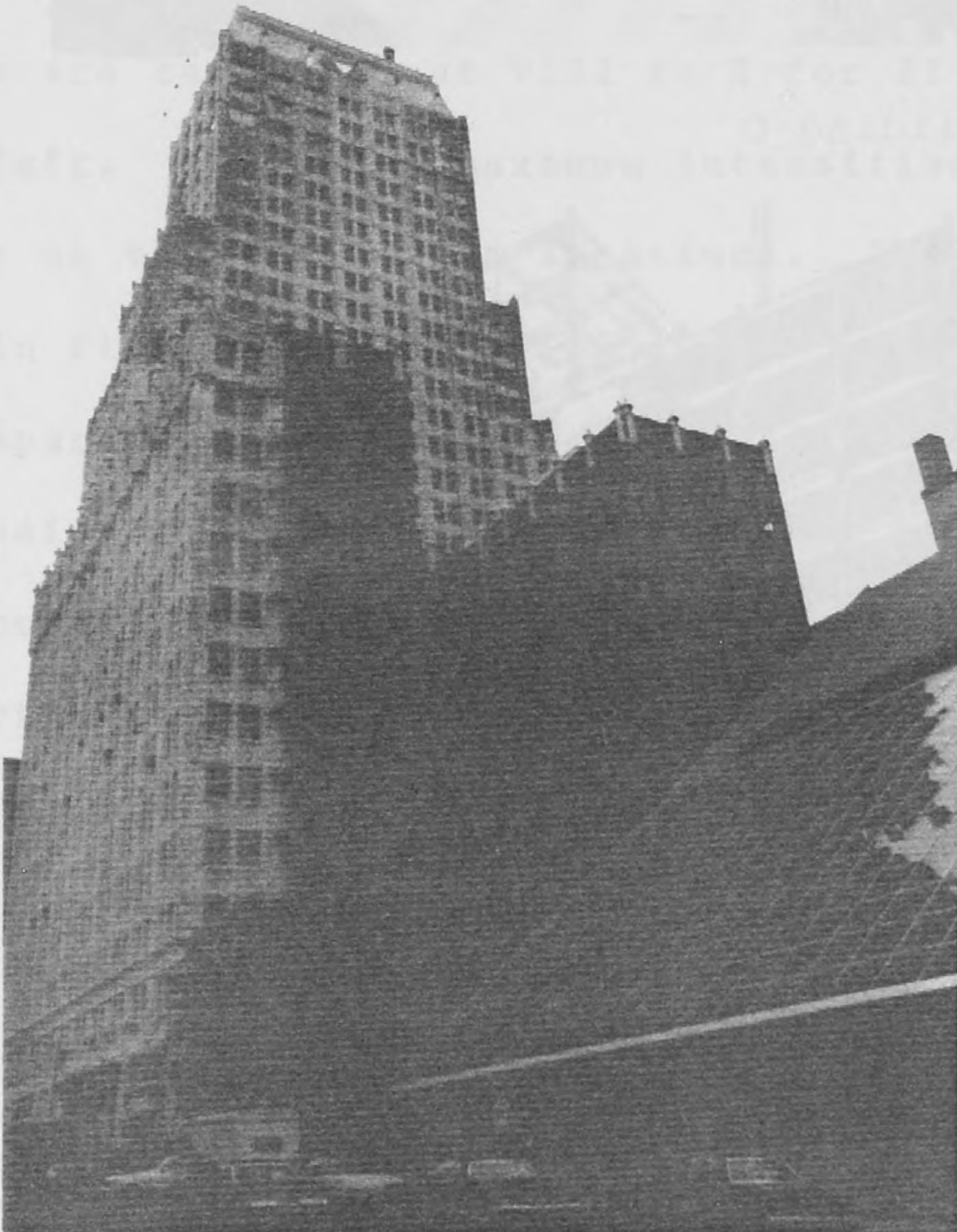
Fig. 6.25 Back Side of Building N
