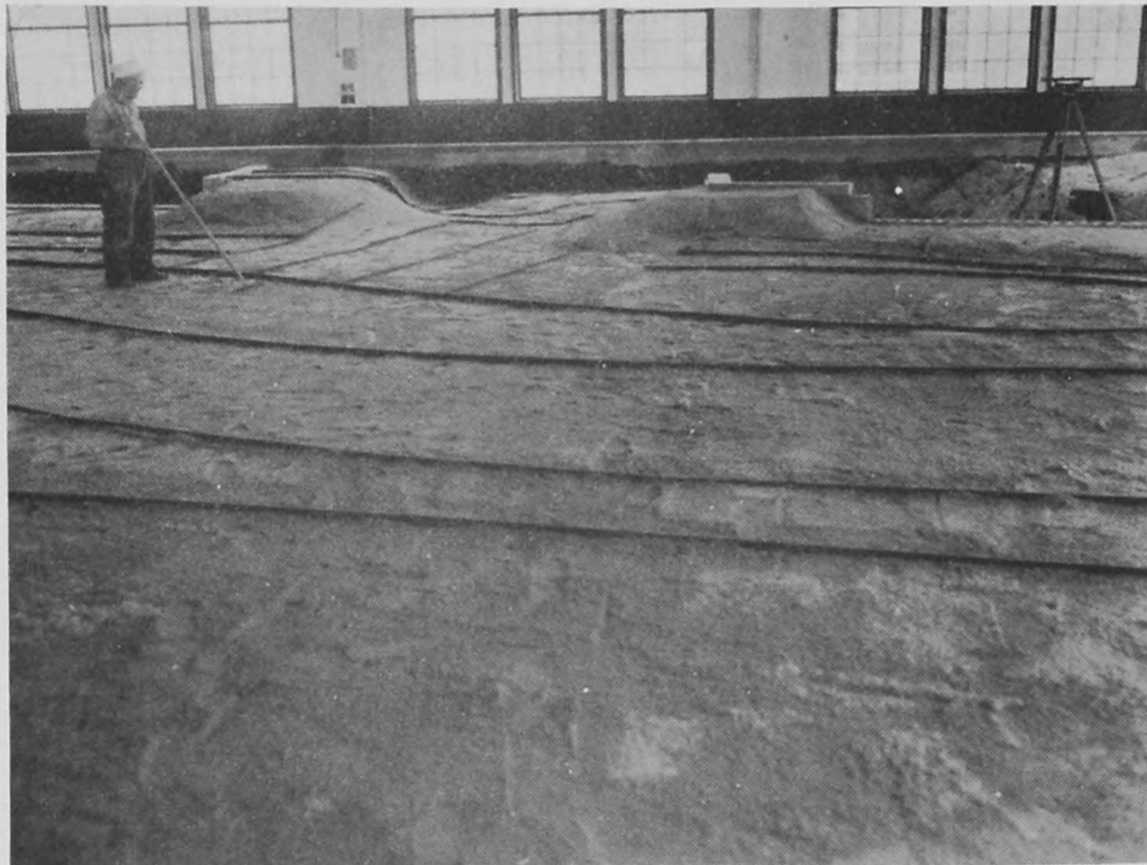
Figure 3. Templates and sand in place.
