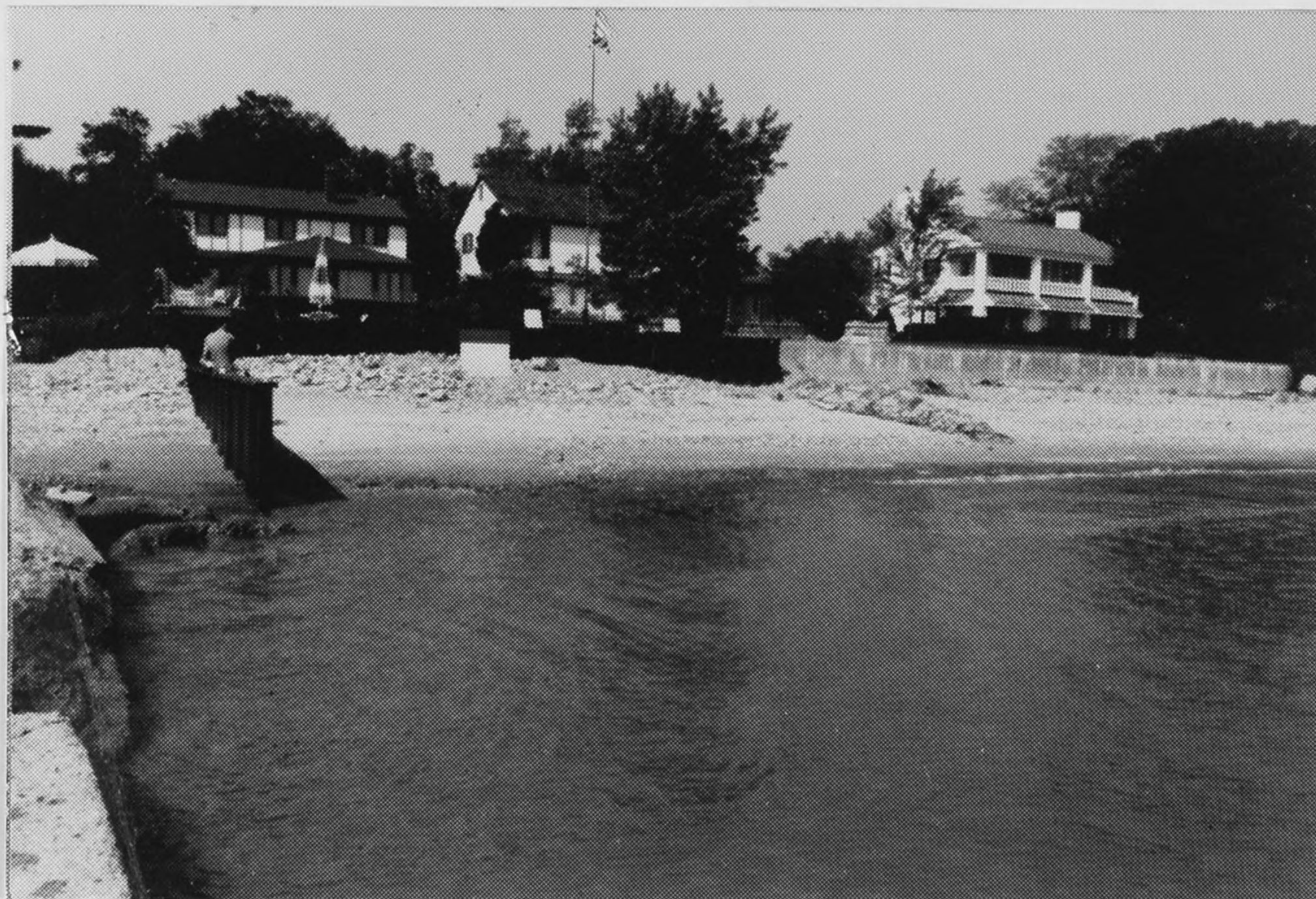
Figure B73. Site HH: Looking towards the southeast from north corner of Wines' beach. Remnant of old concrete groin extends beyond steel groin.
