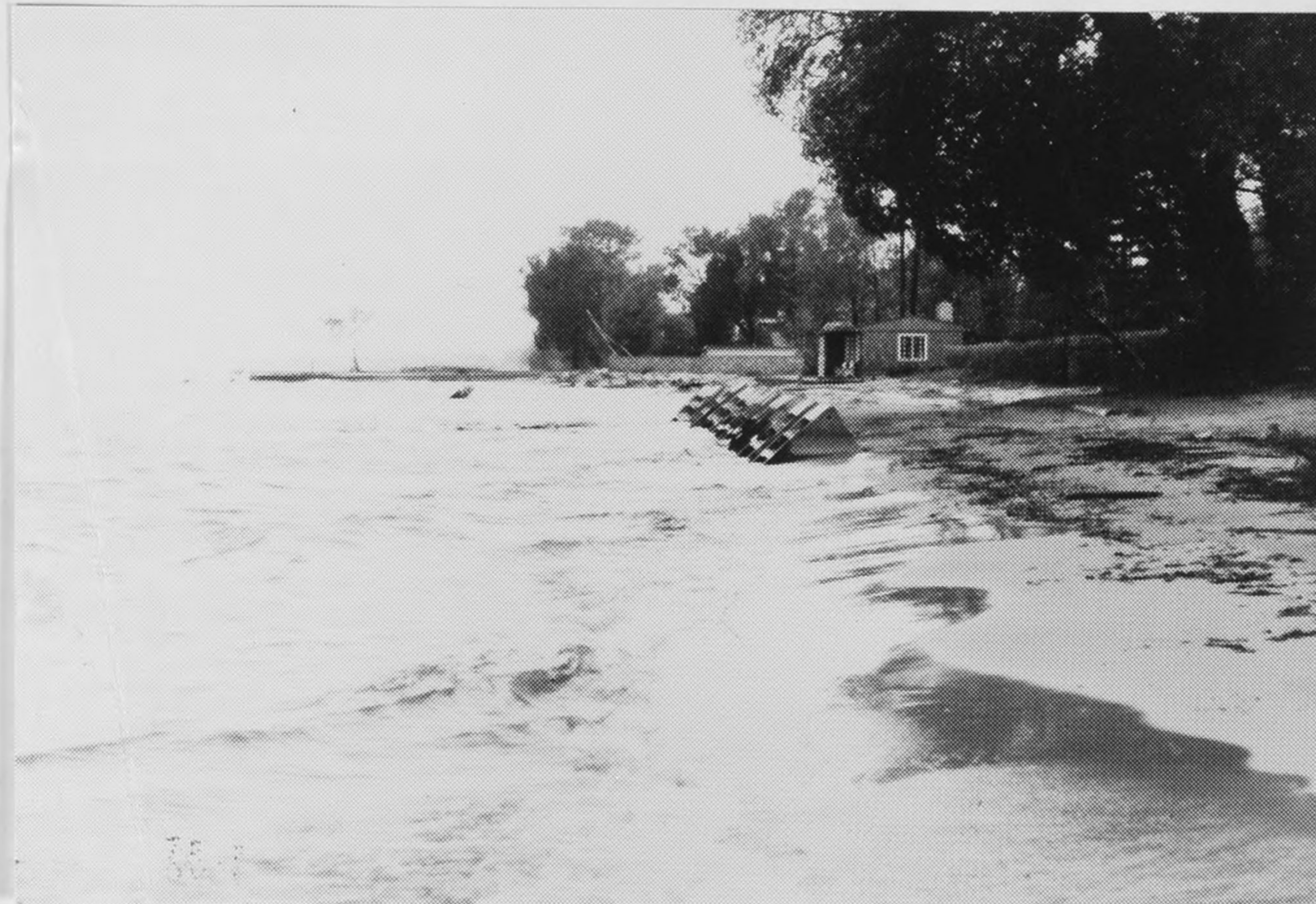
Figure B62. Site X: Looking south at wavebusters at 430 S. State. Note shore protection allows property to south to project farther lakeward.
