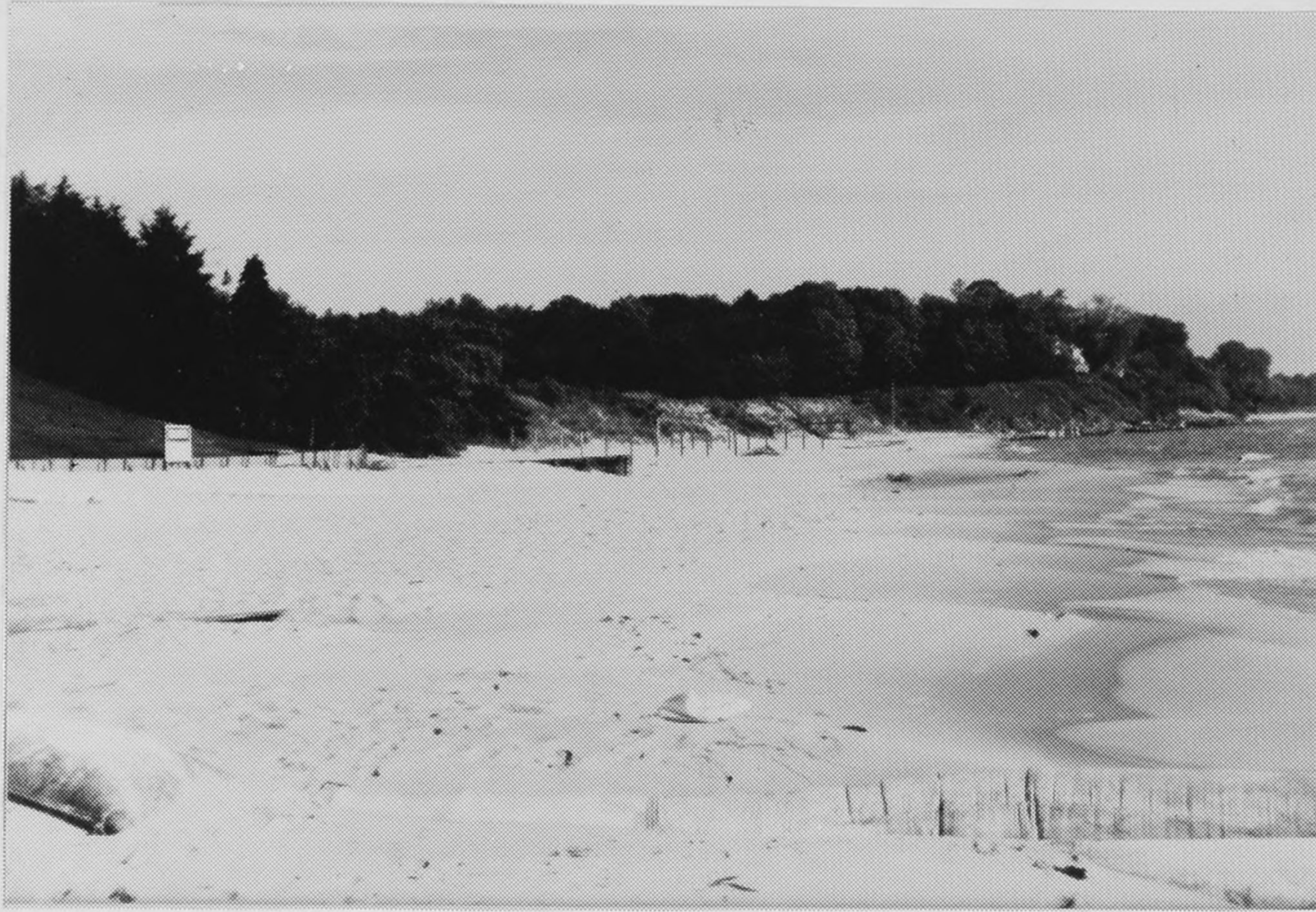
Figure B22. Site I: Looking south across Reid property, standing on Epworth property (site J). Tube groin on south side of Epworth property is in foreground, Light colored tube groin at center of property is barely visible below and right of sign. Timber groin at south side of property is also visible and note lack of beach farther south.
