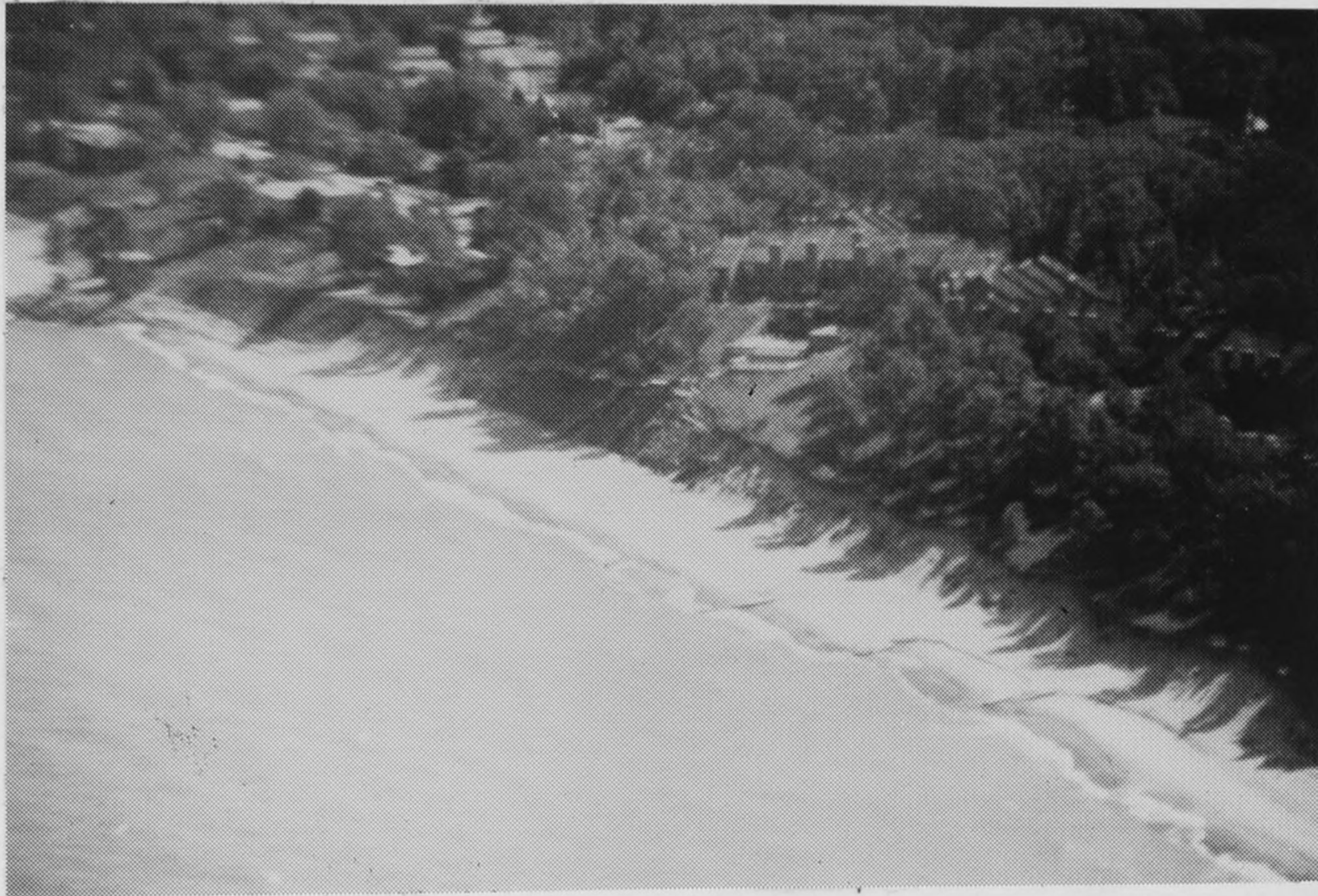
Figure B1. Site A: Aerial view of entire project. Note revetment in upper left of photograph, on northern side of property. Six to eight inch slump in beach visible as dark line in southerly two groin compartments in lower right side of photograph.
