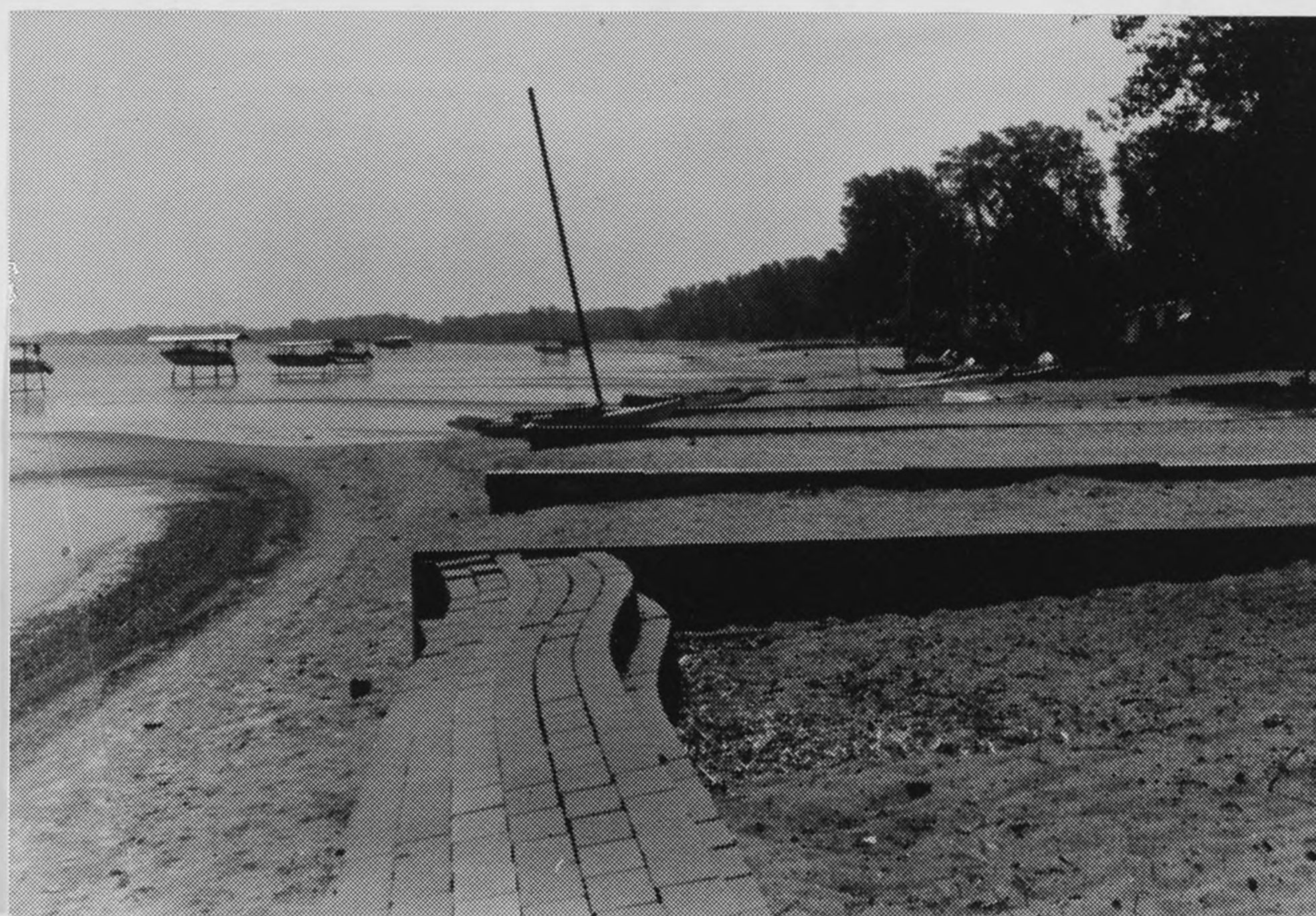
Figure B68. Site BB: Looking south towards site. Property is between two groins between catamaran and sandgrabber wall in foreground. Note sand spit offshore.
