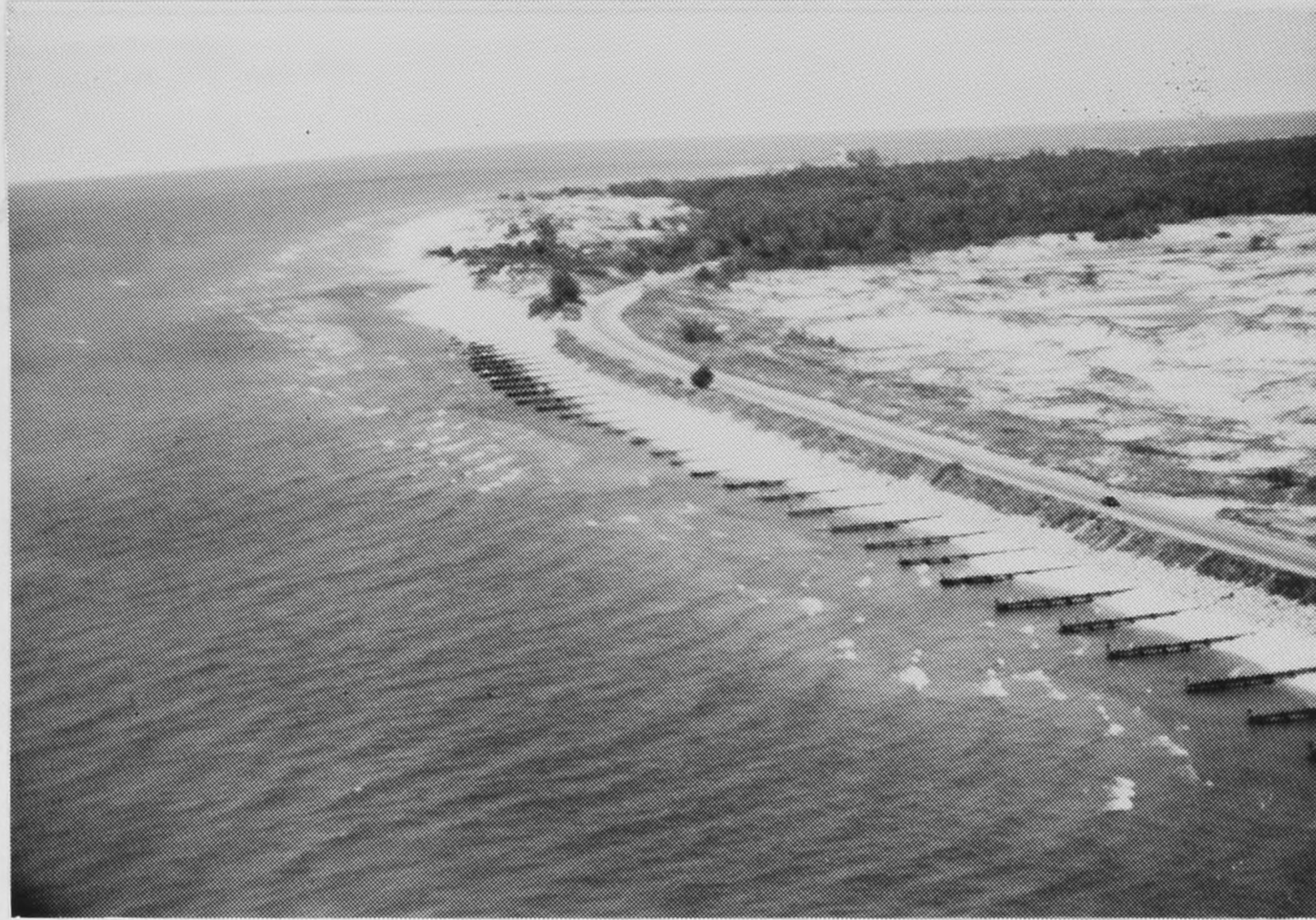
Figure B30. Site K: Aerial view somewhat to the north of Figure B29. Northern end of groin field only is visible. Note that some groins are almost completely filled.
