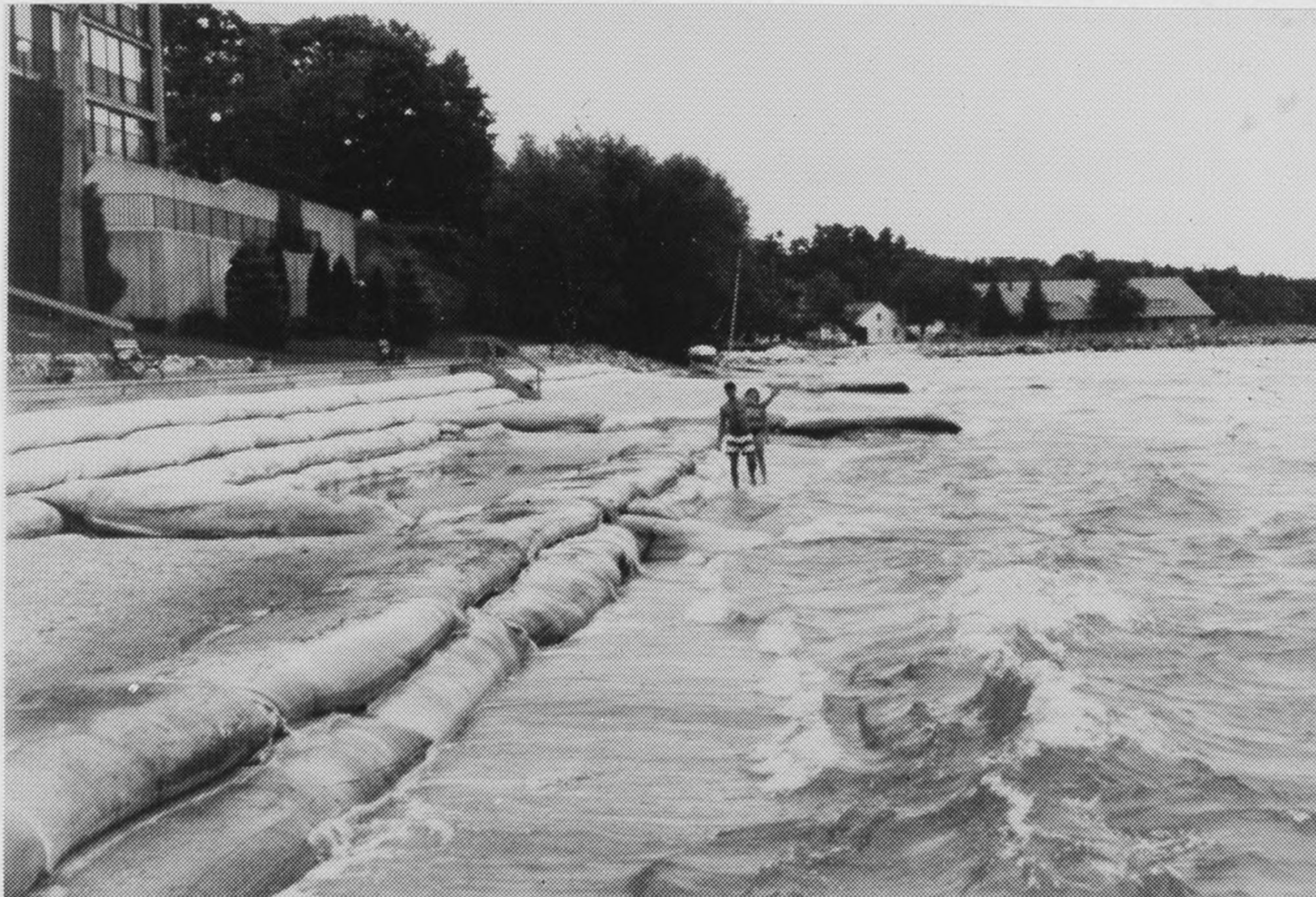
Figure B52. Site U: Looking towards the southwest from the most northerly groin in the system. Beach is higher behind bathers, may be due to artificial filling or littoral drift from the southwest.
