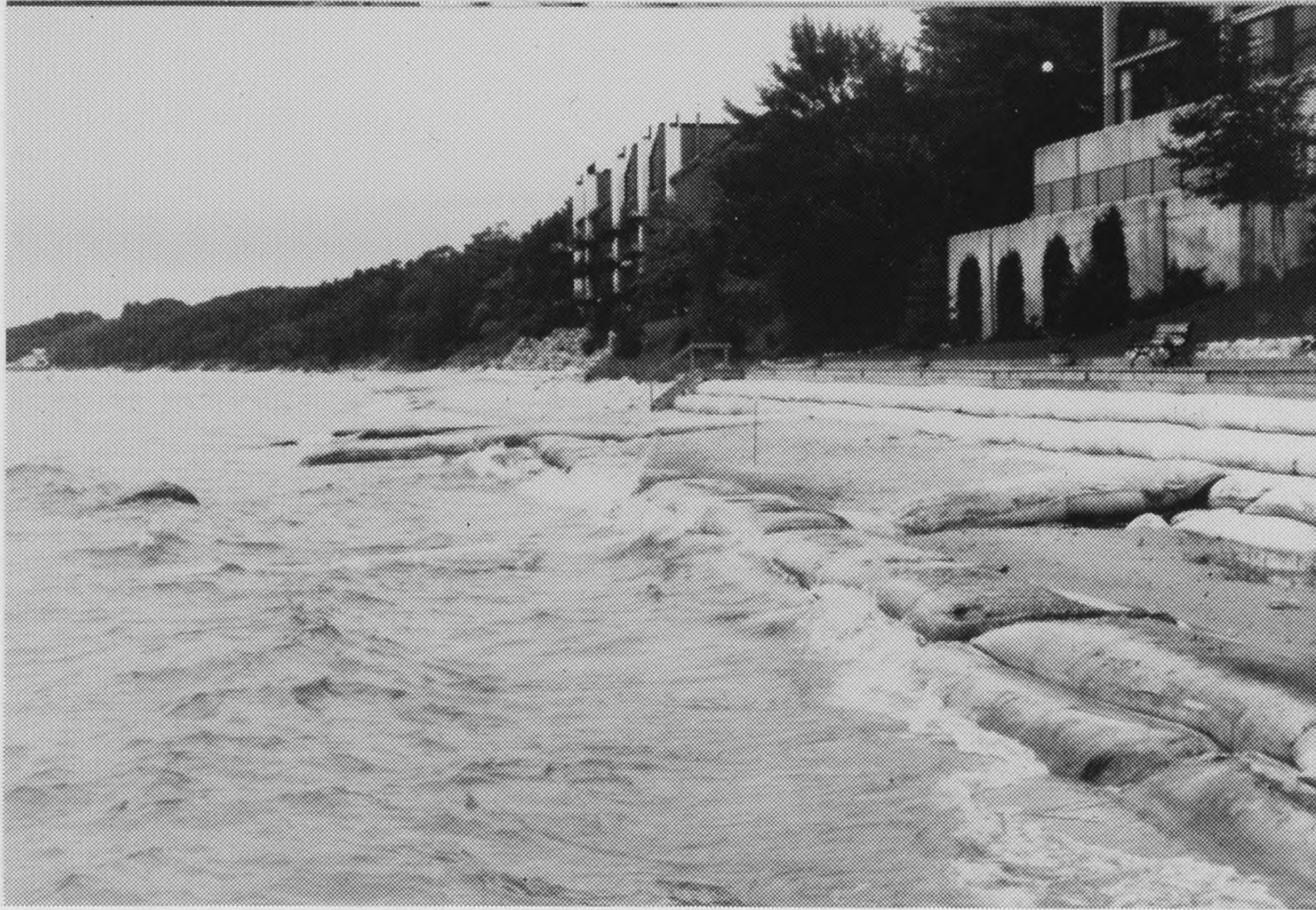
Figure B51. Site U: Looking northeasterly from same point as Fig. B50. Note sand filling behind offshore sill. Beach is beyond sill to the south of this location.
