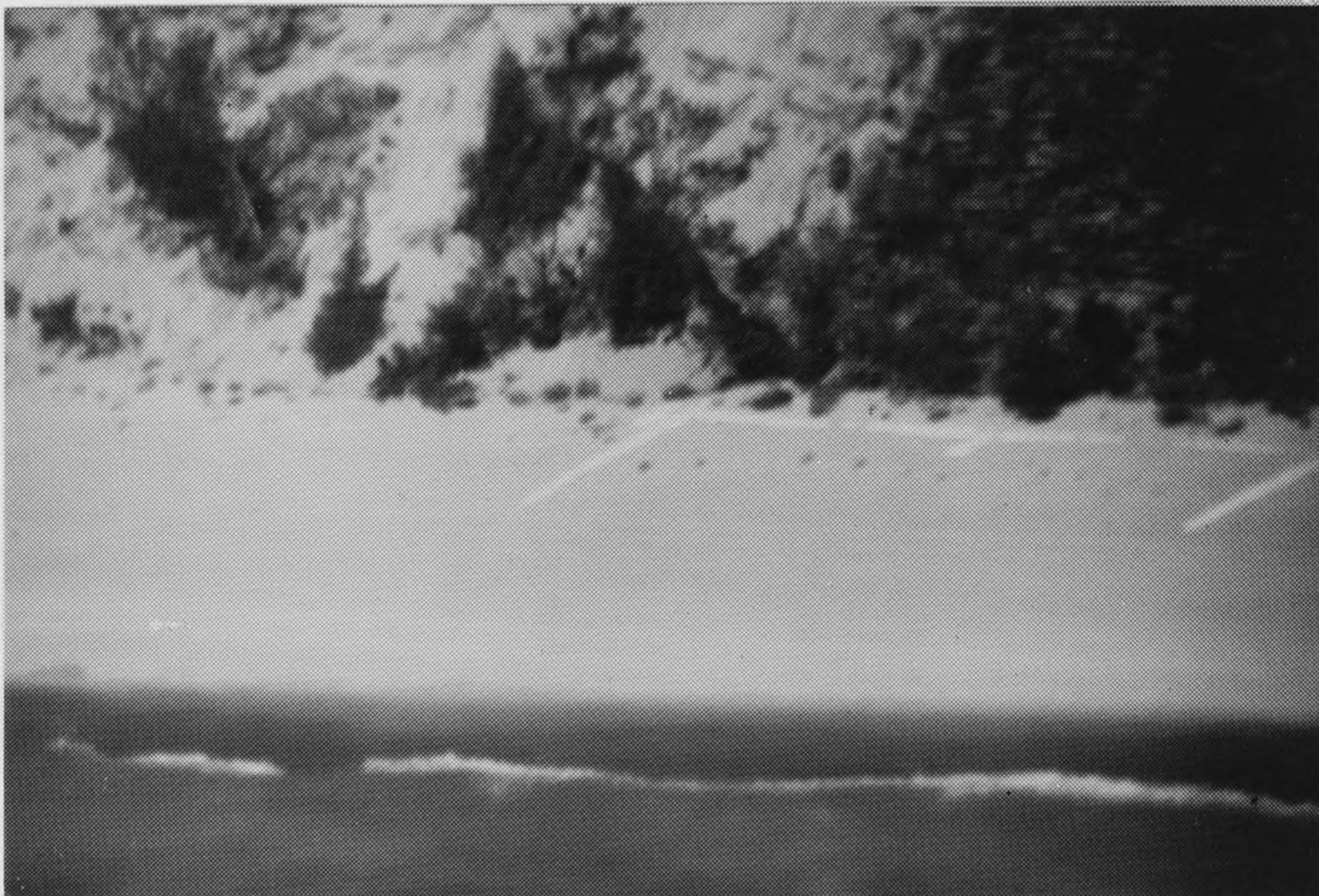
Figure B42. Site O: Aerial view of short revetment at north side of property. Recession of shoreline to north of revetment is visible at left center of photo.
