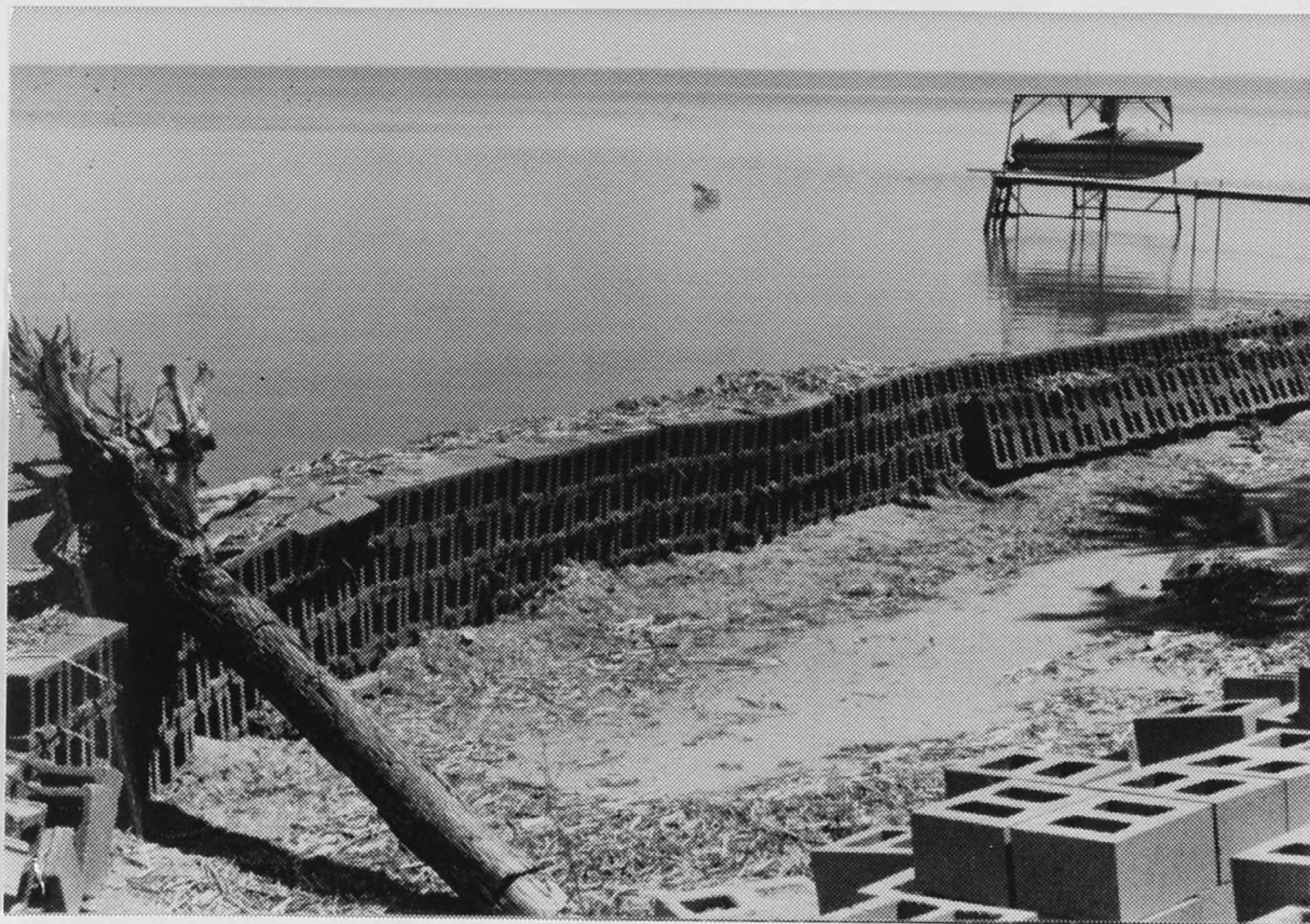
Figure B66. Site Z: Backside of sandgrabber wall, sand level behind slightly higher than in front. Also note tree trunk washed over wall during high water.
