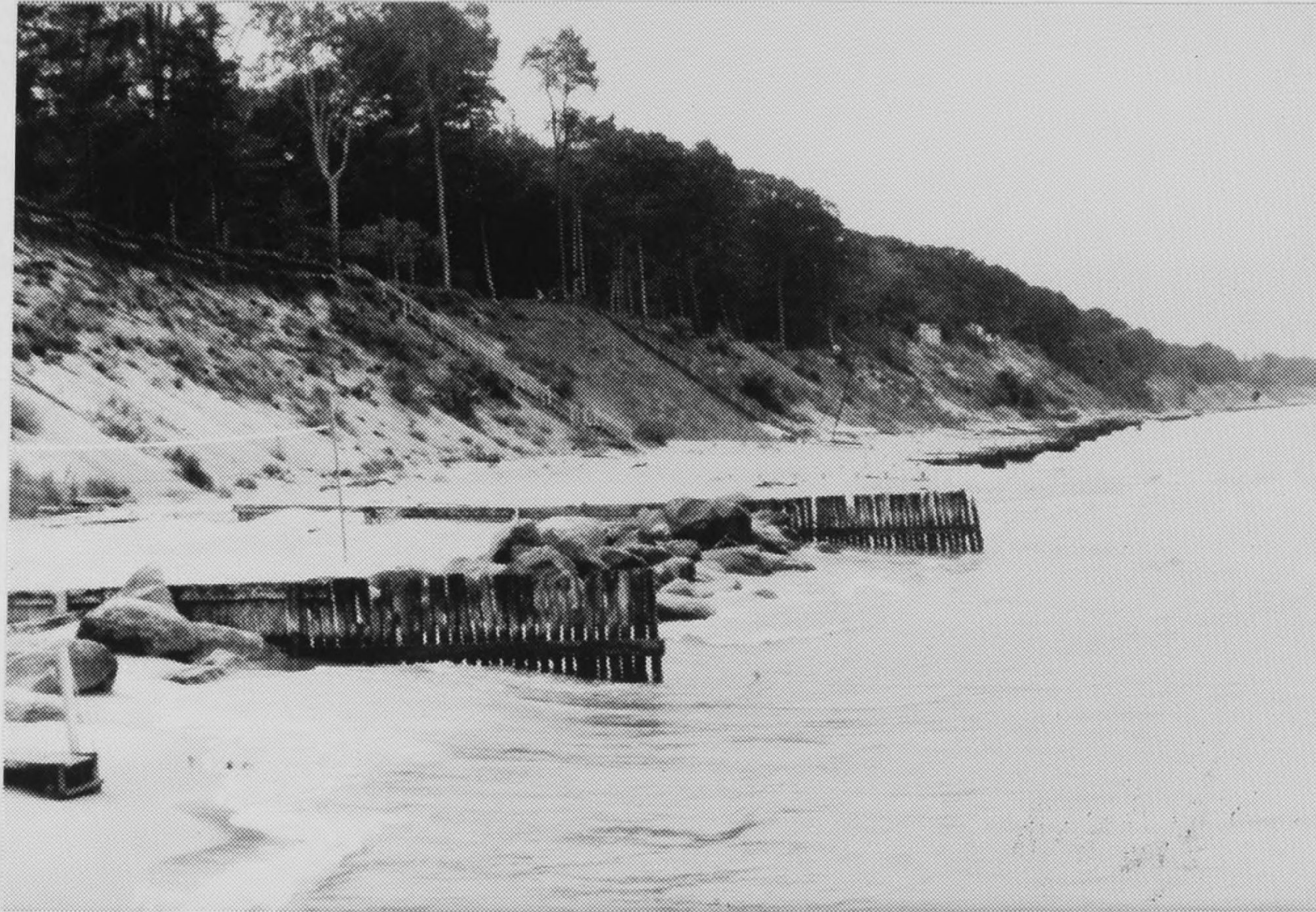
Figure B14. Site F: Looking south towards site from two properties to the north. Top of buried groin is immediately behind stone filled groin compartment in foreground.
