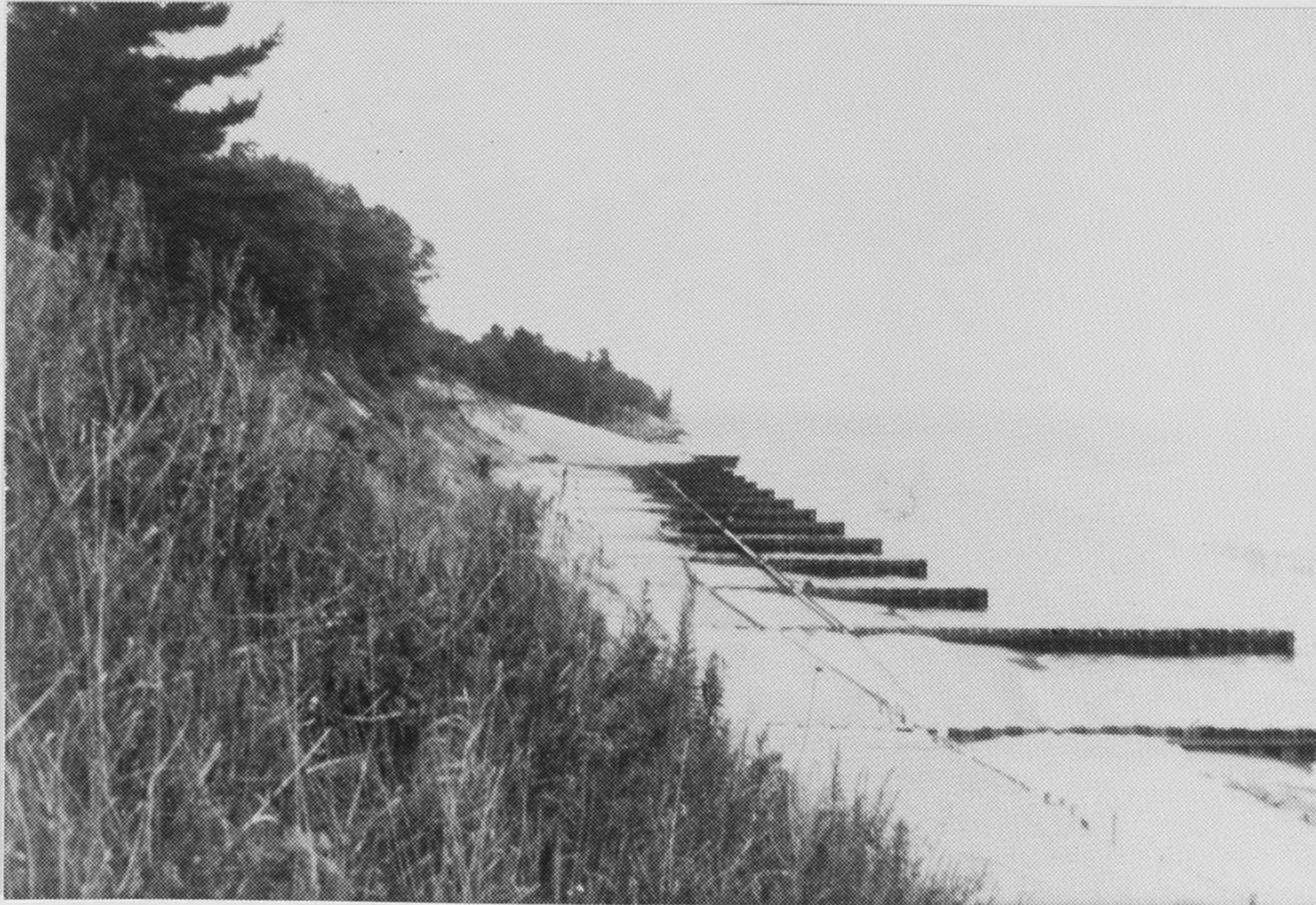
Figure B21. Site H: Looking towards southern end of property from approximately the middle of the groin system. Note that southernmost groins are shorter than the two closest ones. Wavebusters are present in lower right of photo.
