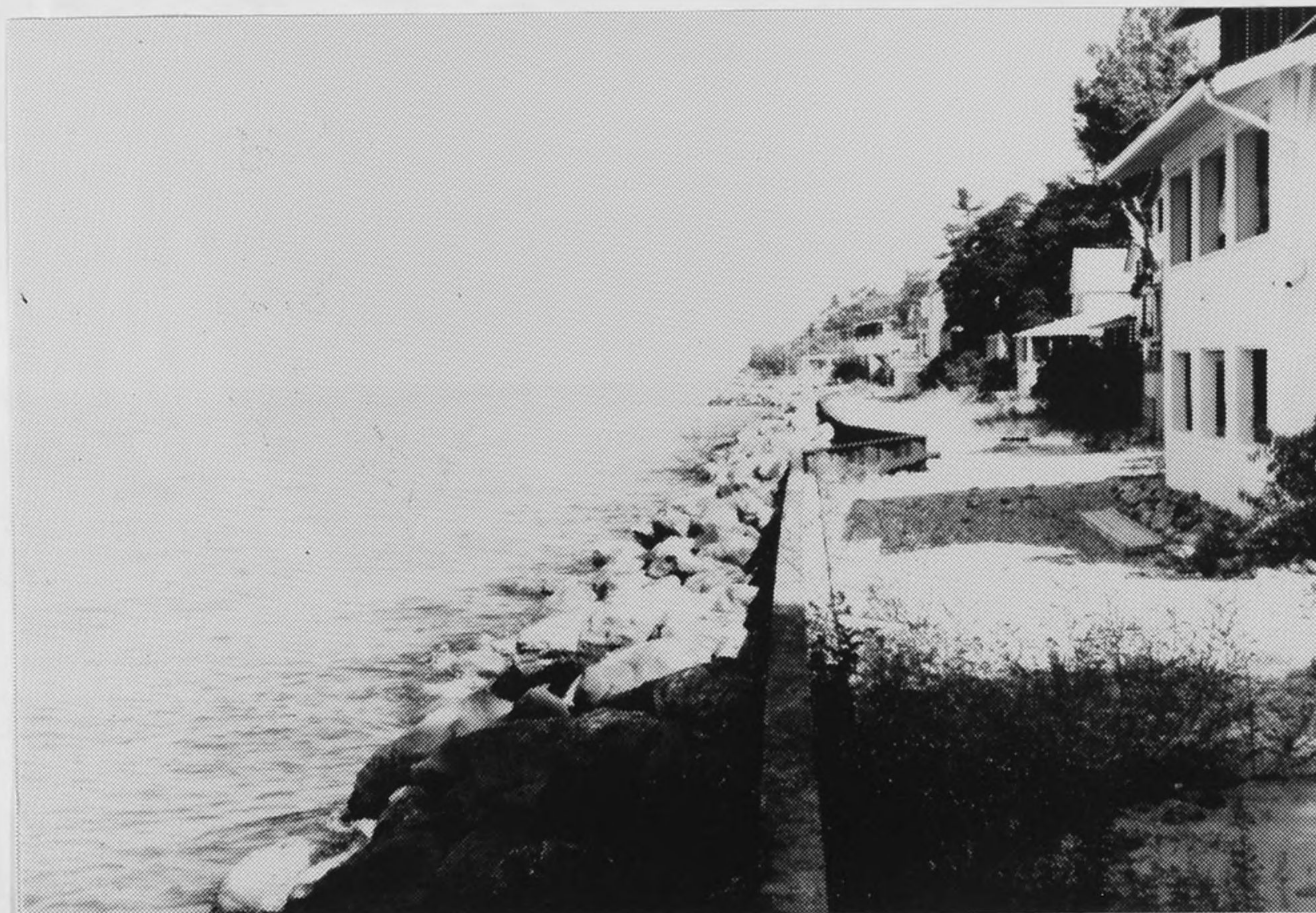
Figure B27. Site J: Closer view of revetment at location where it is backed by a retaining wall.
