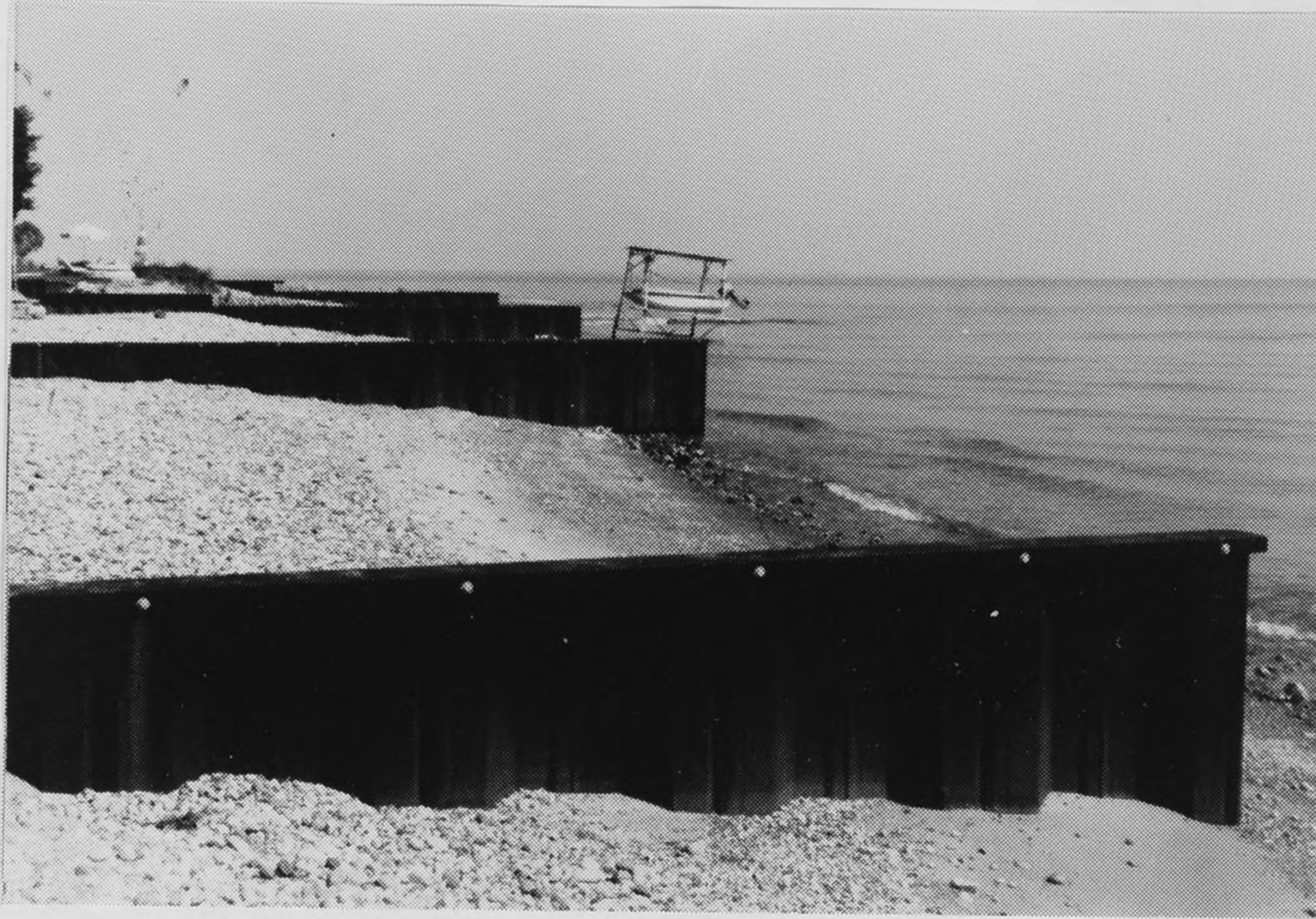
Figure B75. Site II: Looking north across system of groins from just south of property. Note beach nearly fills groin compartments and general coarse littoral material.
