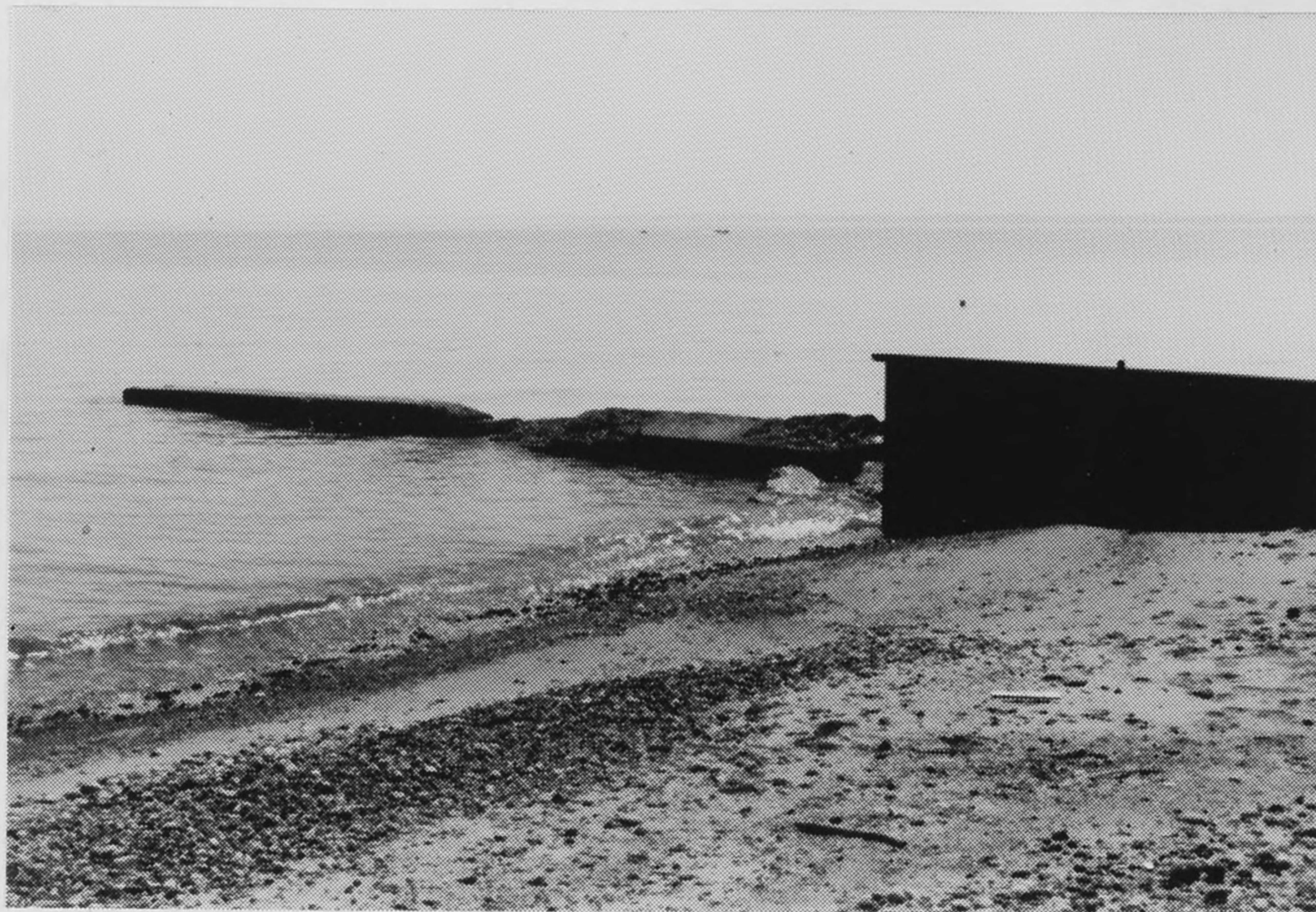
Figure B73. Site HH: Looking towards the southeast from north corner of Wines' beach. Remnant of old concrete groin extends beyond steel groin.
