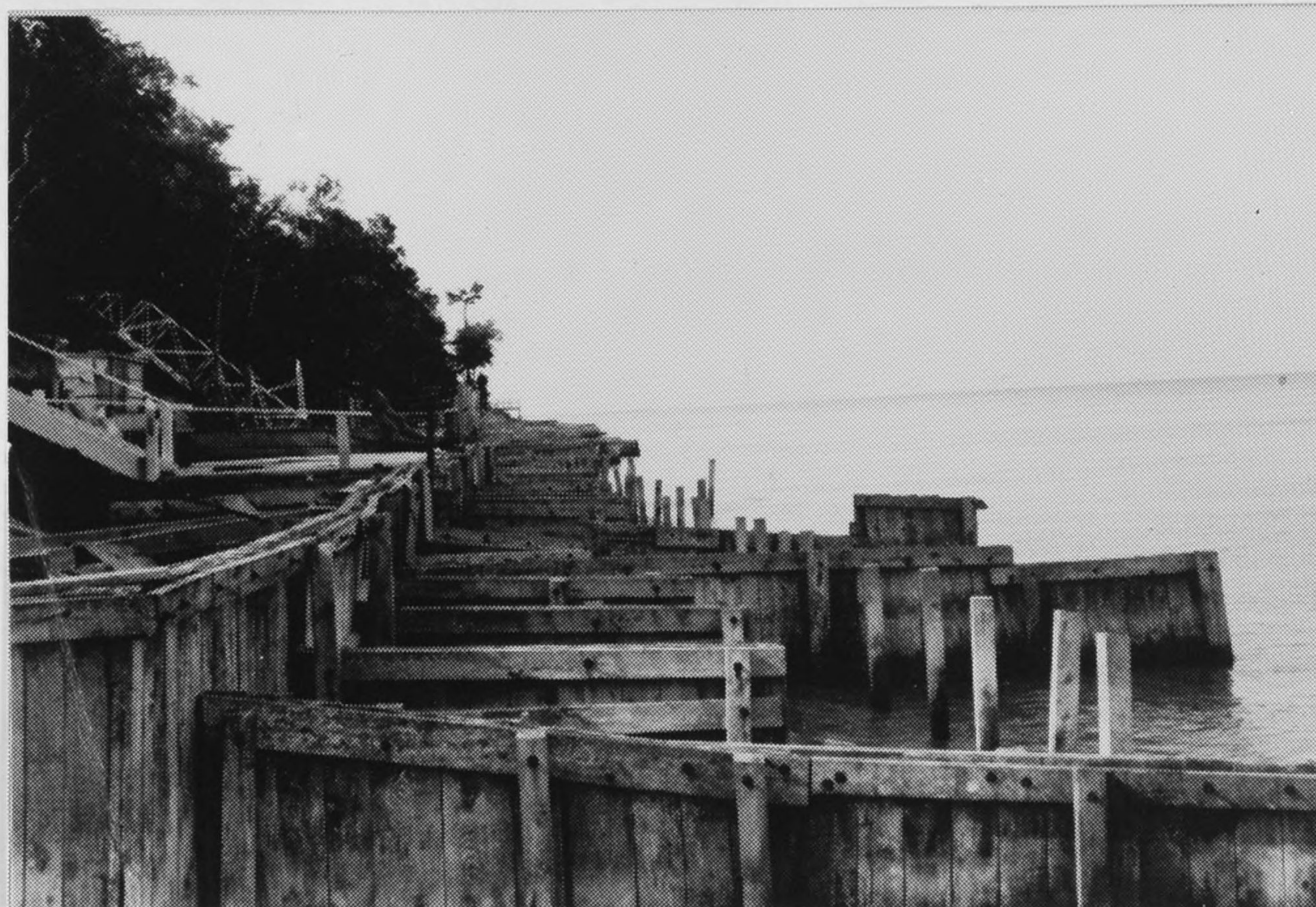
Figure B34. Site L: Looking north across site from the property to the south. Two groins and low retaining wall beyond high retaining wall are part of this system. Note other shore protection along shoreline.
