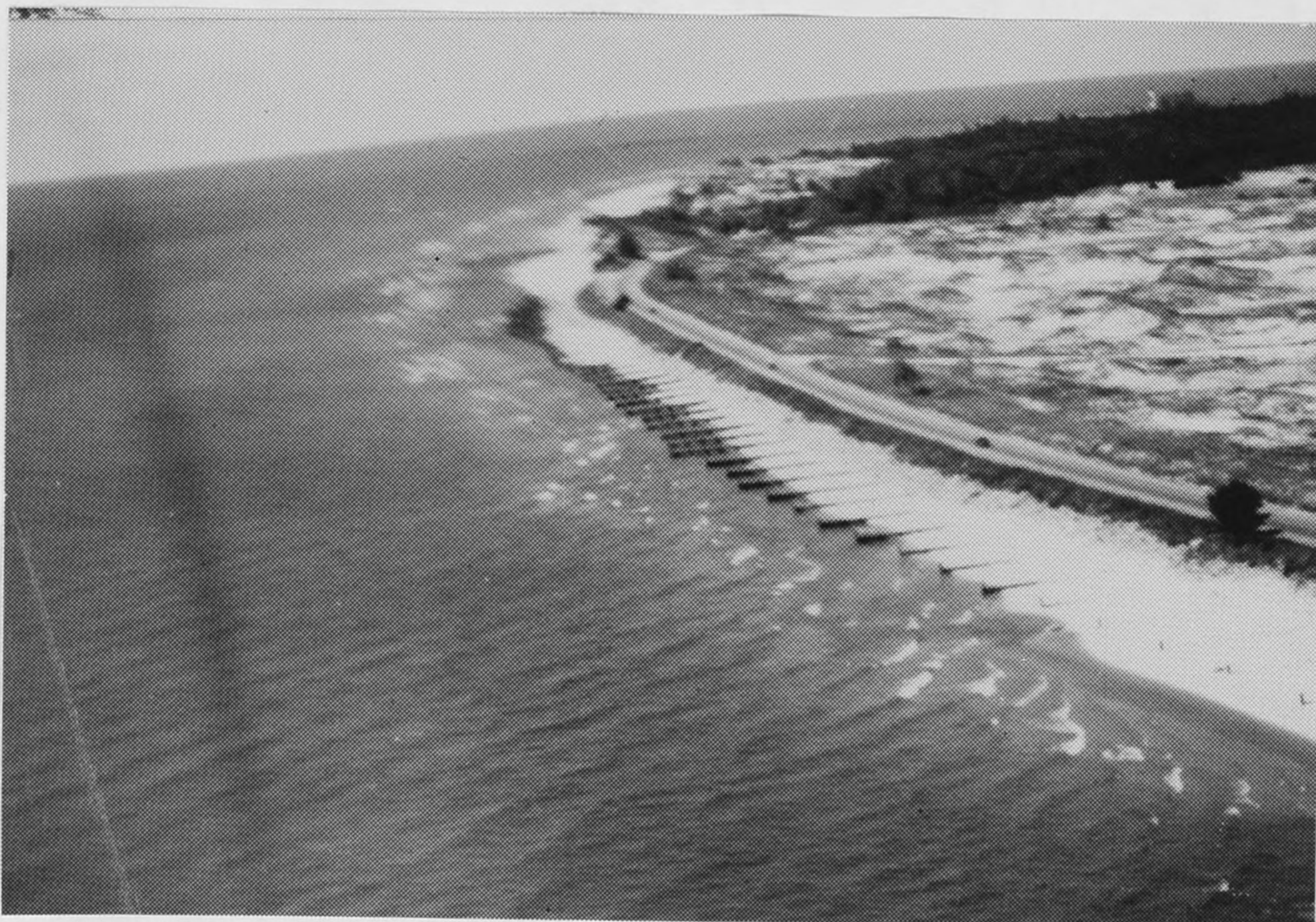
Figure B29. Site K: Aerial view of southern end of long groin field. Note that groins in southern portion of groin field at lower right are completely filled.
