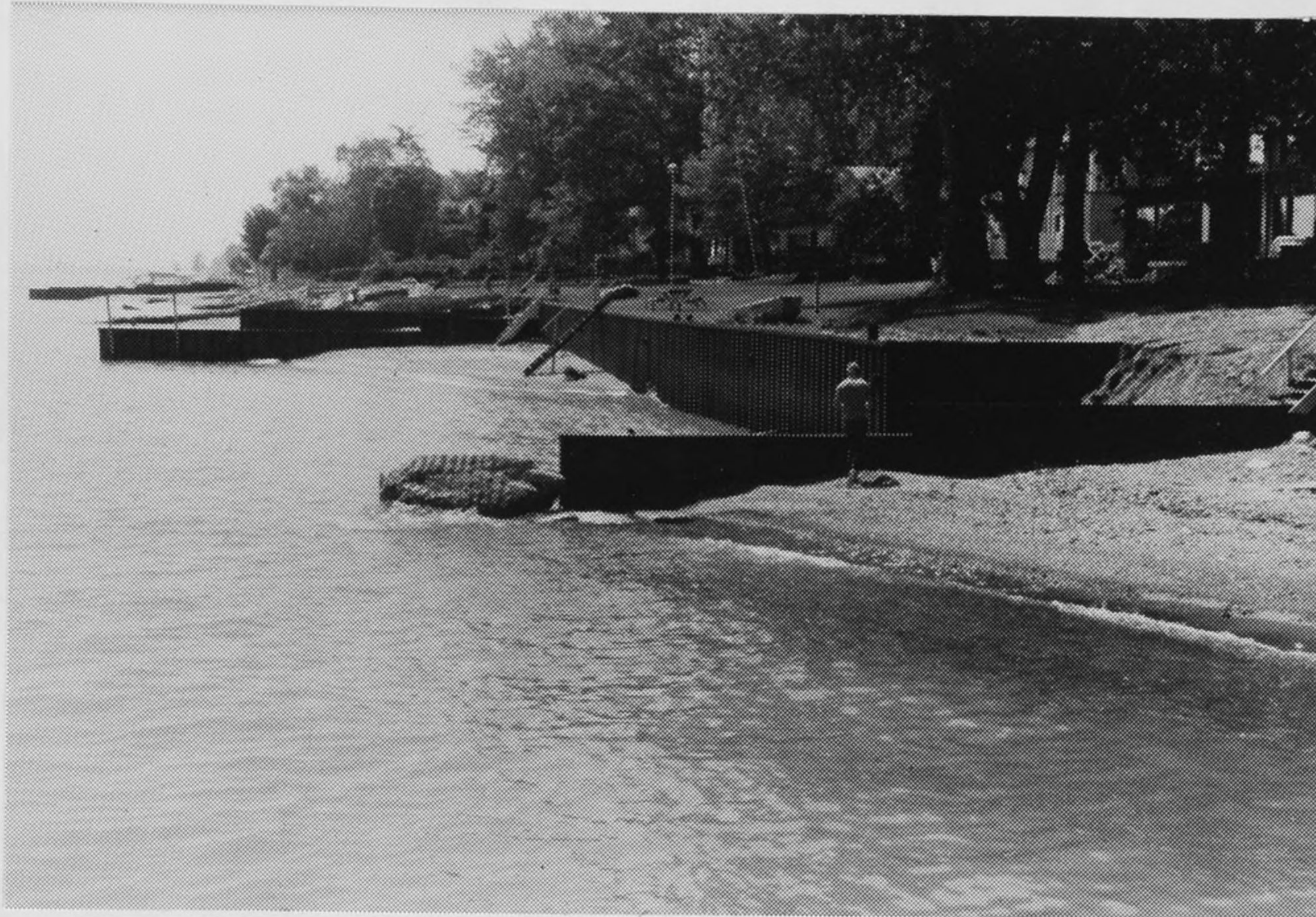
Figure B69 Site DD: Looking south across Sharpe property. Existing groin with large boulder in front is their groin. Note small sand fillet in corner of seawall-groin system immediately to the south. Also note that Sharpe groin does not project as far lakeward as the groin to the south or the groin from which the photo was taken.
