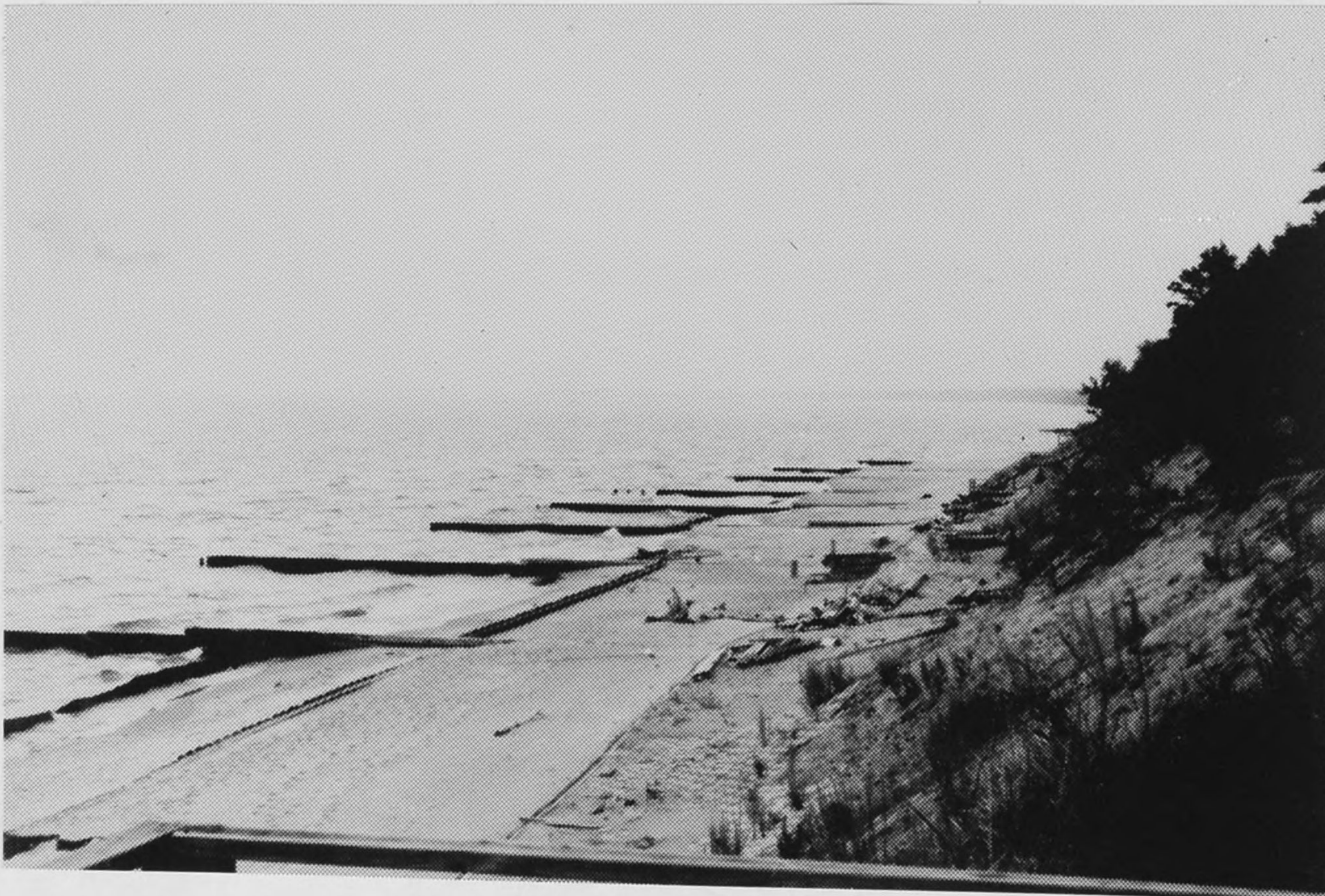
Figure B19. Site H: View towards the north of the last eight groins at the northern side of the system. Tops of wavebusters are visible at lower left side of photograph. Flex-blocks are visible in foreground at toe of bluff.
