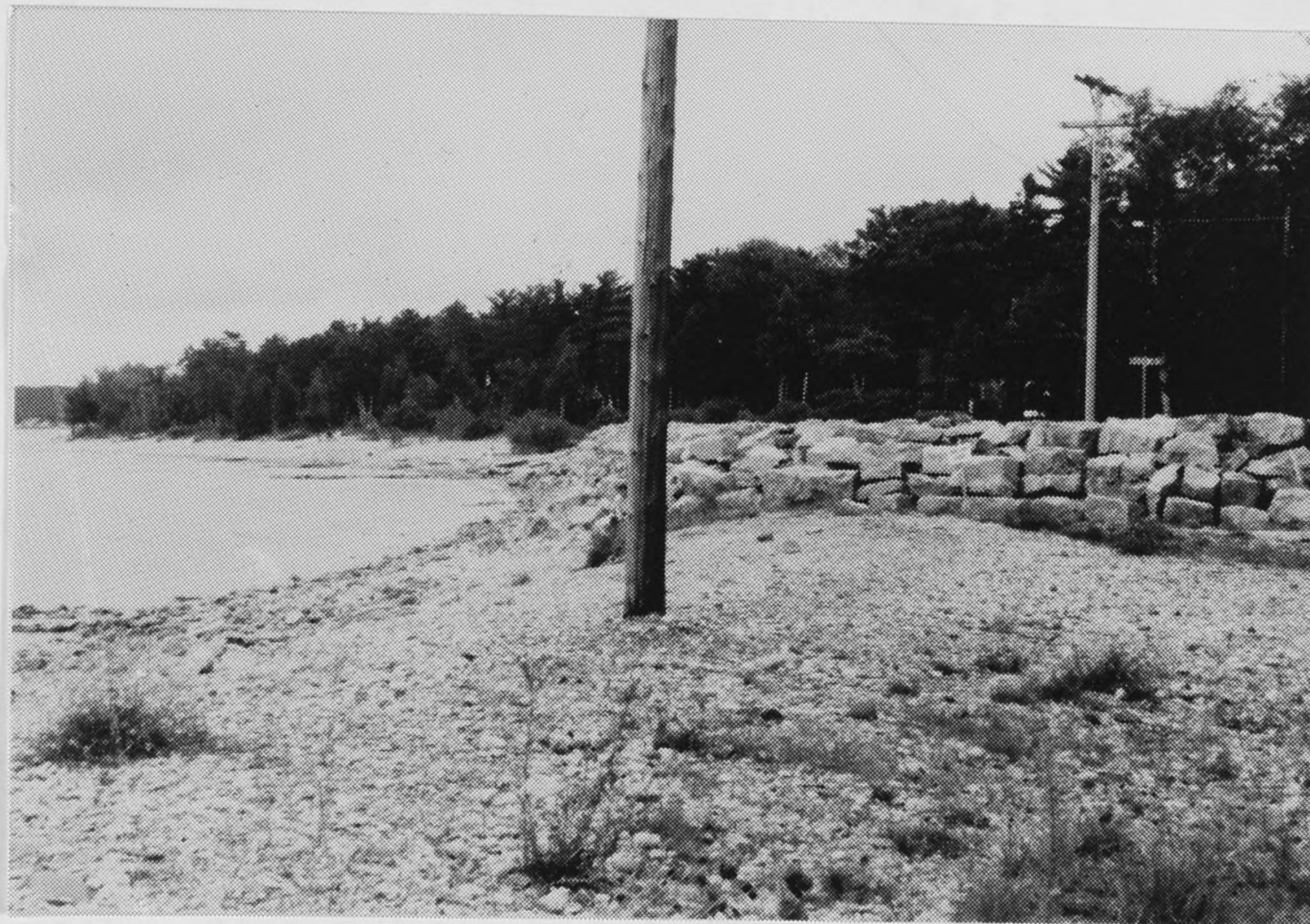
Figure B58. Site W: looking at southwestern side of revetment.
