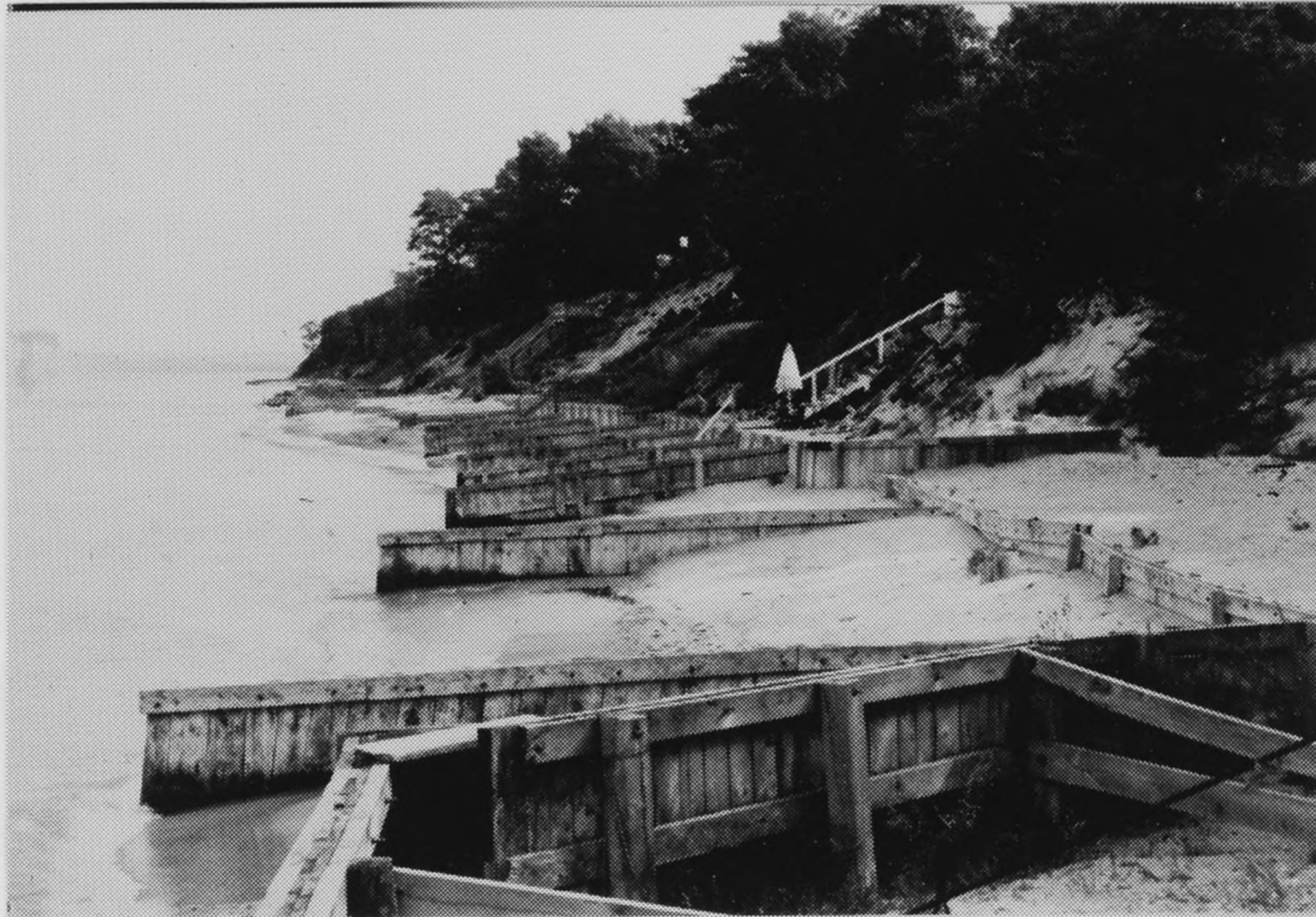
Figure B34. Site L: Looking north across site from the property to the south. Two groins and low retaining wall beyond high retaining wall are part of this system. Note other shore protection along shoreline.
