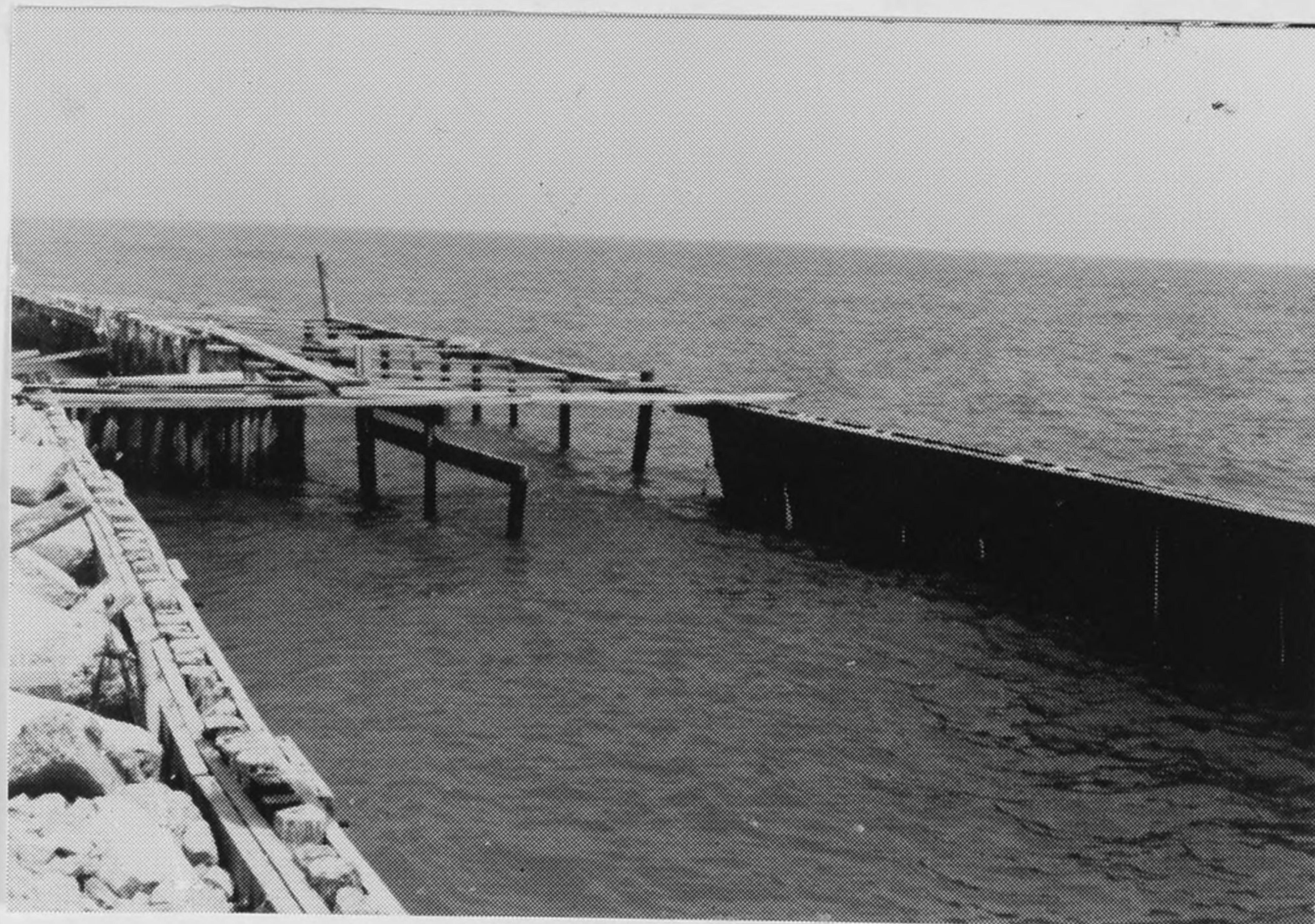
Figure B64. Site Y: New wall construction at Heller property.
