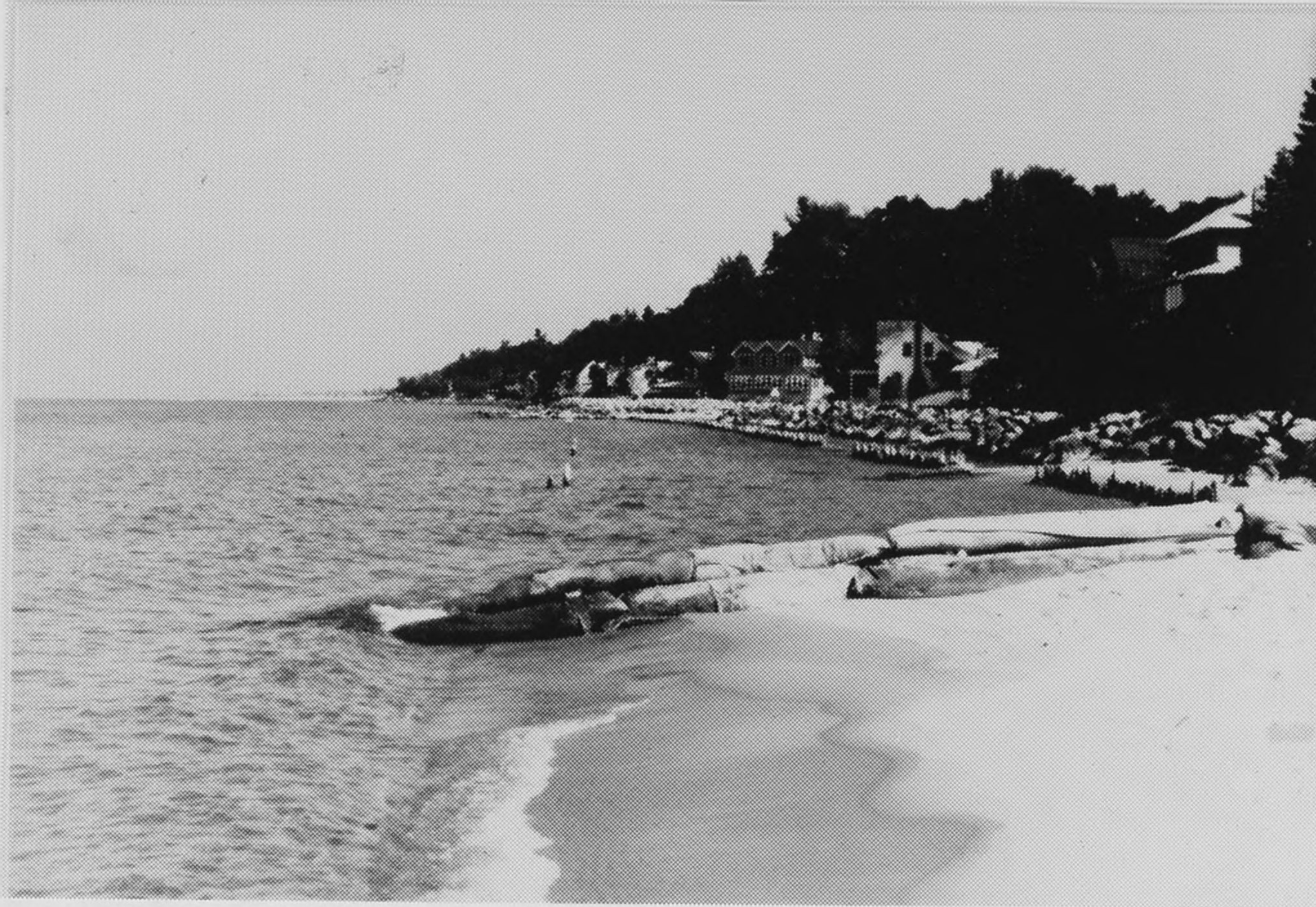
Figure B24. Sites I and J: Tube groin (part of Reid permit) on south boundary of Epworth property. Note accumulation of beach on south side of groin and slight accumulation behind other tube groins to north (in vicinity of old timber retaining wall).
