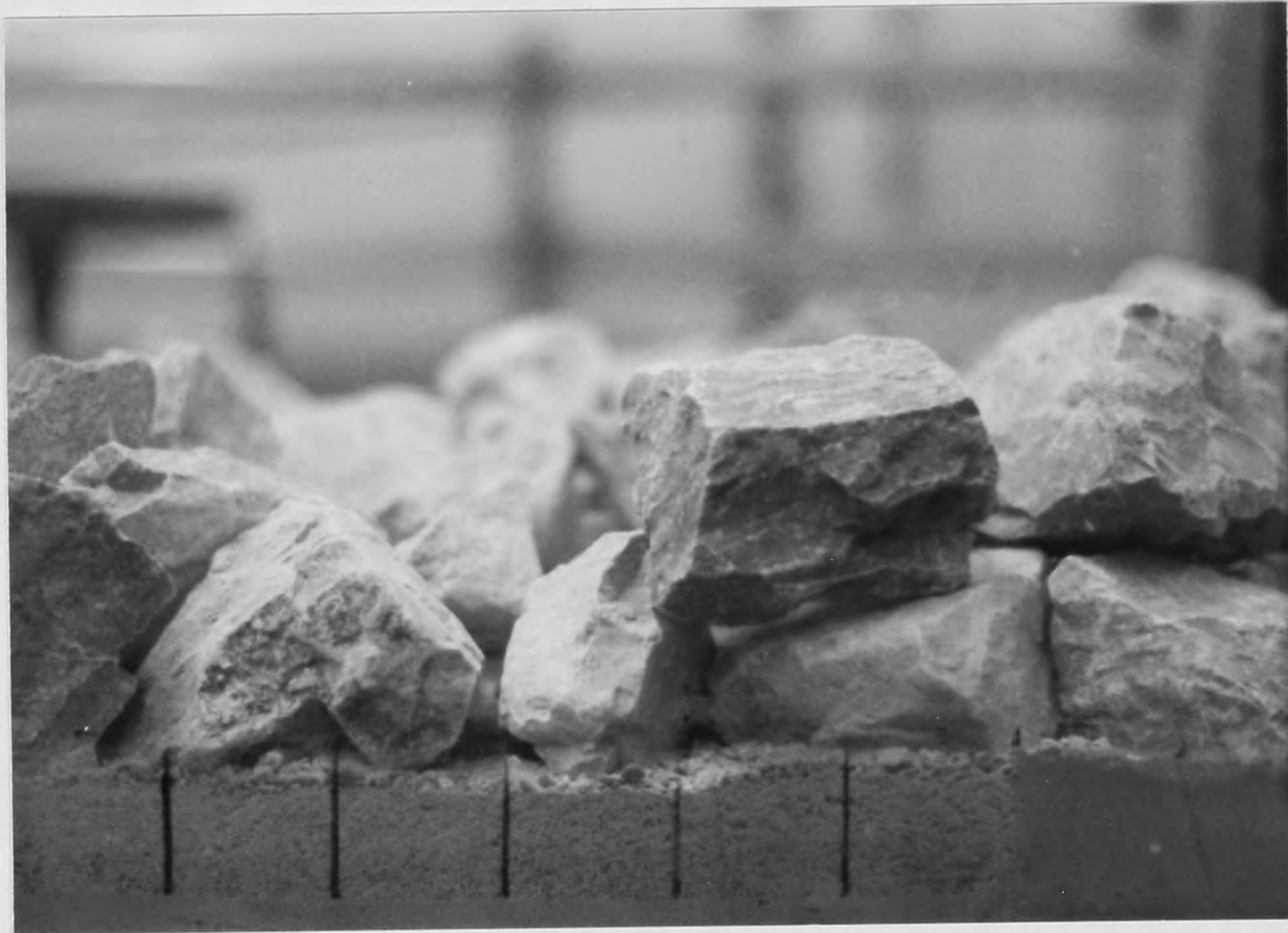
FIG. 3. Intermediate Stage of Test Section Construction (Placement of 4 inches of 2-4 inch Armor over Sand Isolation Layer)
