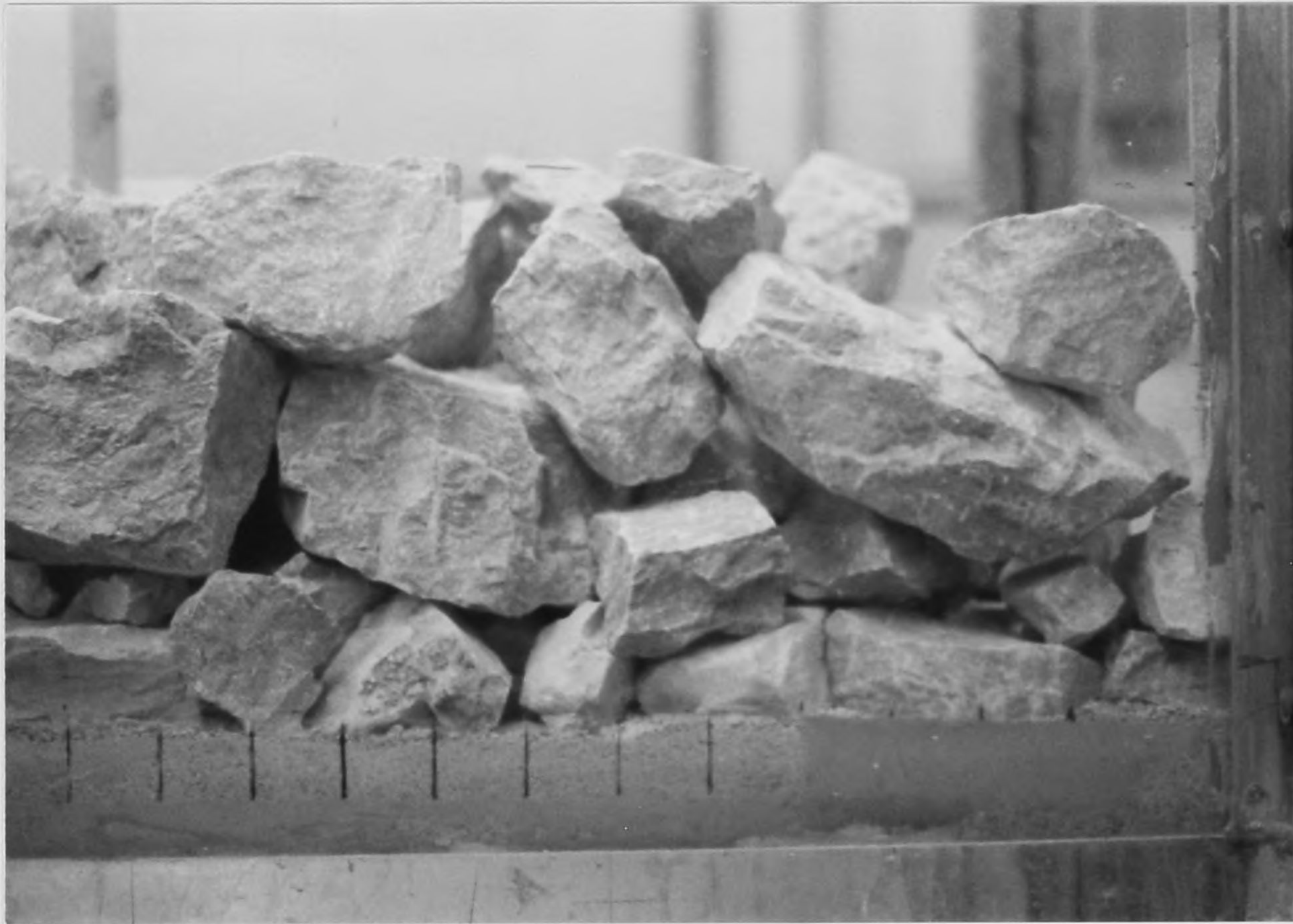
FIG. 4. Completed Test Section (With Final Layer of 4-8 inch Armor Layer)
