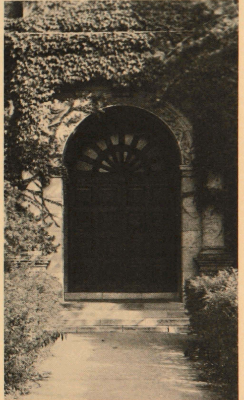
Before renovation this entrance to the Lawyers Club was daunting to people in wheelchairs.
