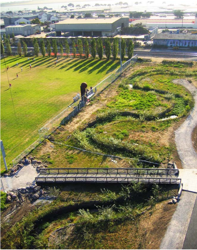
Figure 6. An example of a channel reconfiguration project to restore a 300-m stream reach from a straight, concrete-lined ditch. The high sinuosity design was based on patterns observed on nearby creeks with similar slopes in historical aerial photographs. Since then, the watershed has undergone substantial urbanization, so the project on the Lower Codornices Creek in Berkeley, California, will serve as an experiment to see how this historical shape evolves under changed conditions. Photo by Cris Benton.
