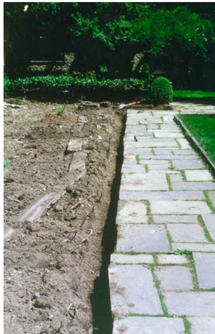
Replacing the walkway edging
