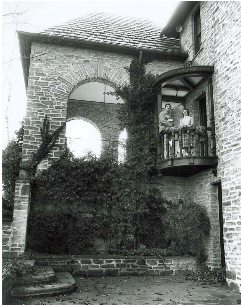
Students looking out from the balcony
