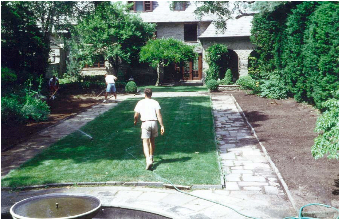
Raking down the new topsoil
