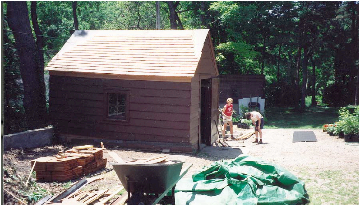
Replacing the roof of the shed
