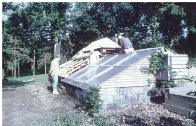
Replacing the fiberglass windows on the coldhouse
