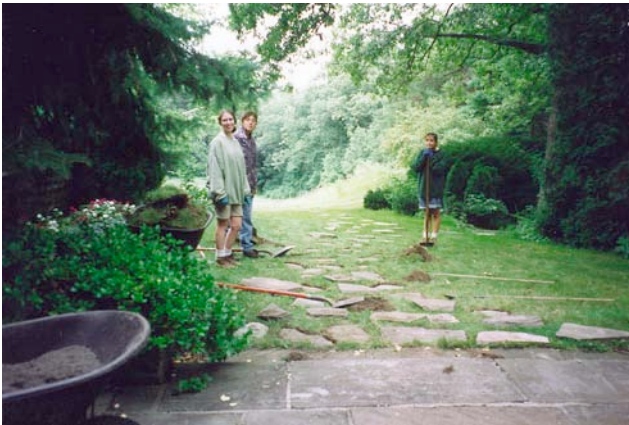
Laying the stone for walkways
