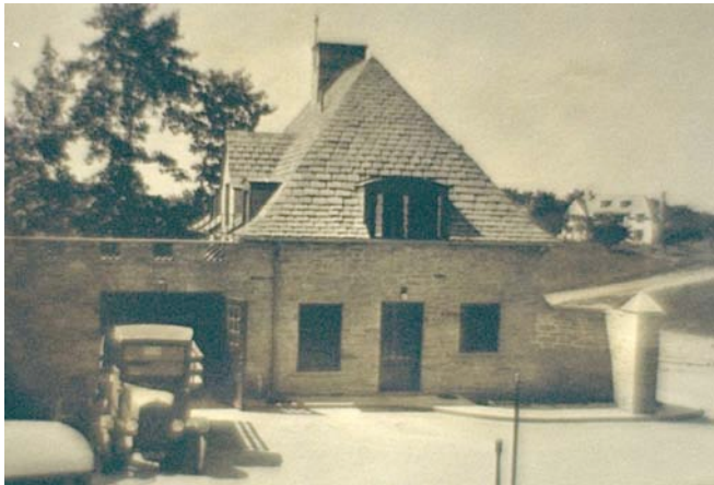
The caretaker's cottage
