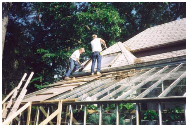
Replacing the shop windows
