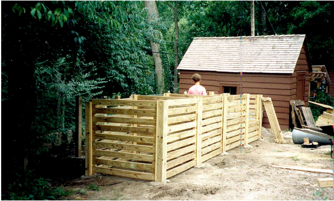
Building the new compost bins
