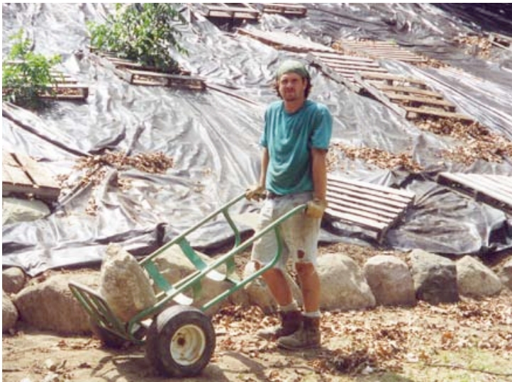
Laying the stones at the base of the bank
