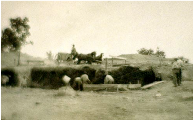
Excavation of the foundation (by mules)
