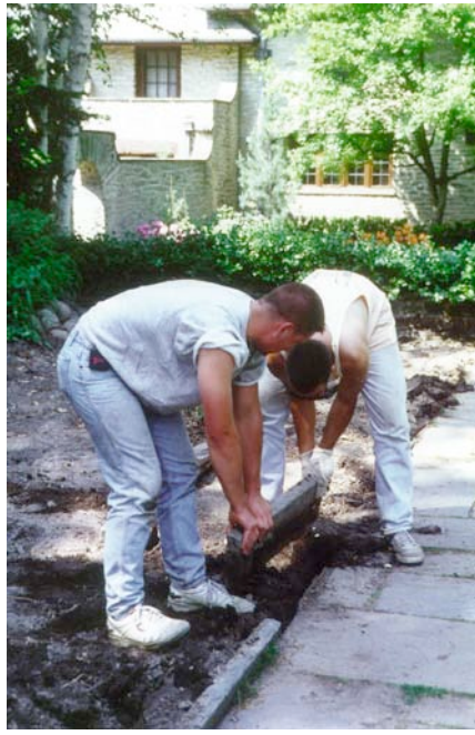
Placing the edging stones in the formal gardens
