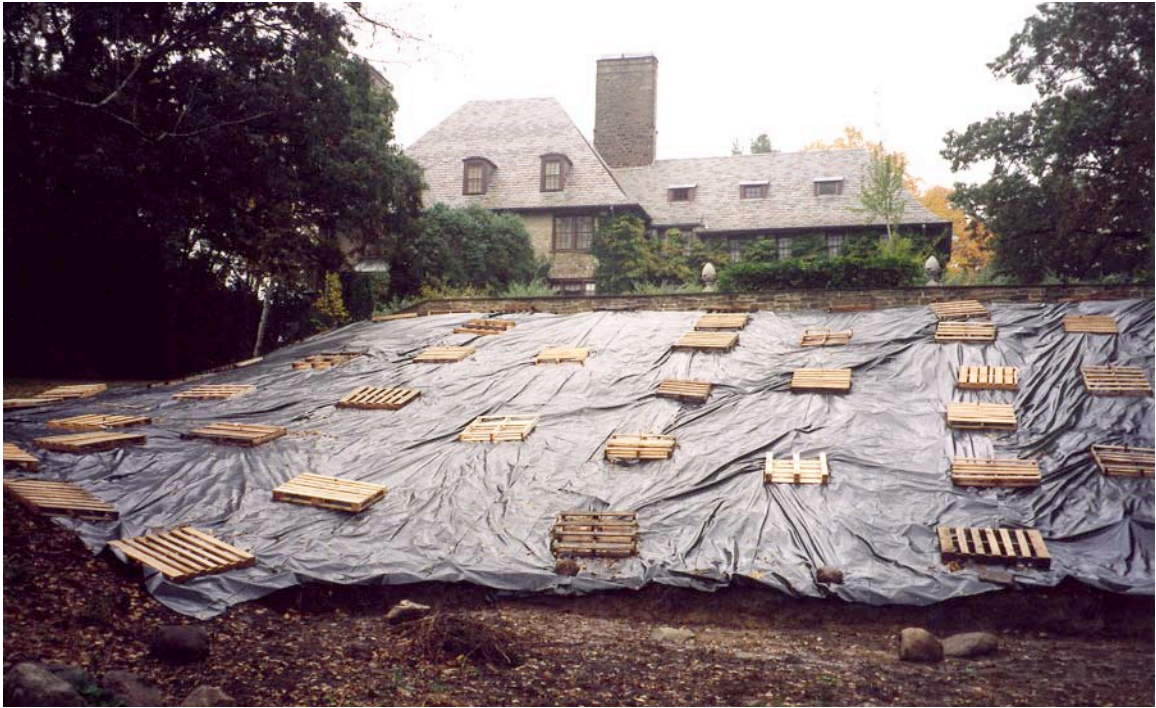
Covering the bank with plastic tarp
