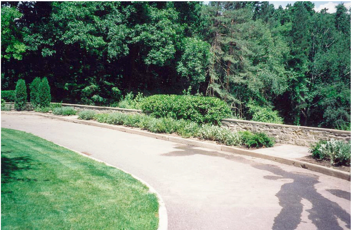
Relandscaping the front circular drive
