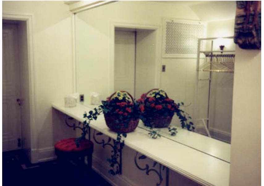
The ladies powder room after renovation
