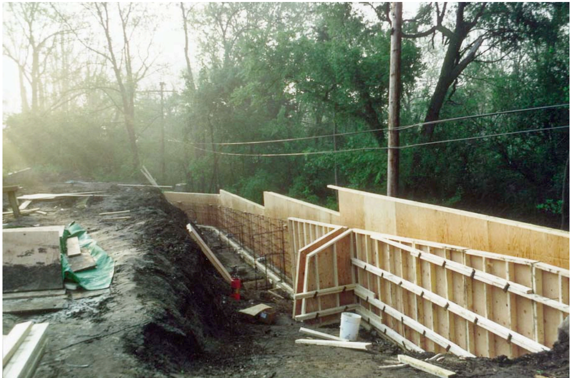
Replacing the retaining wall
