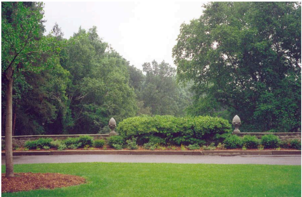
Placing the ornamental elements
