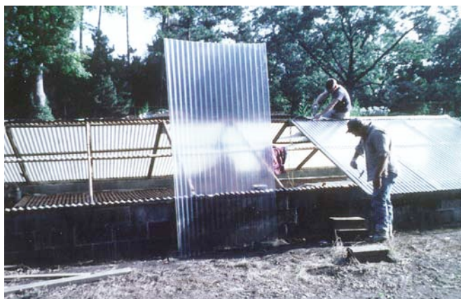
Replacing the fiberglass windows on the coldhouse
