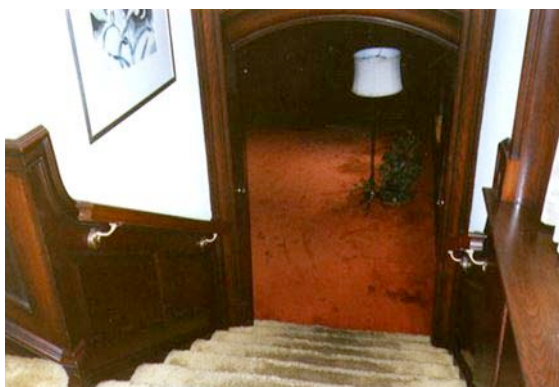
The threadbare staircase
