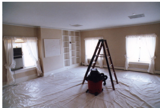
Stripping all the color from the house
