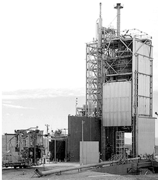
The Kiwi nuclear reactor test stand
