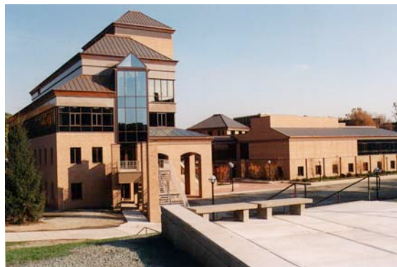
The Lurie Engineering Center
