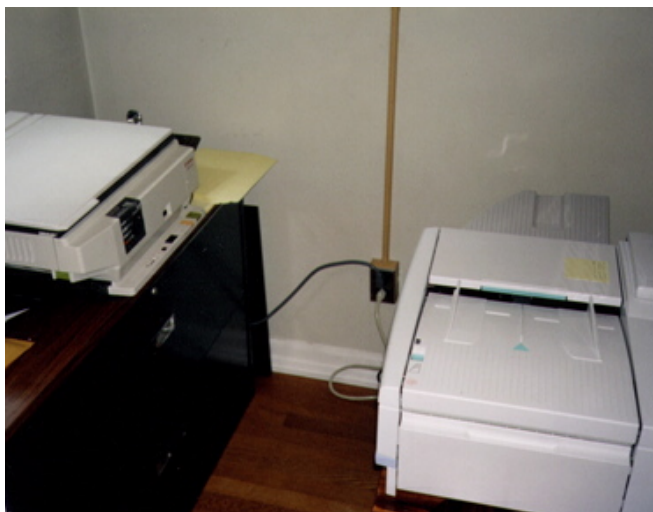
The telecommunications center in The President's House
