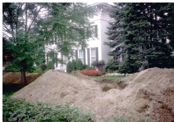
Trenches surrounding the house
