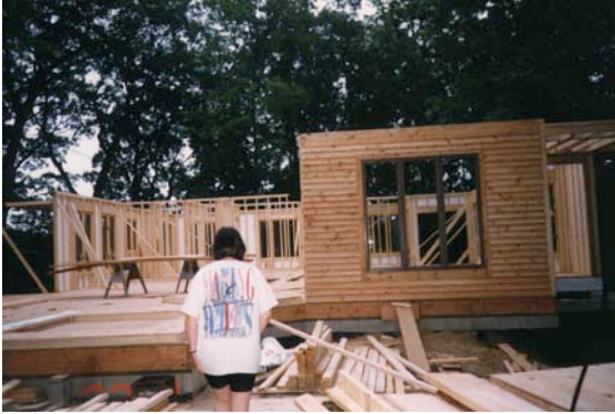
Early framing of the new house
