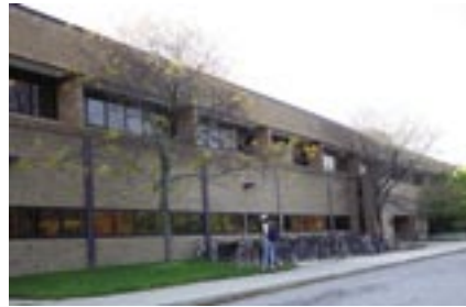
Adding a floor of offices to GG Brown Lab
