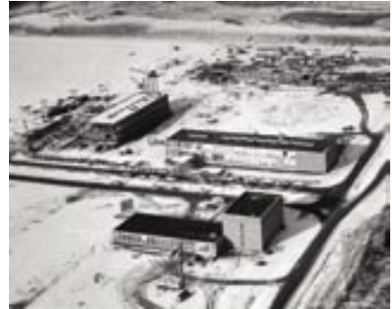
The construction of the Phoenix Laboratory (upper left)
