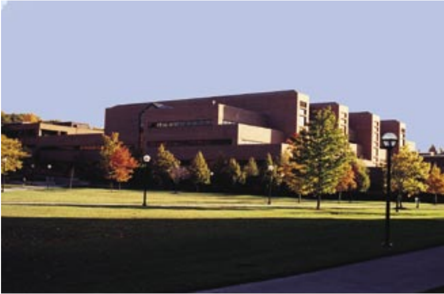
The new EECS building
