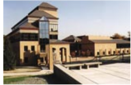
Lurie Engineering Center
