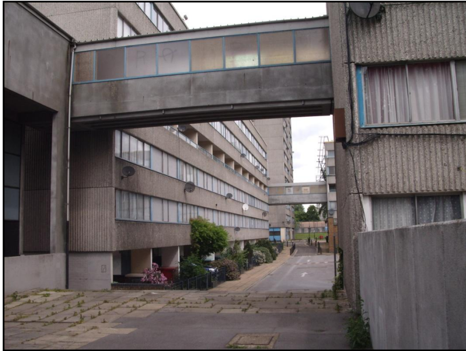
Image 5.1: Block architecture of Ferrier Estate
