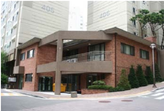
(9) Facility management and community center
