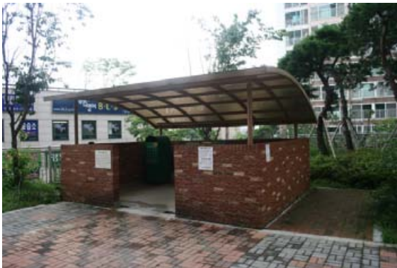
(15) Waste and recycle container
