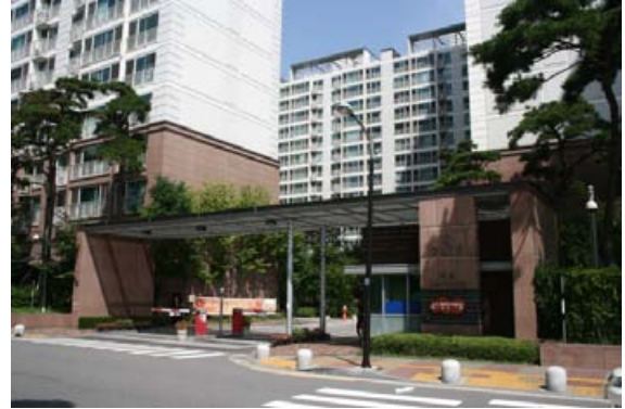
(2) Main gate at the apartment estate
