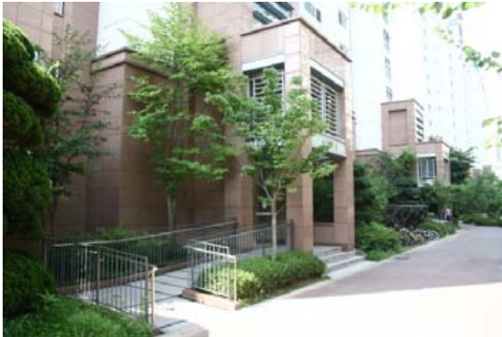
(5) Entrance to an apartment building
