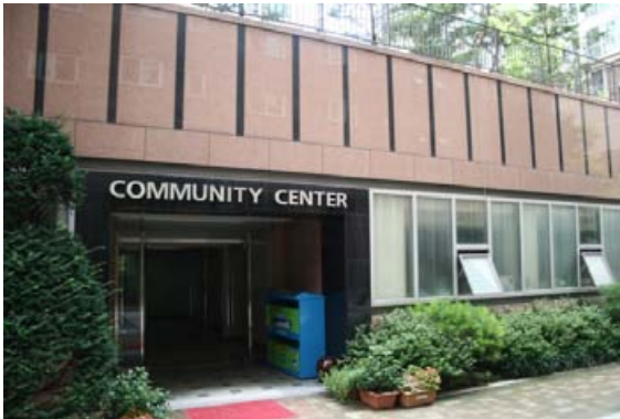
(9) Facility management and community center
