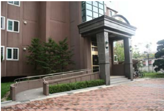
(5) Entrance to an apartment building
