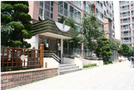
(5) Entrance to an apartment building
