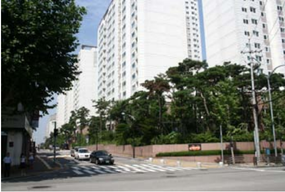
(1) Road approaching the apartment estate
