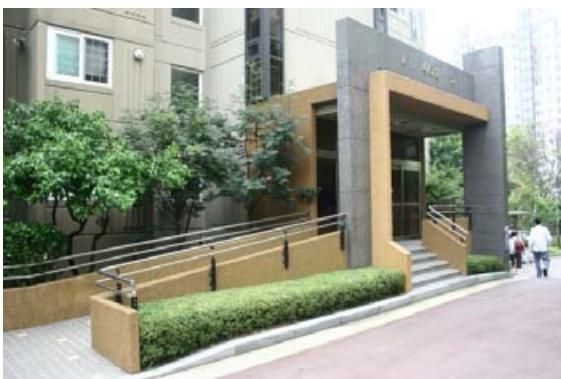
(5) Entrance to an apartment building
