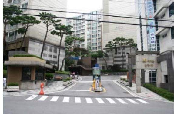
(2) Main gate at the apartment estate
