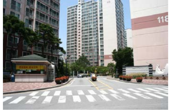
(2) Main gate at the apartment estate
