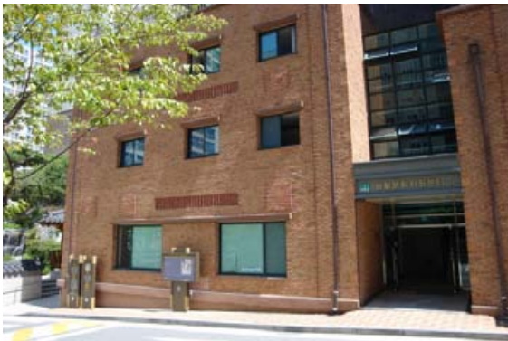
(9) Facility management and community center
