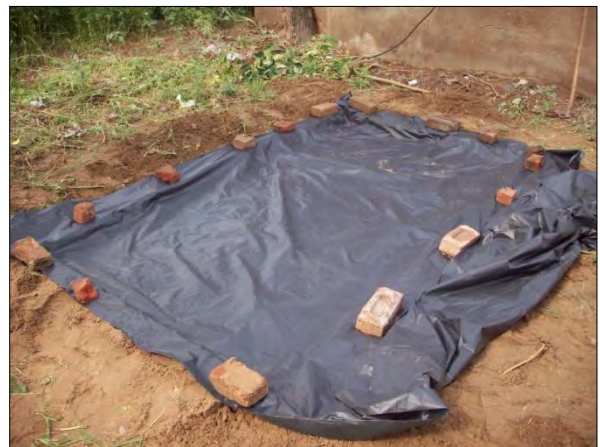
COCO (Bagar): Evaporation pit lined with black plastic (07/17/11)
