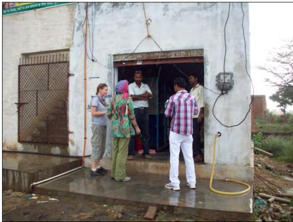
Rajgarh: RO unit and operations building
