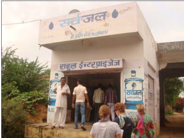
Chirawa: RO unit and operations building
