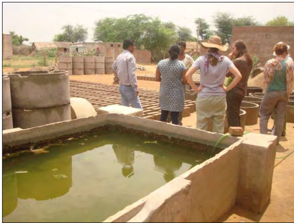
Ramgarh-1: RO brine holding basin
