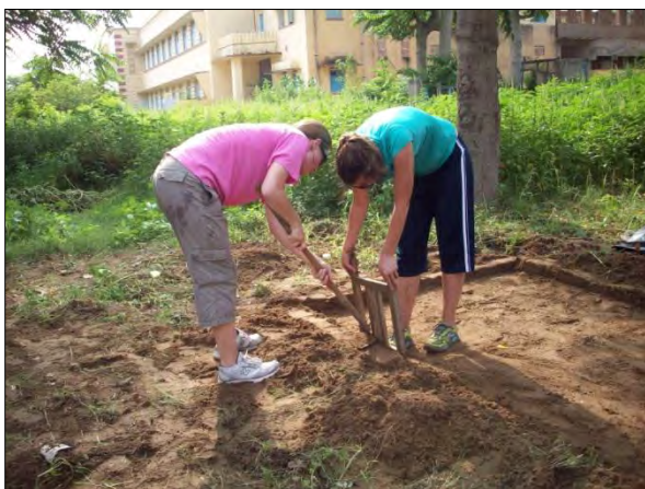
COCO (Bagar): Forming evaporation pit for bench test (07/17/11)
