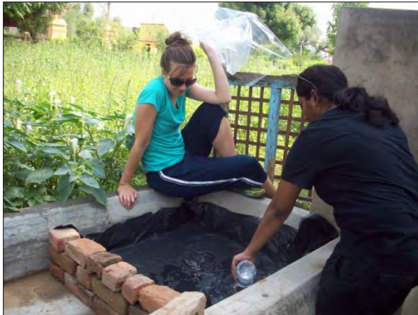
COCO (Bagar): Filling lined evaporation basin in concrete structure (07/19/11)
