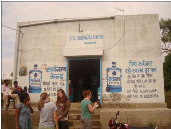
Mandawa-2: RO unit and operations building
