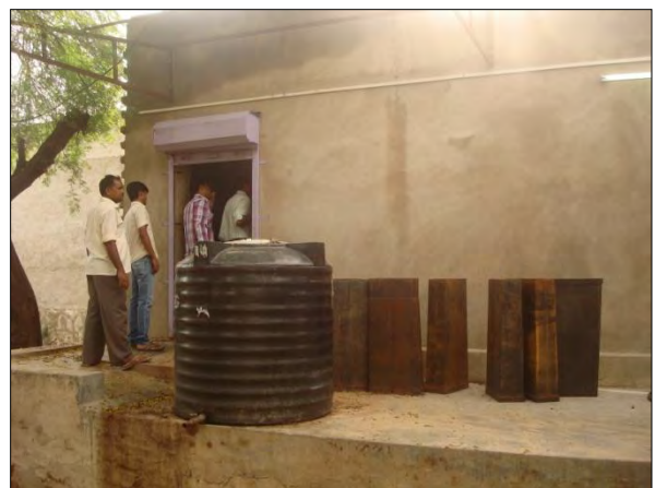
Chirawa: Ice-making operations building and ice bins
