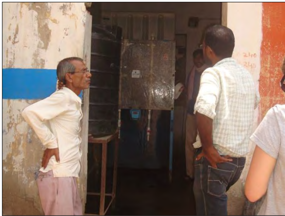
Mandrela: Discussing RO unit operations
