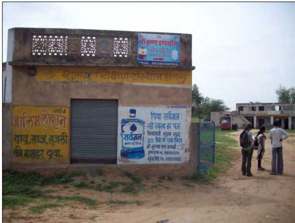
Mukundgarh: RO unit and operations building
