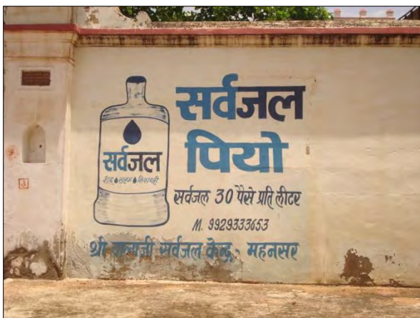
Ramgarh-2: Building front - owner not present
