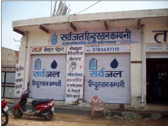
Nawalgarh: RO unit and operations building
