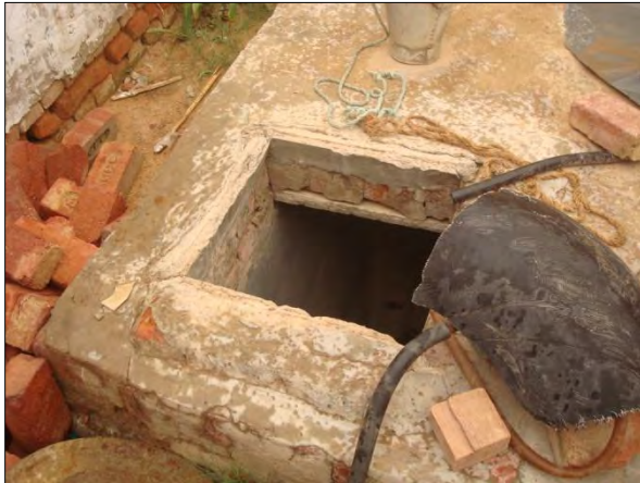
Sadulpur: Groundwater recharge pit
