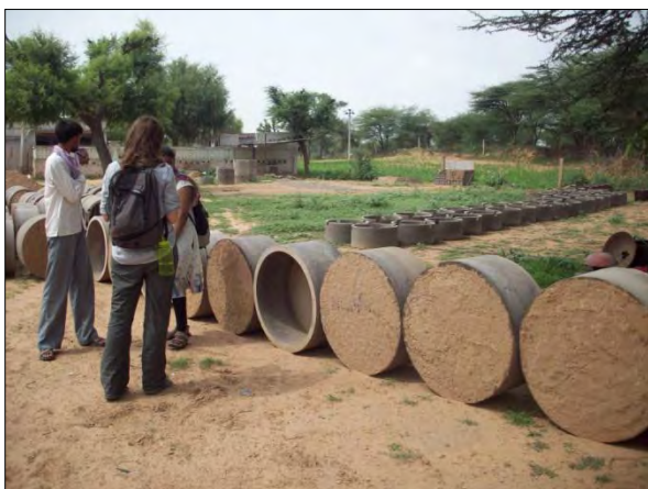
Mukundgarh: Concrete septic tank forms
