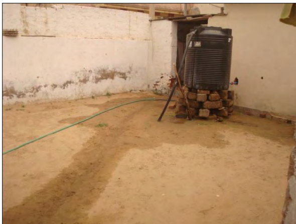
Fatehpur-2: RO brine holding tank area
