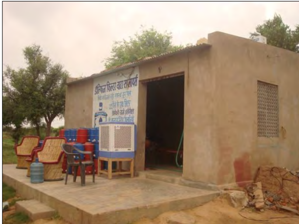
Siriyasar Kalan: RO unit and operations building
