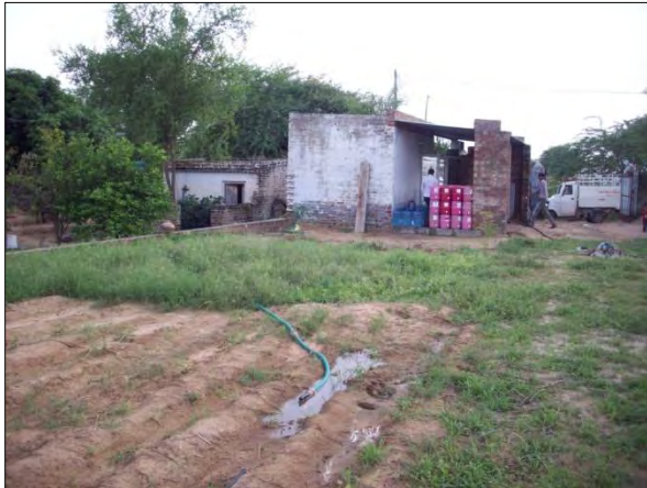
Taranagar: RO unit and operations building
