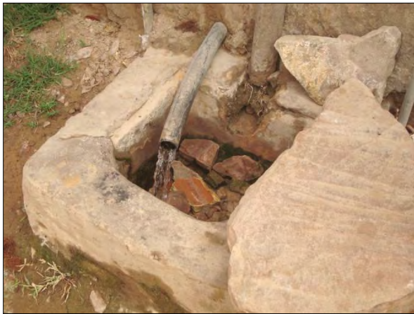
Copper-1: RO brine discharge to sewer
