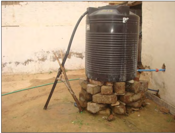
Fatehpur-2: RO brine holding tank
