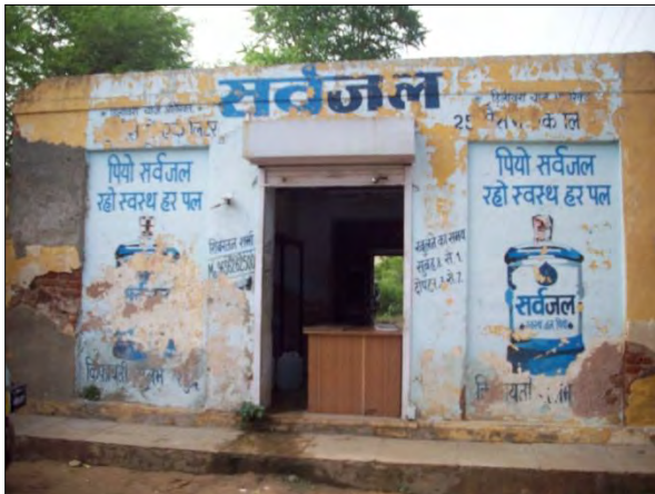
COCO (Bagar): RO unit and operations building
