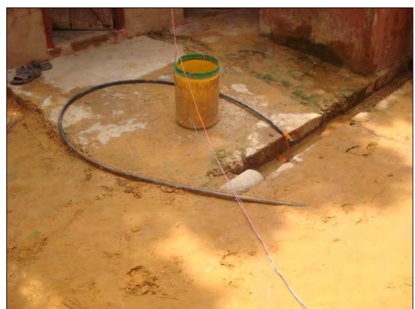
Gothara: RO brine discharge to irrigation ditch
