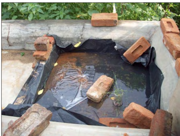
COCO (Bagar): Evaporation basin after vandalism (07/20/11)
