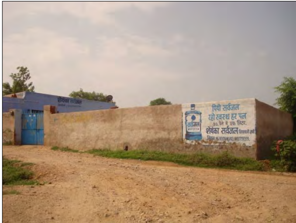
Singhana-2: RO unit and operations building
