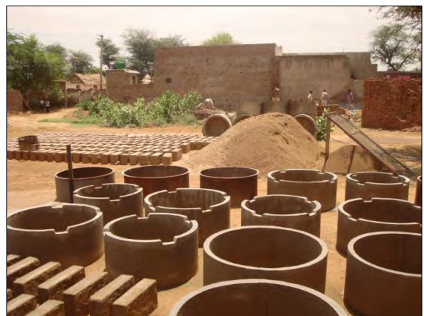
Ramgarh-1: Concrete operations
