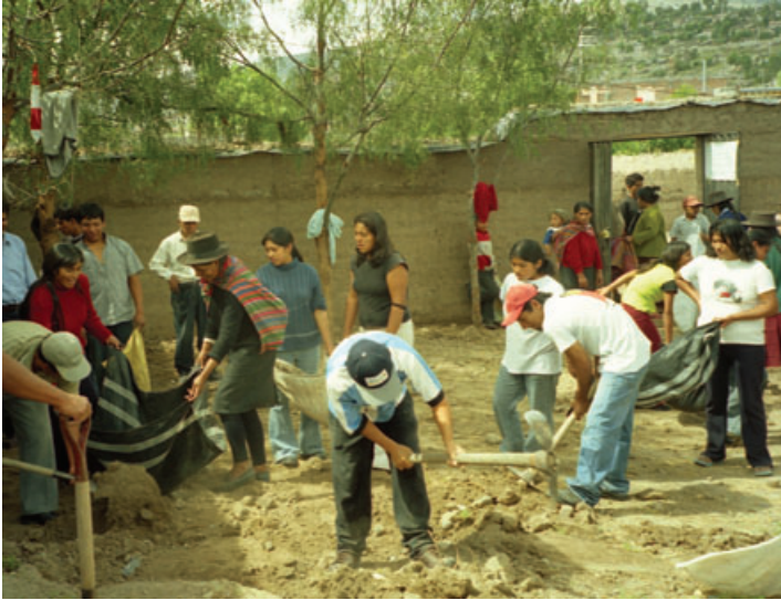
Figure 2. Faena (Work Party) to Construct a Community Centre, Los Olivos
