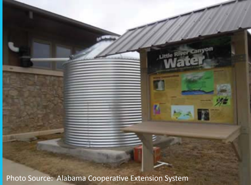
Figure 16: Rain water harvesting system at Little River Canyon Center in Alabama
