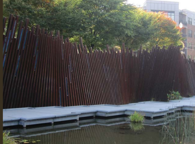
Figure 5: Tanner Springs, a constructed wetland and city park is located in downtown Portland
