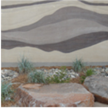
School 1: Natural building techniques demonstrated in clay wall
