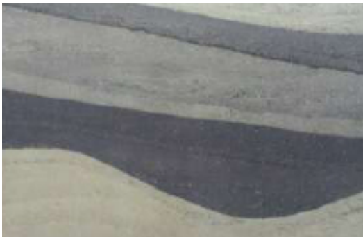
Building Materials: “This picture shows one of the walls in the school that soaks up the heat, so that in the hot summer months, it’s nice and cool inside” (Student 34).
