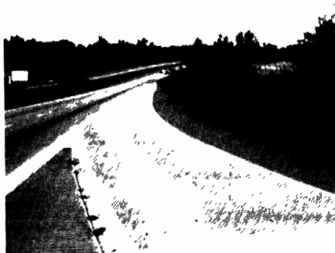
Figure D-22. Three Views of the Entrance Ramp as a Vehicle Proceeds Up the Ramp to the Acceleration Lane.
