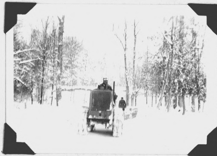
Snowplowing with A.C. Model M and homemade plow.
