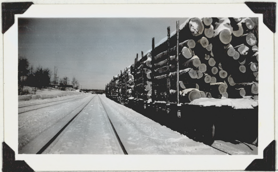
Flat cars loaded with logs on the main line. Car capacity varies from 5M - 8M.
