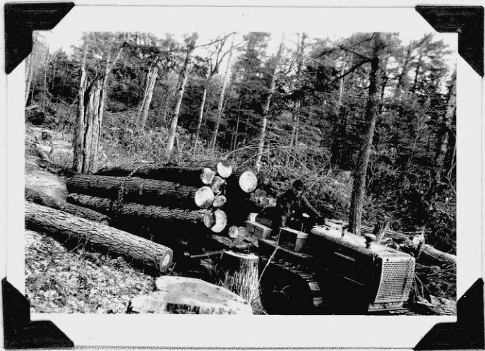
Dray haul using Caterpillar RD4
