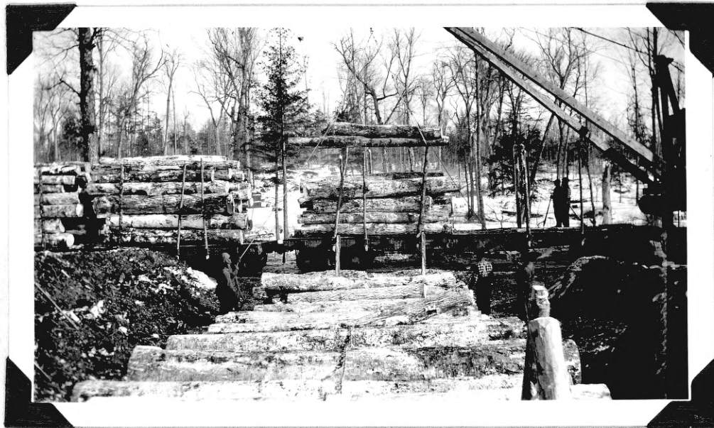
The loading crew, consisting of two hookers, two tailers down, one top loader and one jammer bullcook. The hoist operator cannot be seen. Note the expensive skidway necessary on this operation.
