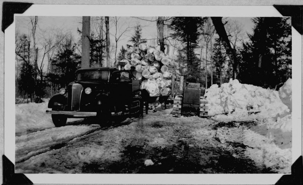
Another View Of Sleigh Haul Unit. Truck is Equipped With Two Speed Rear Axle
