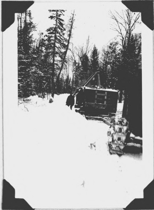
Icing road with sprinkler
