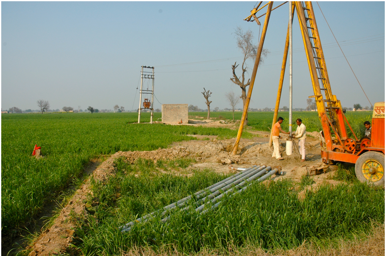
Figure 4-2. Digging a well in a field. Bani, Sirsa District, Haryana.
