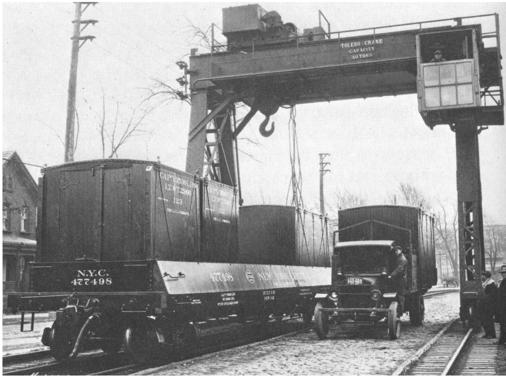
Figure 5.2: Containers being transferred between train and truck in the 1920s
