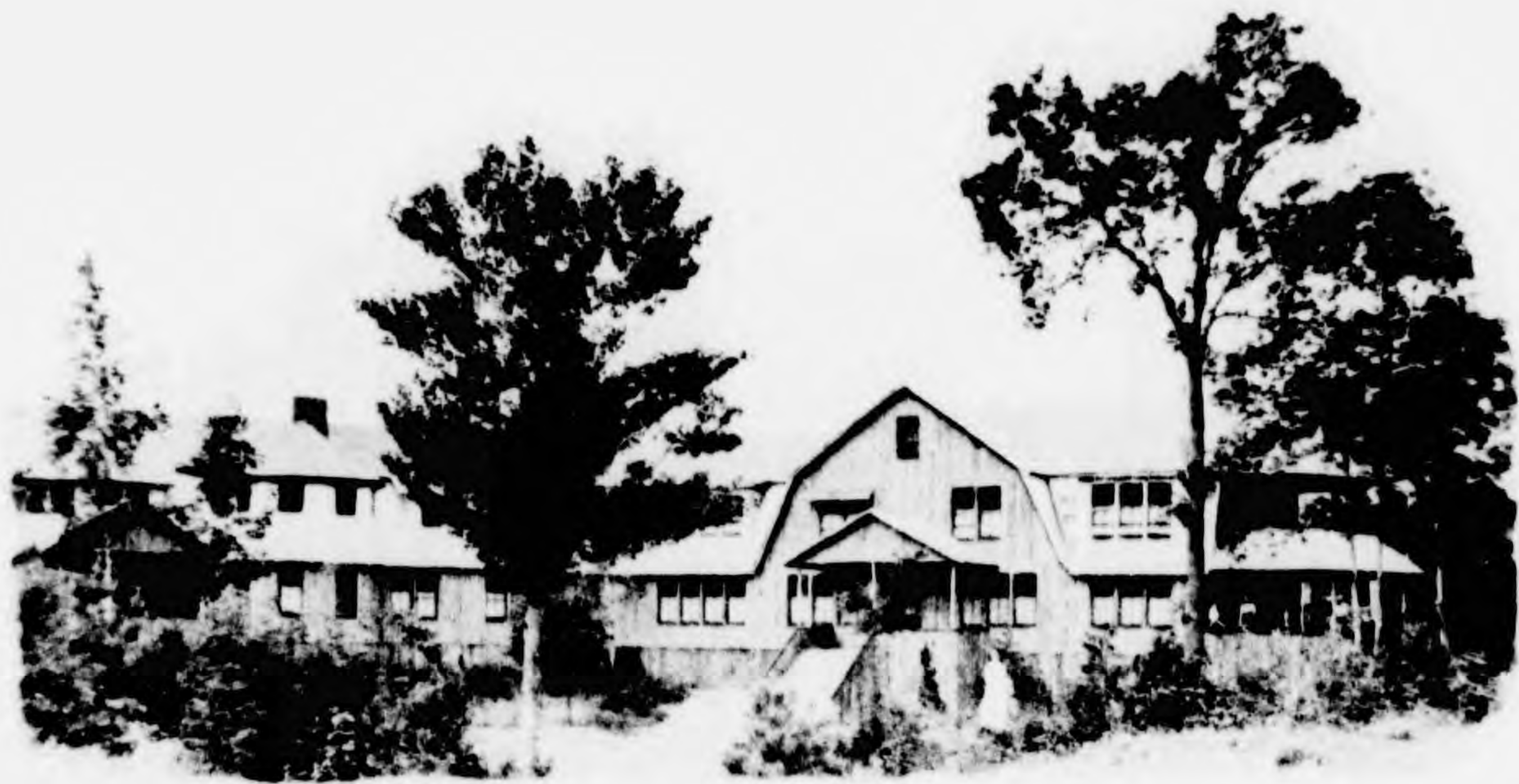
CLUB HOUSE—Harbor Beach Association. Managed on a Co-operative Basis.
