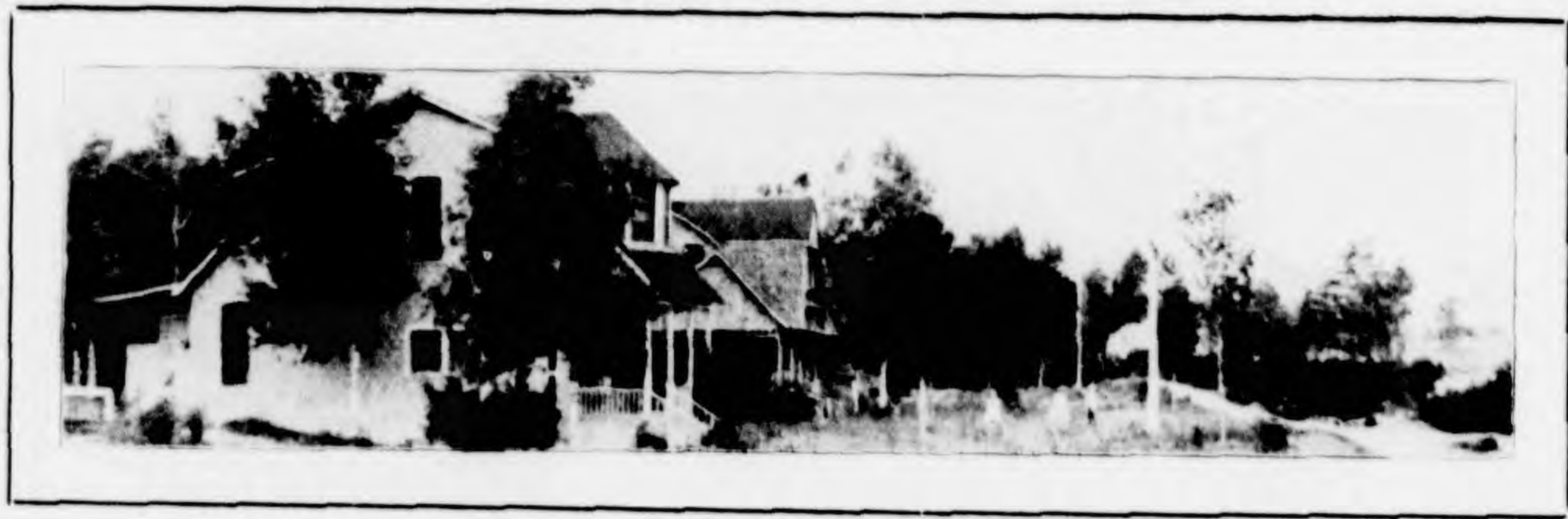
SOUTH OF GROUNDS, LOOKING TOWARD CENTER
