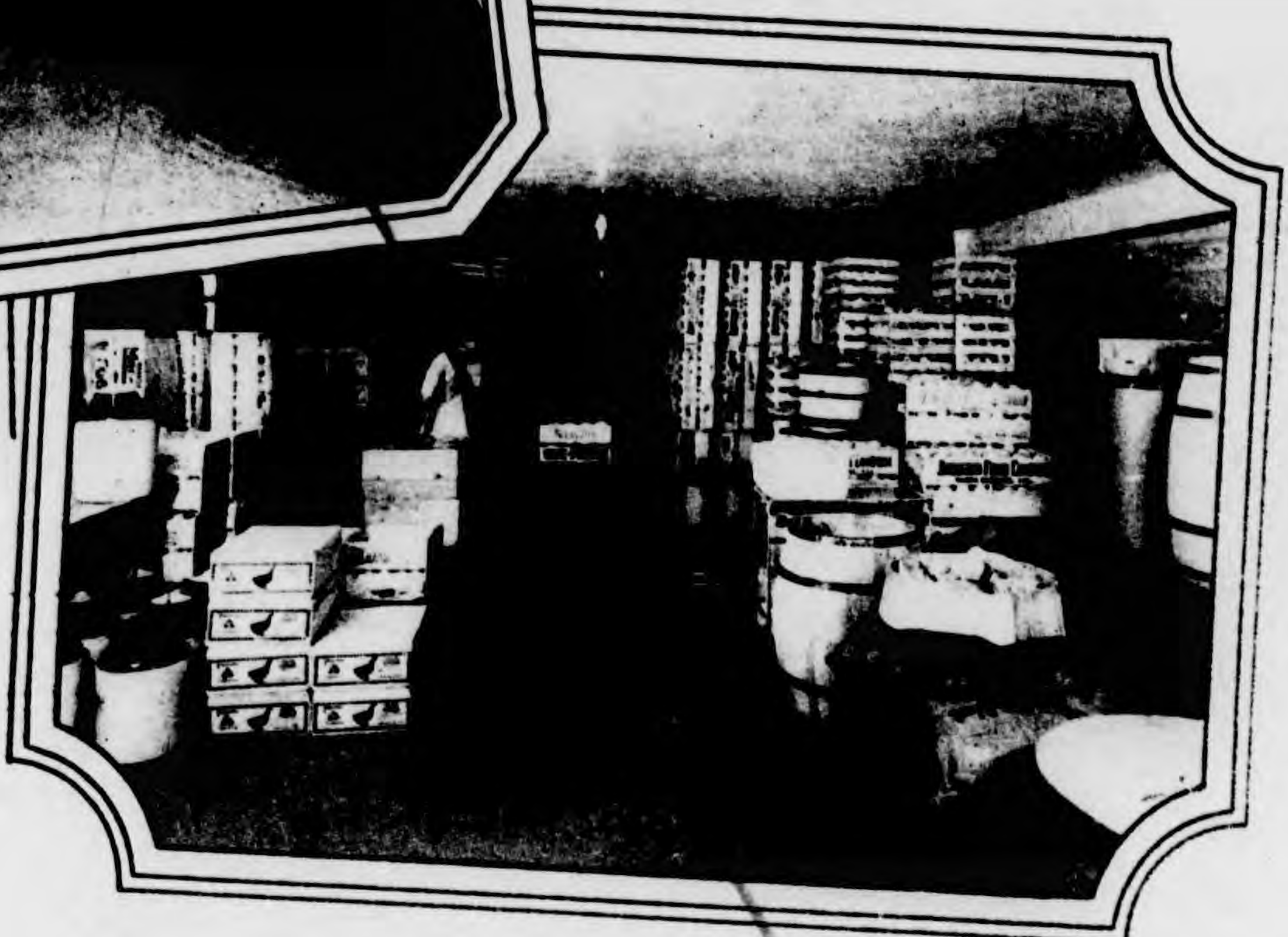
Interior of Refrigerating Room
