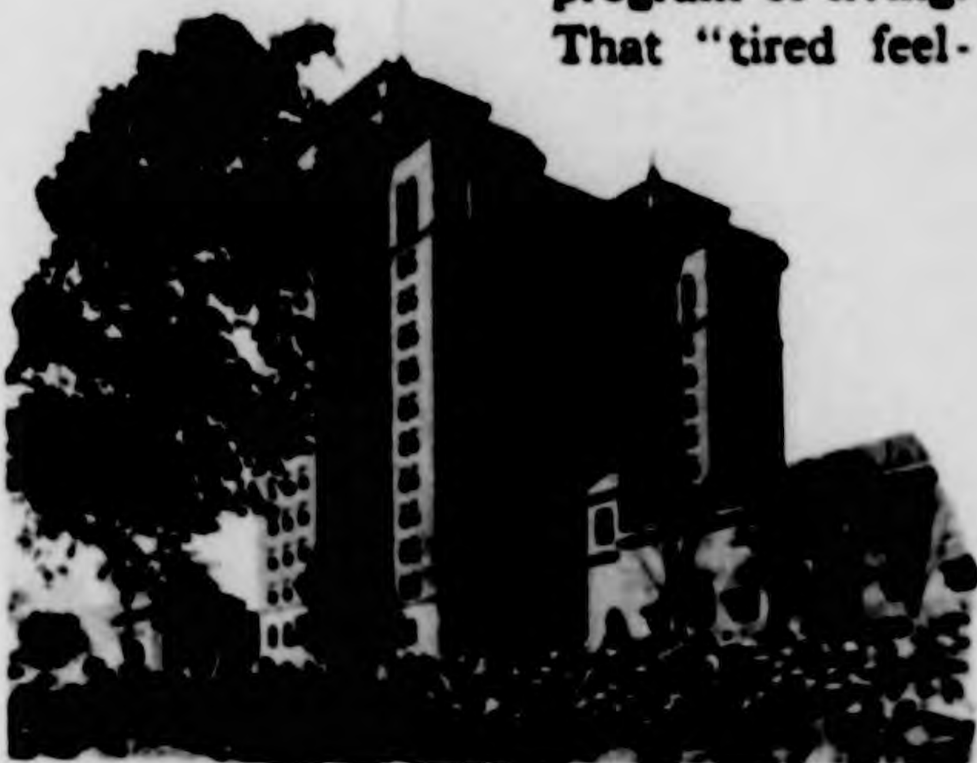
A glimpse of the new Sanitarium Fifteen-Story Addition from the Rock Garden
