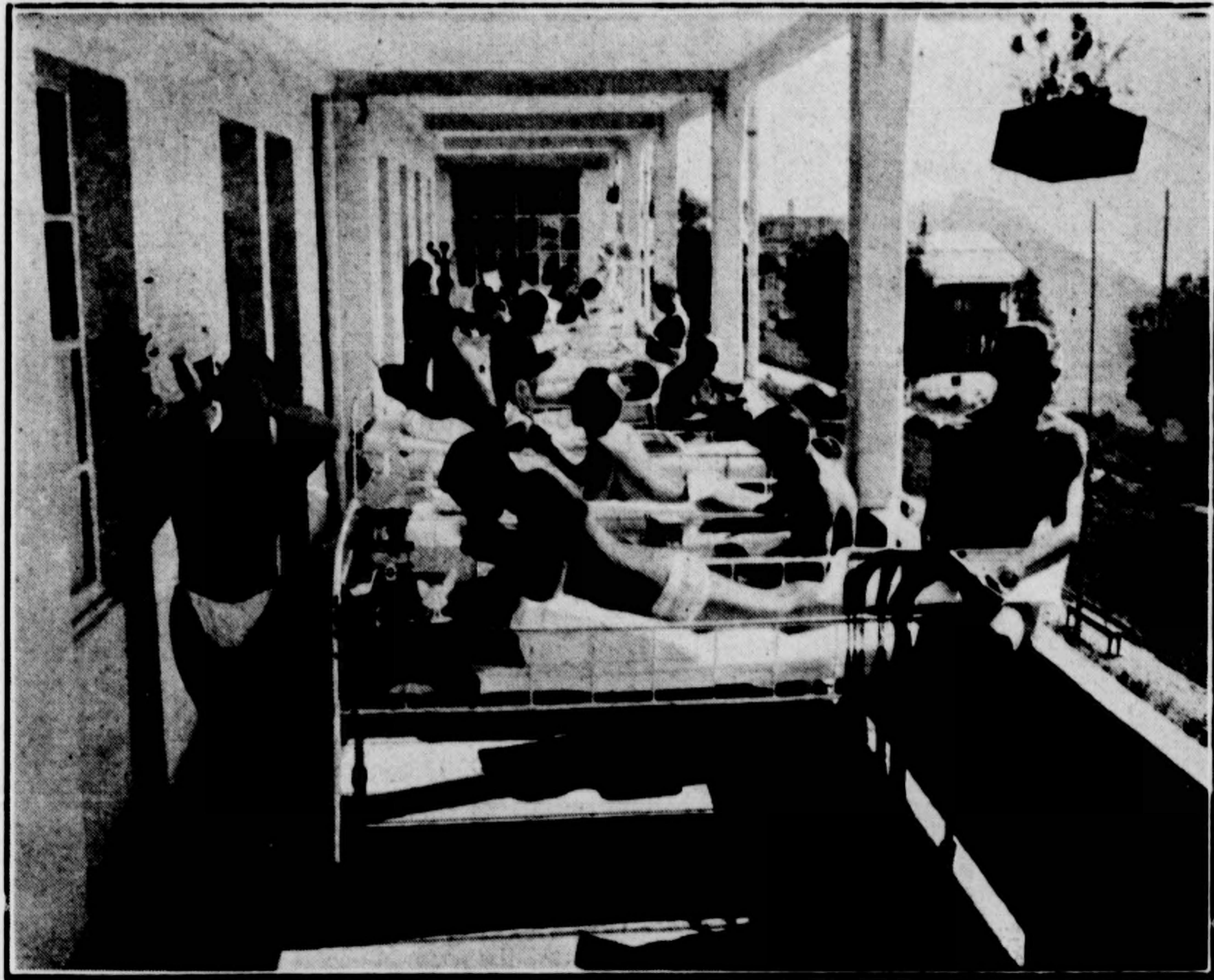
FIG. 73. — A balcony of the military clinic where one sees in natural association heliotherapy and the work cure, under constant medical control.
