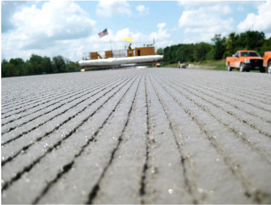
Figure 33. Texturing concrete pavement with longitudinal tining.
