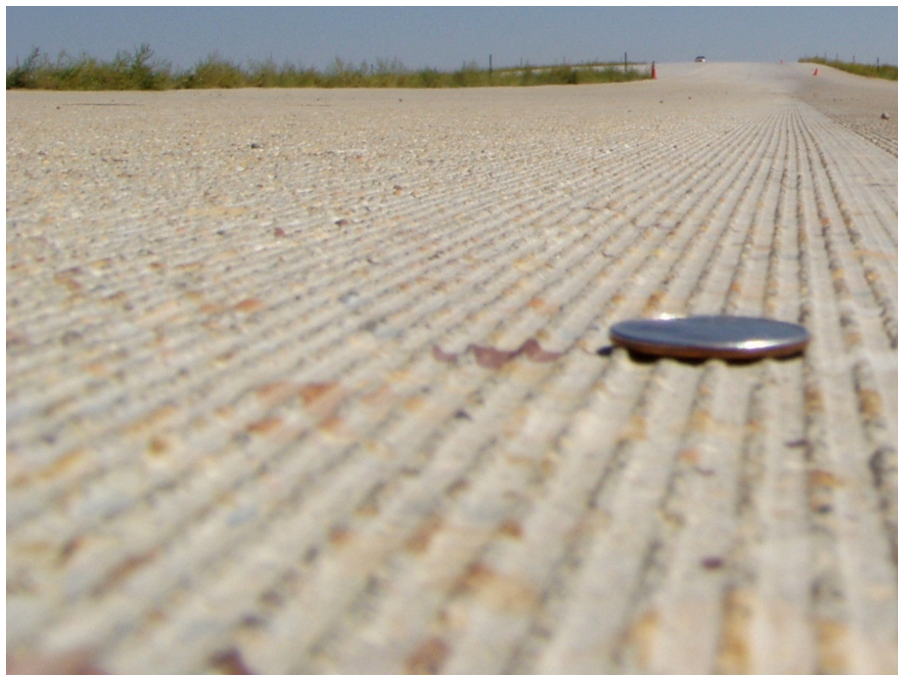
Figure 36. Texturing concrete pavement by diamond grinding.
