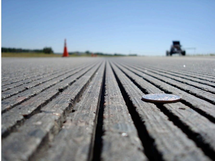
Figure 37. Texturing concrete pavement by grooving.
