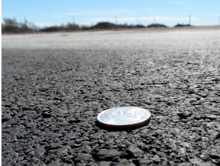
Figure 27. Dense-graded asphalt wearing course.
