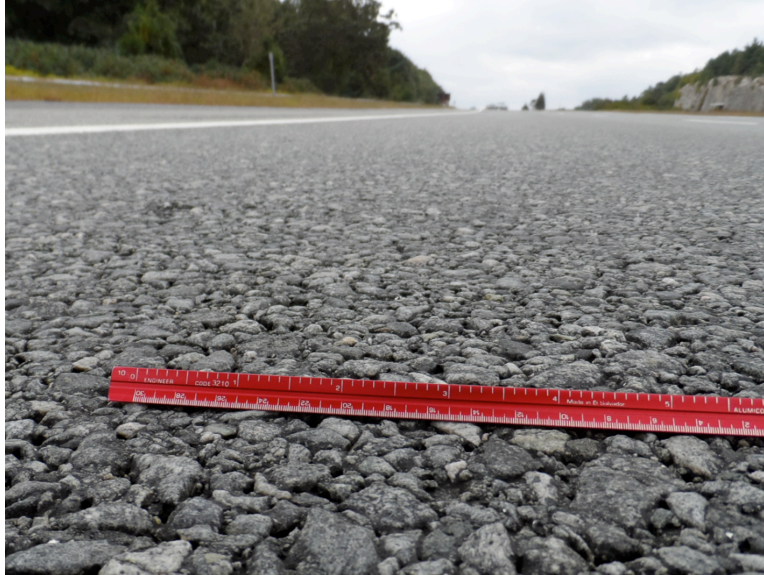
Figure 28. Open-graded asphalt wearing course.
