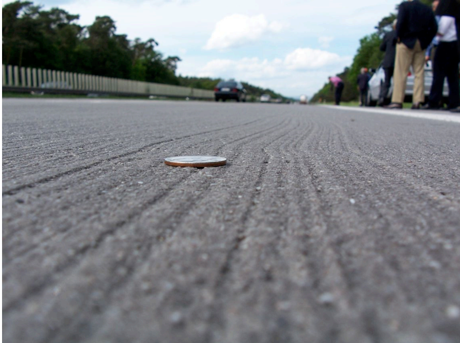
Figure 35. Texturing concrete pavement by artificial turf drag.
